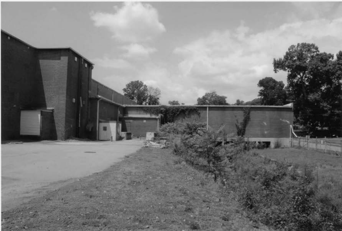
42. Drayton Mill 1802 Drayton Road, Spartanburg vicinity Spartanburg County, South Carolina Weaving building addition (east elevation)
