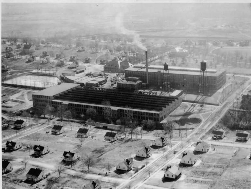
AIRPLANE VIEW SHOWING LARGE WEAVE BUILDING IN FOREGROUND AND SPINNING MILL IN REAR
