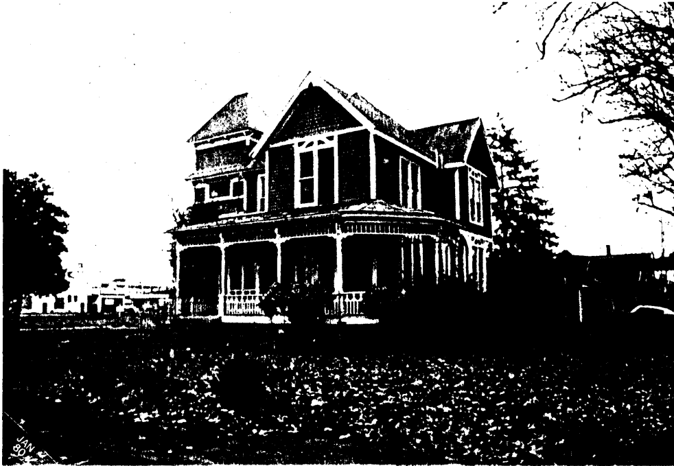
1. View southeast of the Gilbert House prior to restoration.
