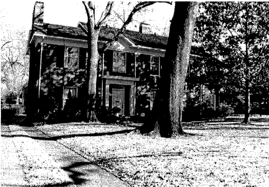
Figure 105: 720 South Broadway, Colonial Revival. Photo by Diane E. Williams
