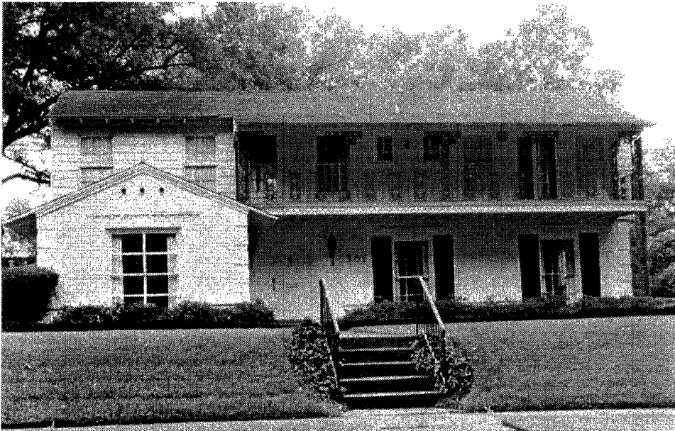
Figure 119: 301 East Third Street, Monterey Revival. Photo by Diane E. Williams
