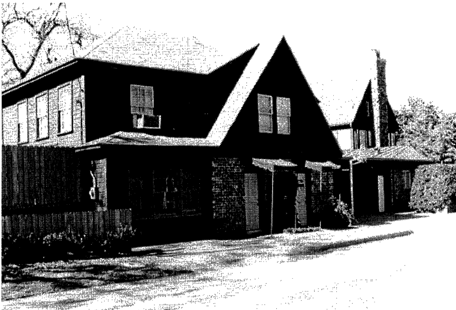
Figure 127: 703 South Fannin Avenue, Gardener's Cottage. Photo by Diane E. Williams
