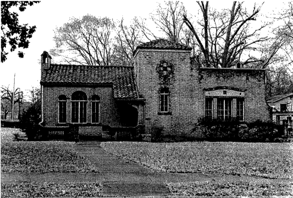
Figure 115: 625 West Dobbs Street, Spanish Colonial Revival. Photo by Diane E. Williams
