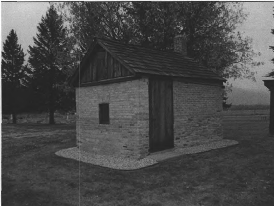
Photograph no. 0020. Smokehouse, south and west elevations.
