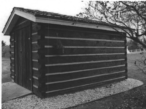
Photograph no. 0032. Pump house, southwest view.
