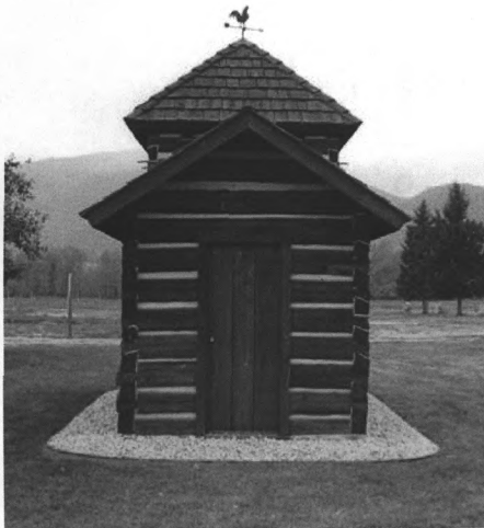
Photograph no. 0031. Dove cote, east elevation.
