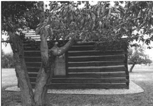
Photograph no. 0018. Victor's house, south elevation.
