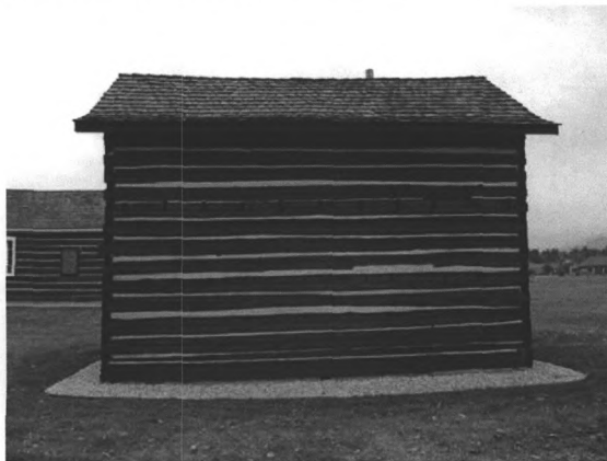
Photograph no. 0008. Father Ravalli's House/Pharmacy, north elevation.
