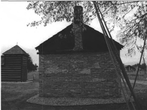
Photograph no. 0021. Smokehouse, north elevation.
