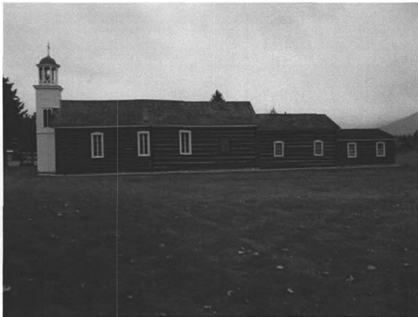
Photograph no. 0004. St. Mary's Mission, north elevation.
