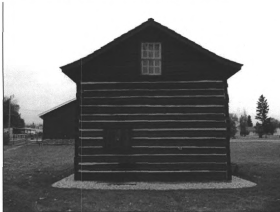
Photograph no. 0009. Father Ravalli's House/Pharmacy, west elevation.
