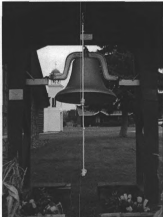
Photograph no. 0016. St. Mary's bell and bell tower, south elevation.
