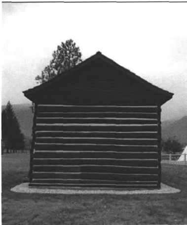
Photograph no. 0007. Father Ravalli's House/Pharmacy, east elevation.
