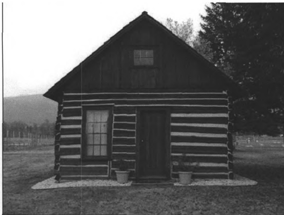
Photograph no. 0017. Victor's House, east elevation.
