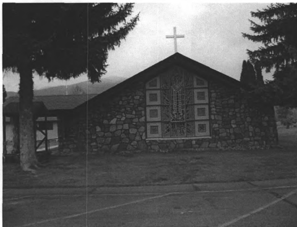
Photograph no. 0012. St. Mary's Church and Rectory, church, east elevation.
