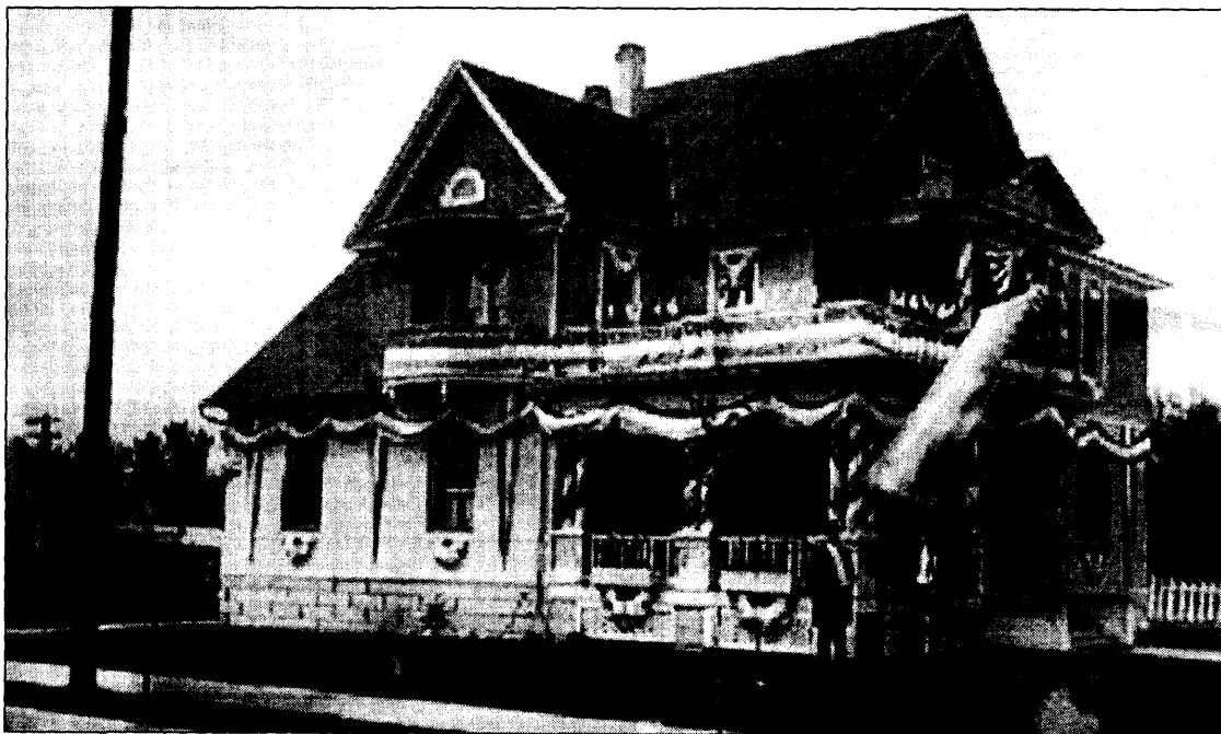
Figure 2. Undated early view of the Bode House decorated in bunting for a Colorado-Wyoming Encampment of the Grand Army of the Republic. SOURCE: www.rootsweb.com , Chaffee County, Colorado, website, accessed 10 October 2007.
