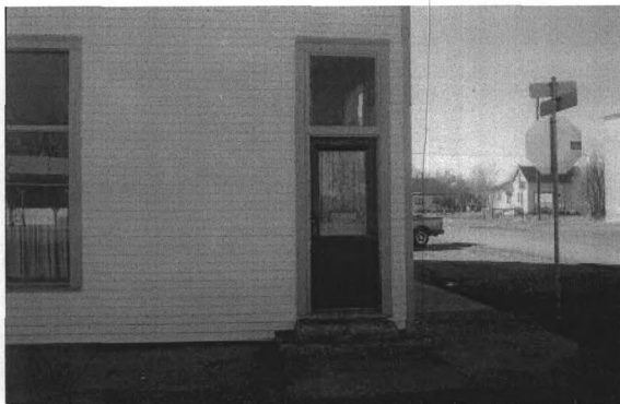
Detail of east elevation entry.
