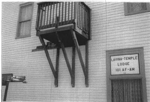
Detail of north elevation.
