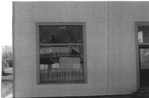
Detail of east elevation first story window.
