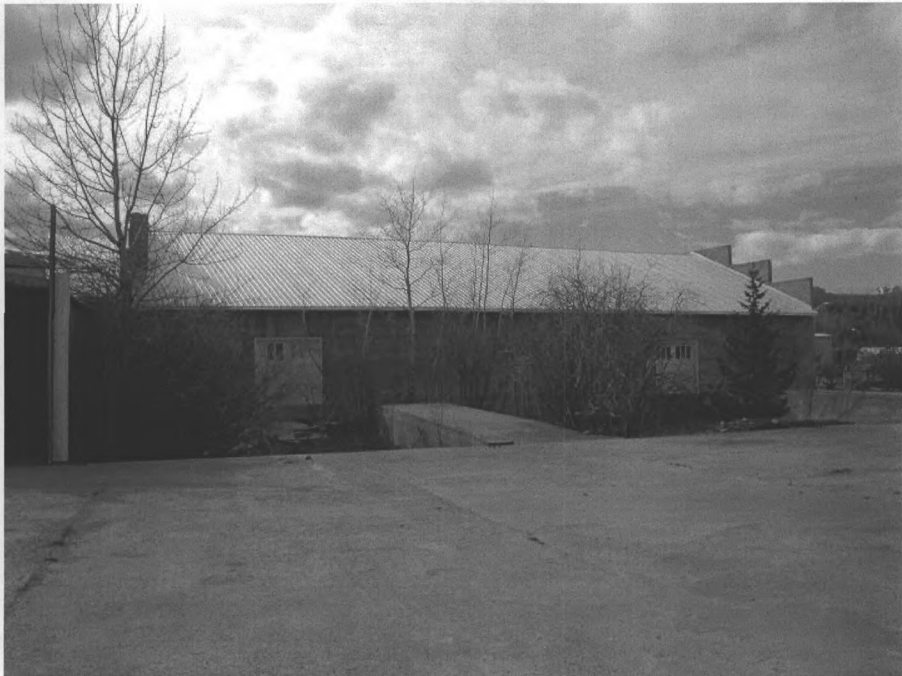
Red Lodge Cannery warehouse foundation, view to west.
