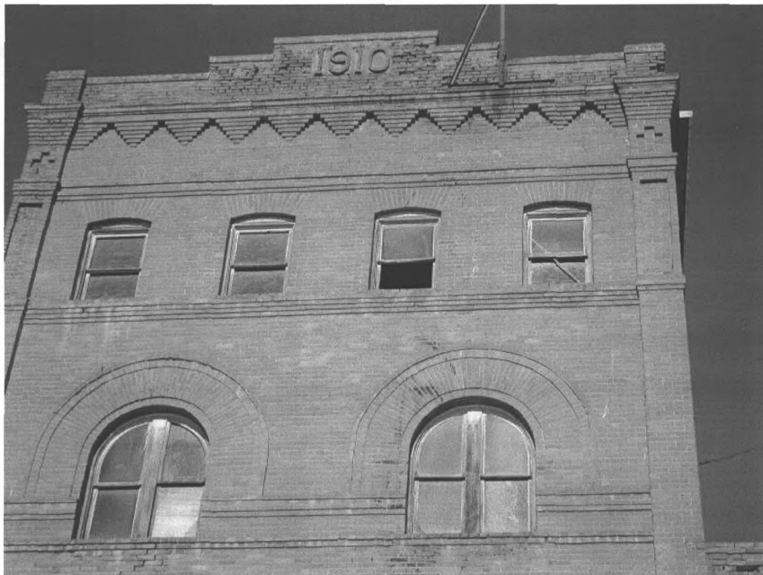
Brewery façade, detail. View to north.
