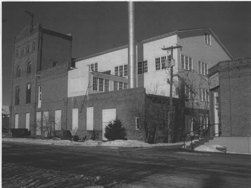
Red Lodge Brewery/Red Lodge Cannery, view to northwest.
