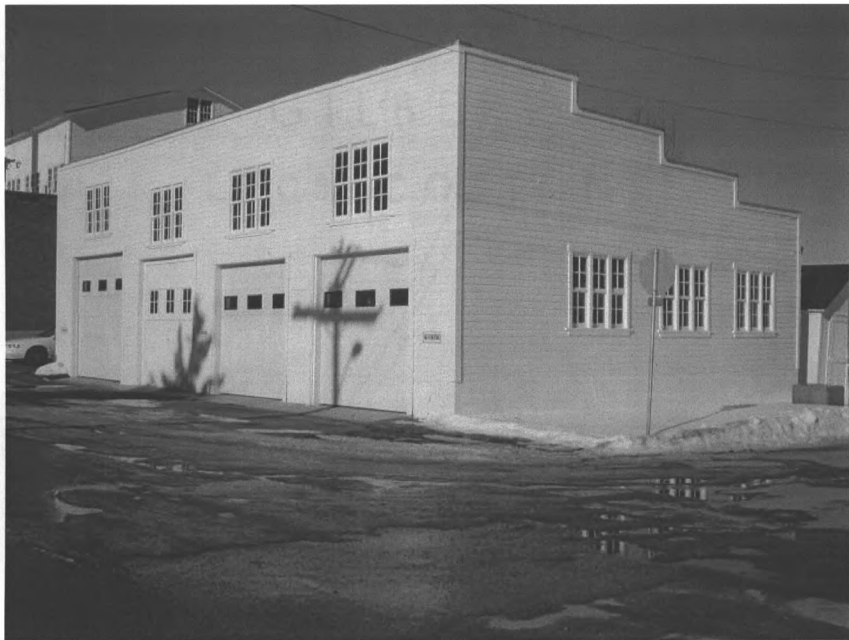
Red Lodge Cannery truck garage, view to west.
