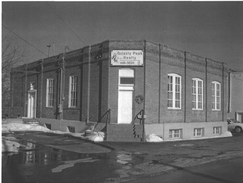
Red Lodge Brewery/Red Lodge Cannery office, view to northeast.
