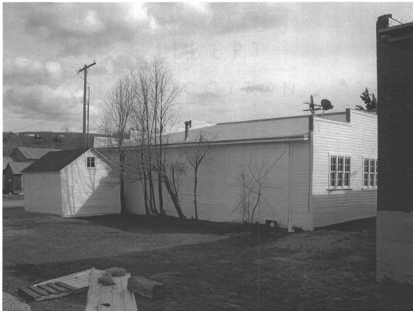
Red Lodge Cannery garages, view to southeast.
