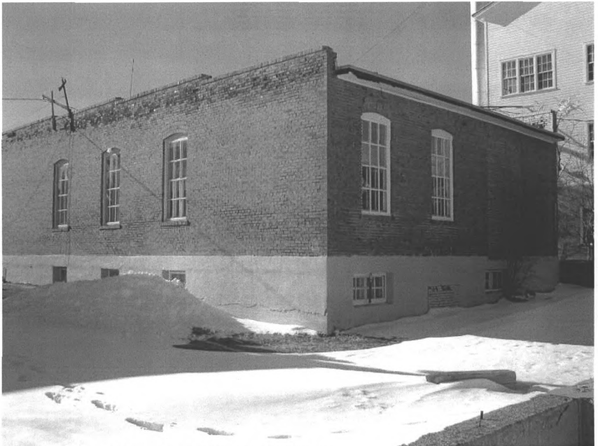
Red Lodge Brewery/Red Lodge Cannery office, view to southwest.
