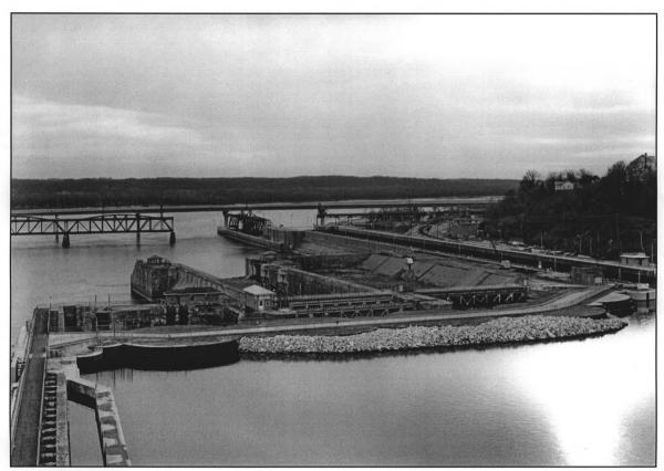
PHOTO 8. General View of Old Lock, Dry Dock, and Sheet Pile Cell Closure Wall. New lock and Keokuk Municipal Bridge in background. Taken before construction of new bridge.
