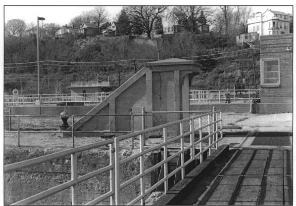
Land Wall Stairway Building. The river wall stairway building is identical PHOTO 7. to this one and mirrors its placement. New lock river wall control station at right side of photo. Visitor's center in background, to the left of the stairway building. Houses in background atop the bluff along the Iowa shore.
