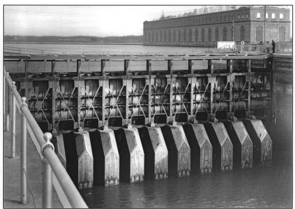
PHOTO 21. Upstream Vertical-lift Service Gate of New Lock, Downstream Side. Photographer: Date of Photograph: Location of Original Negative:
