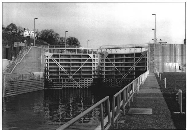
PHOTO 20. Downstream Miter Gates of New Lock, Downstream Side.
