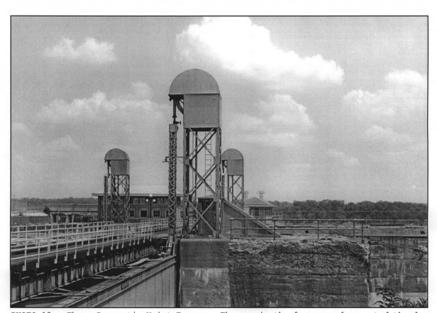
РНОТО 13. Three Pneumatic Hoist Towers. The one in the foreground operated the dry dock gate. The one in the left rear operated the emergency lock gate. The one in the right rear, the main upstream lock gate. Photographer: Peter A. Rathbun
