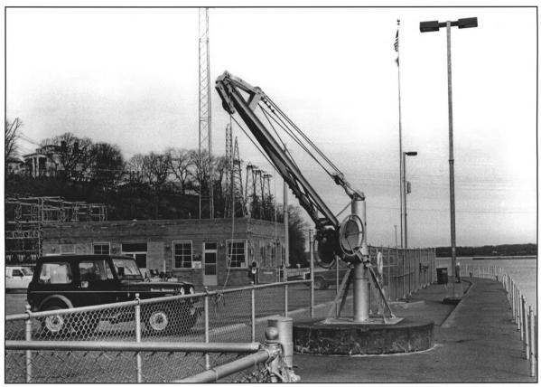
Upstream Land Wall Boat Davet on New Lock. Office and shop in the PHOTO 22. background. Incoming power transformer immediately to left of office and shop building. The other three boat davets on the new lock are identical to the one pictured here.
