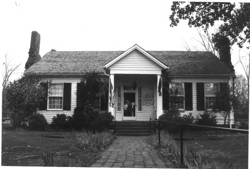
Ivy Green Tuscumbia, AL Main House, Front view Photo by: Doug Letson, 2/90
