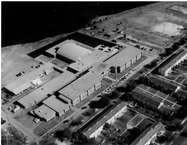
Howard W. Blake High School, Tampa, 1957. Built in 1956, this school was a classic Equalization era school that suffered a fate similar to other black high schools across the state when it was demoted to a junior high school in the early 1970s (source: Hillsborough County Public Library)
