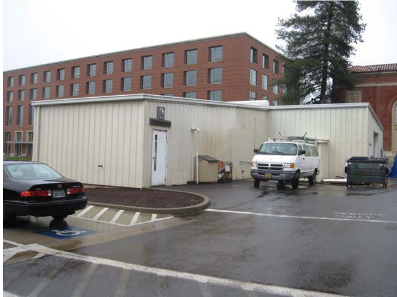
The southeast elevation of the remaining portion of Fairbanks Annex. The brick building stood in the area where the white van is parked in this photo.
