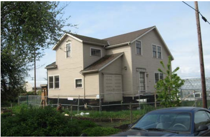
The northeast elevation of the former Black Cultural Center, currently located at 3036 Orchard Avenue.
