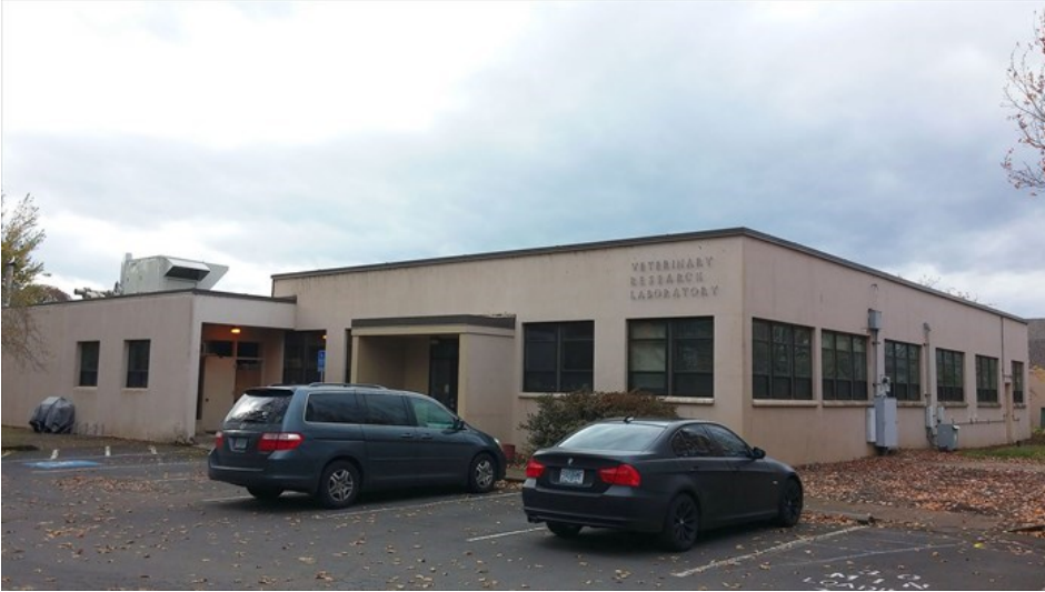
The northeast corner of the building and the primary entrance. This elevation of the building was modified in 1959 and 1972 and is visible from 30th street.
