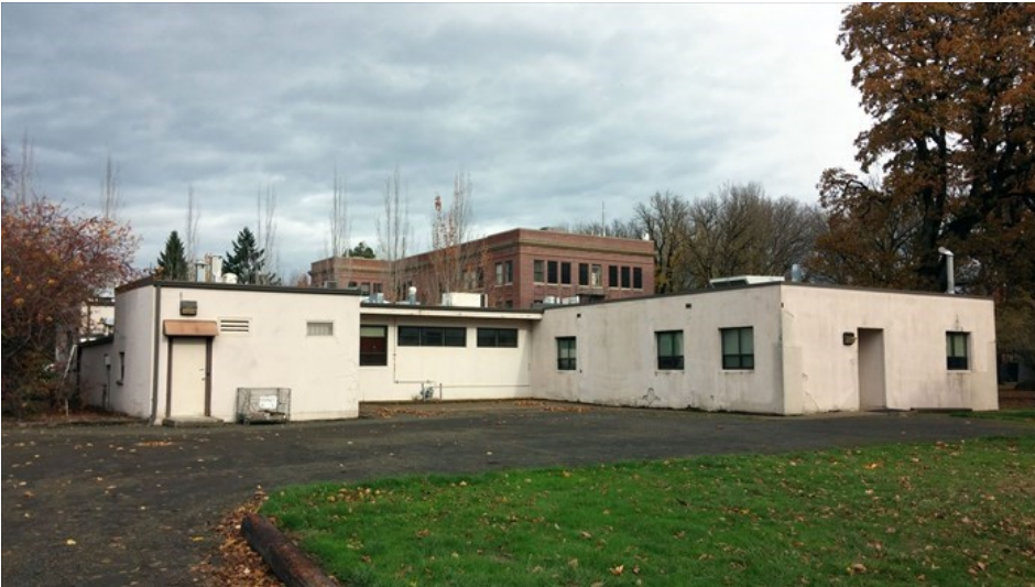
The south end of the building and the two additions added in 1965 and 1972. This is the elevation visible from Washington Way.
