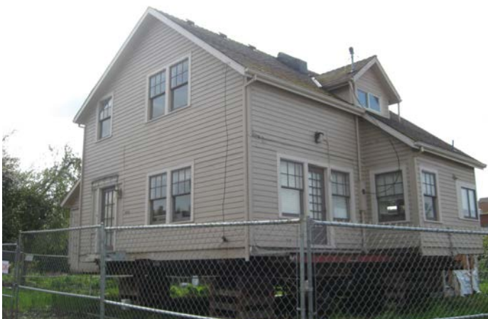
The northwest elevation of the building, viewed from the adjacent alley.
