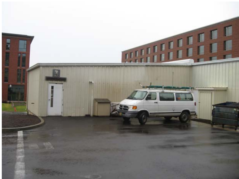
The east elevation of the remaining portion of Fairbanks Annex. The brick building stood in the area where the white van is parked in this photo.
