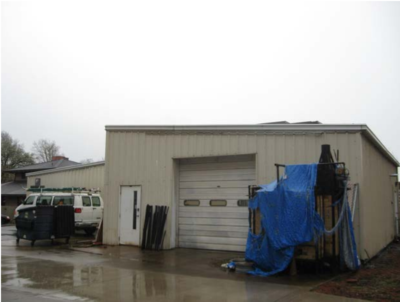
The northeast corner of the remaining portion of the Fairbanks Annex building. The original demolished brick building stood in the area where the white van is parked in this photo.
