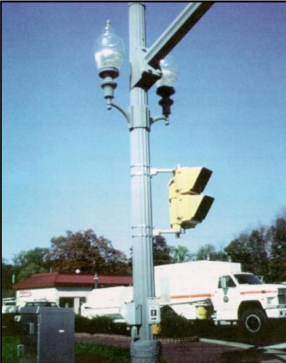
*Pedestrian signals integrated with a combination traffic signal support and street light pole.*
