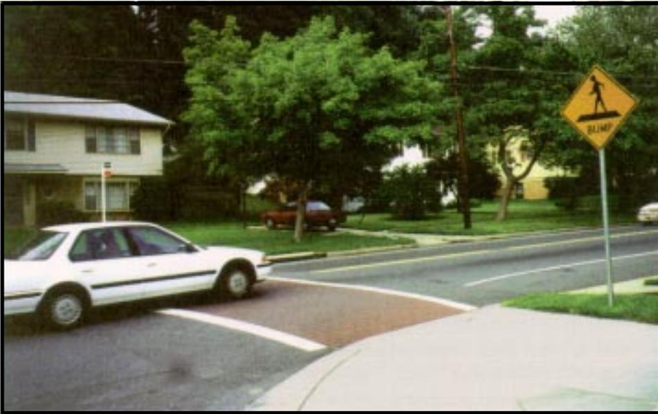
*A clearly delineated and elevated crosswalk, signage, and appropriate turning radius design contribute to this pedestrian-friendly intersection.*
