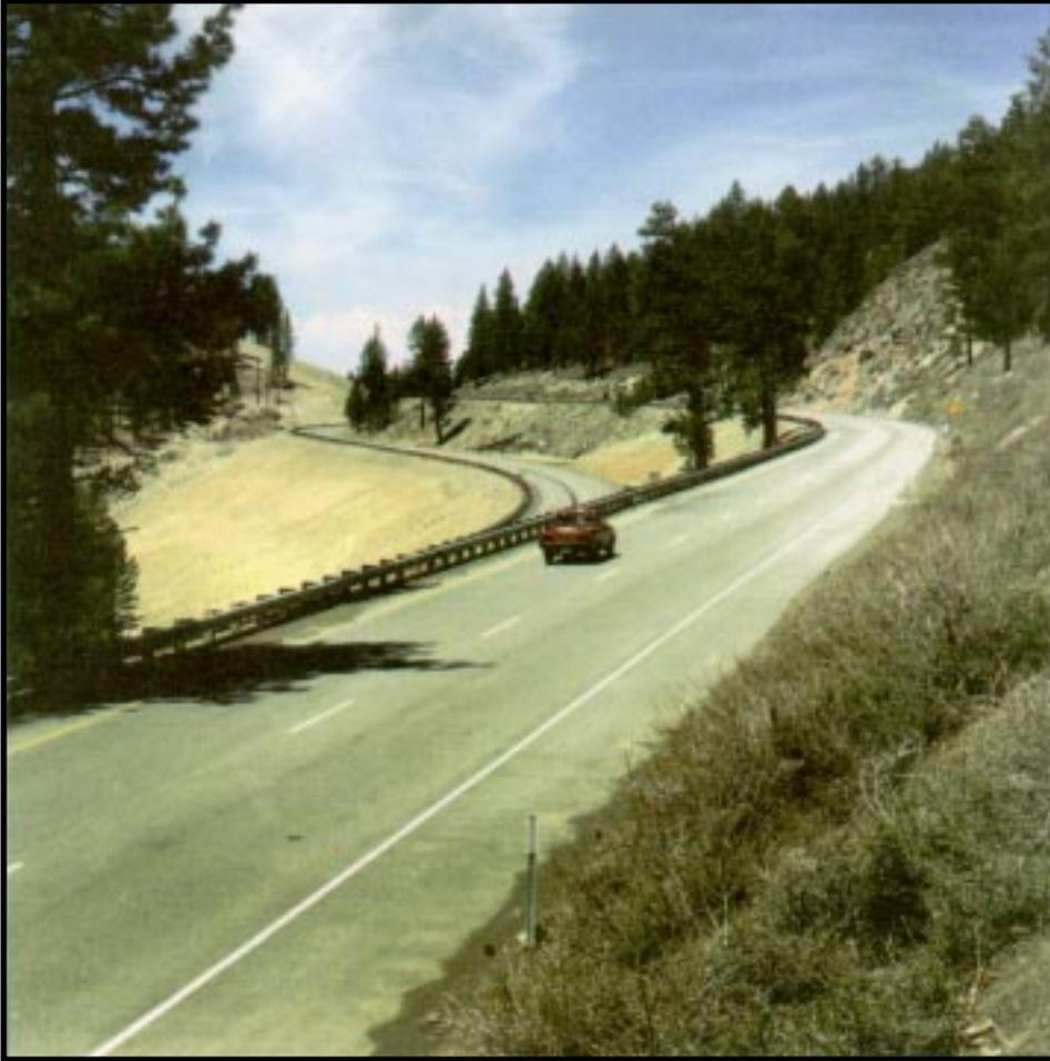
*Separate profiles and varied median widths on divided roadways are options for designers to minimize impact on the environment.
