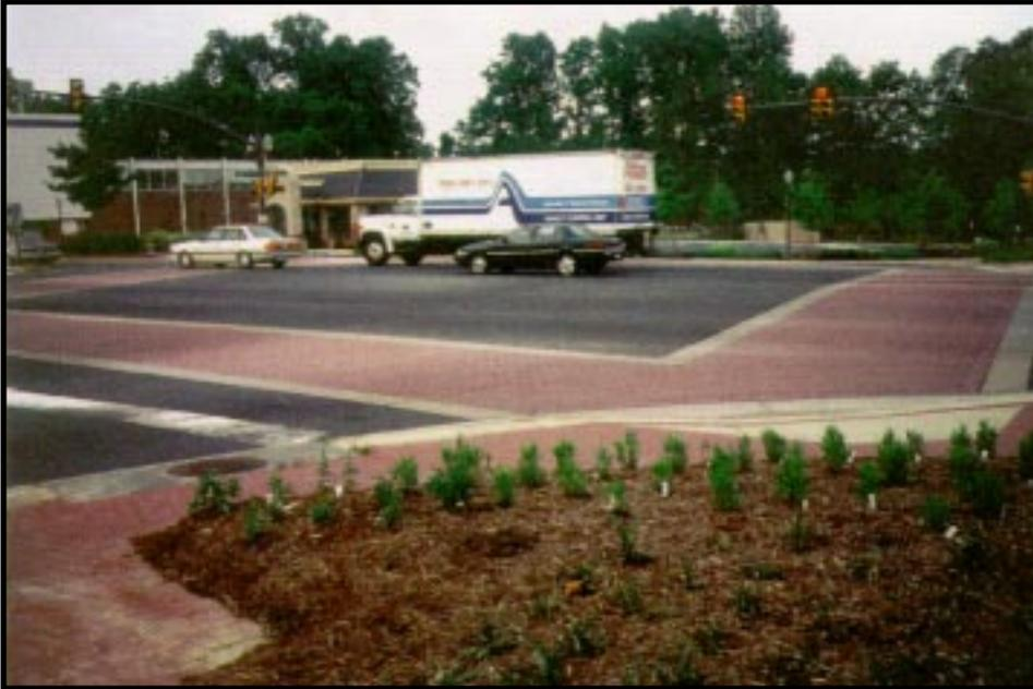
*Pedestrians rely on intersection locations to cross roadways. At the same time, by adding left- and right-turn lanes and large turning radii, intersections can be and often are the widest parts of roadways. The distance pedestrians must cross is an important consideration in design.*
