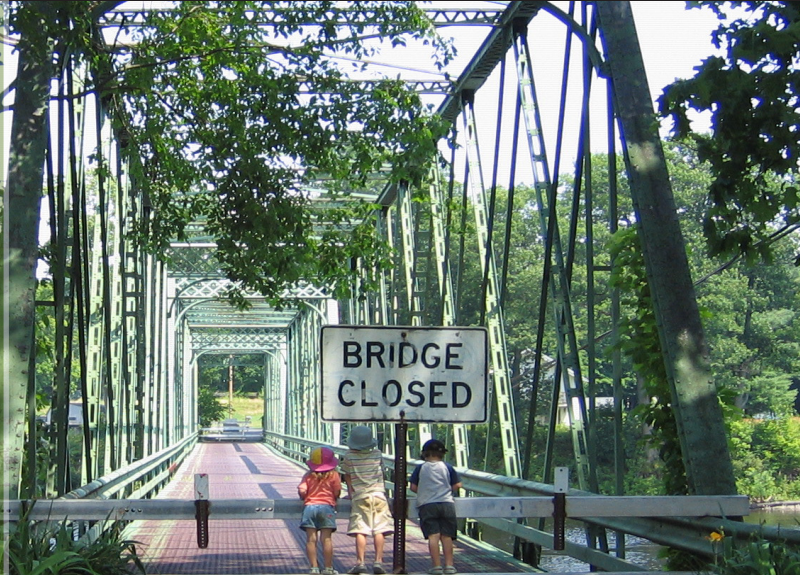
After years of disuse, Dix Bridge in Schuylerville will be restored
