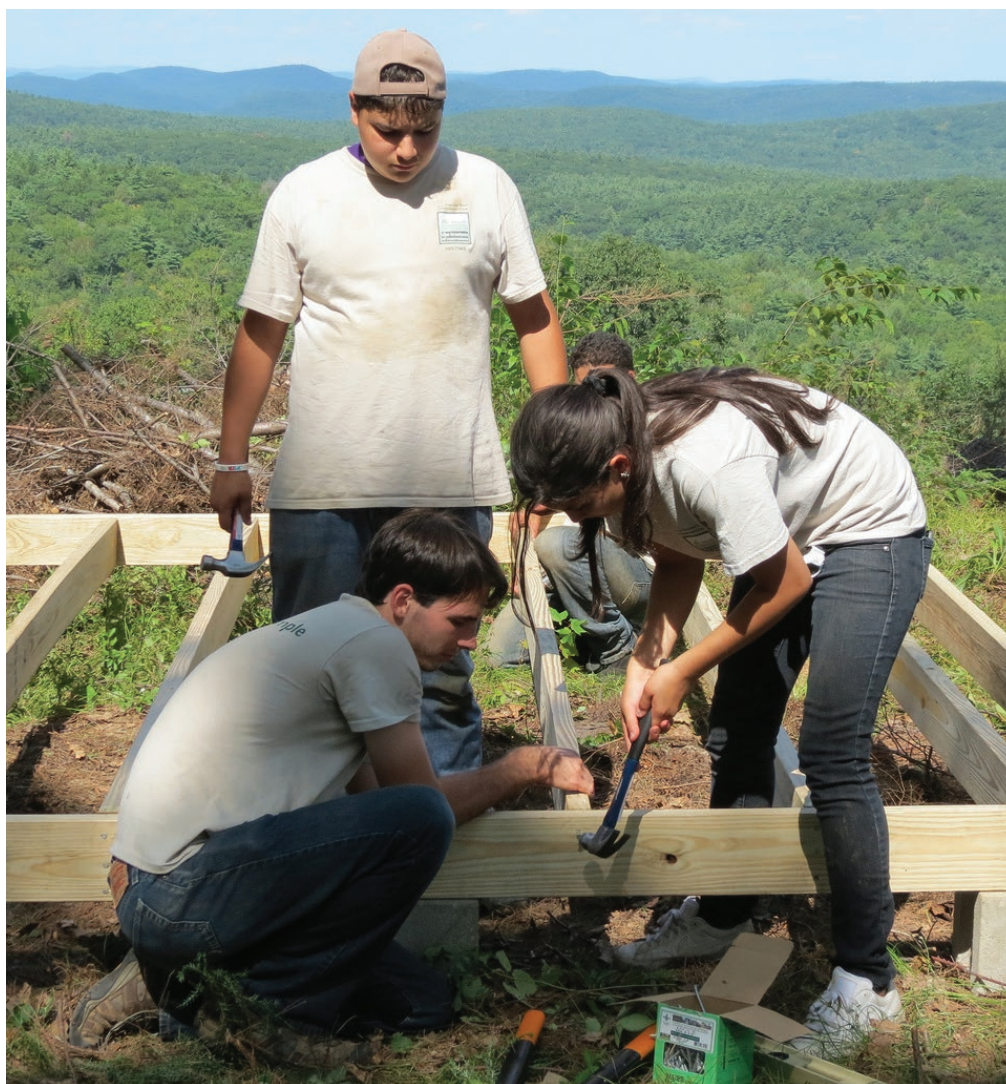
Youth Conservation Corps team building tent platforms on the New England Trail. Photo: Appalachian Mountain Club
