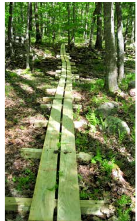
A bog bridge constructed by volunteers in Tillinghast Pond Preserve. Photo: Tim Mooney
