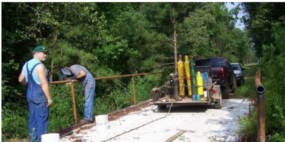
Volunteers deck and rail a bridge. Photo: Friends of DeKalb Trace
