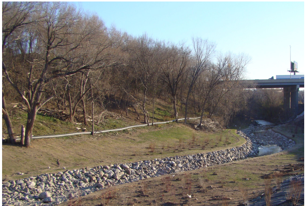
Kinnickinnic River Trail major restoration completion is a great project success.
