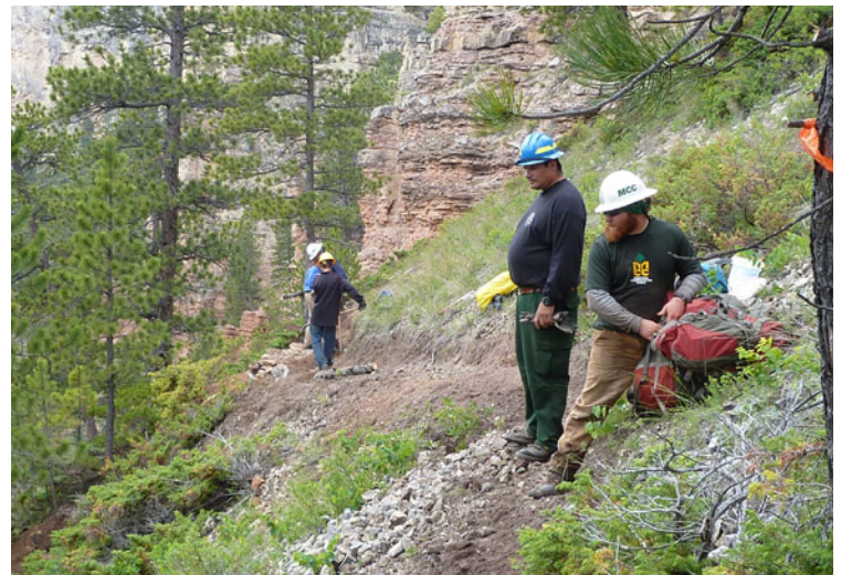
Construction of Hole-in-the-Wall trail, Fort Belknap Indian Reservation
