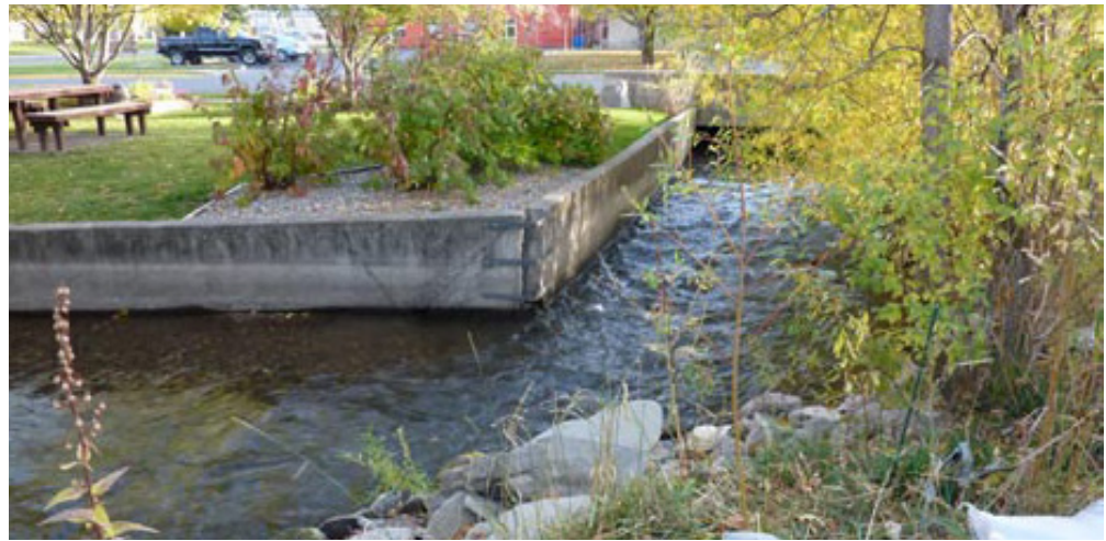
Frequently flooded area along Bozeman Creek
