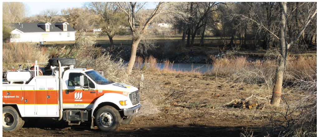
Clearing the corridor for the Aztec Ruins Trail.
