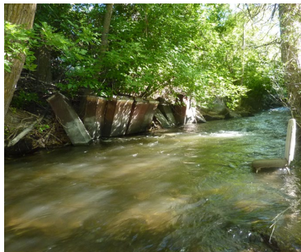
Kitchen riprap is common along Bozeman Creek.
