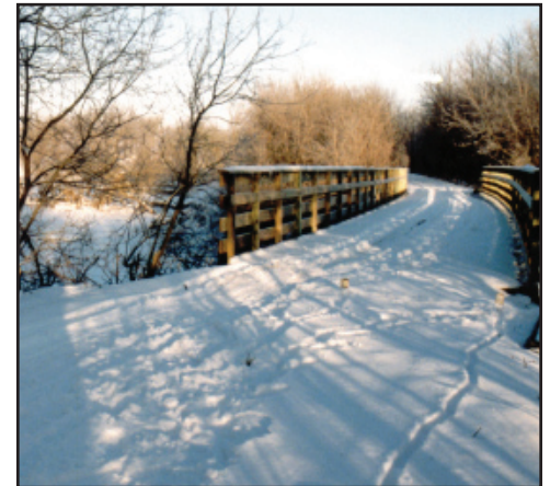
Curved bridge on the GRR Trail
