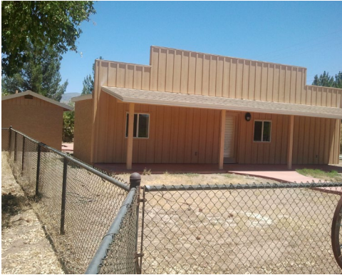
Black Canyon Heritage Park's renovated visitors center.
