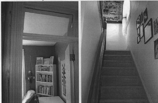
Left: maid's room, second story; right: stairwell. Photos taken by Elizabeth Kohlstaedi, December 2004.
