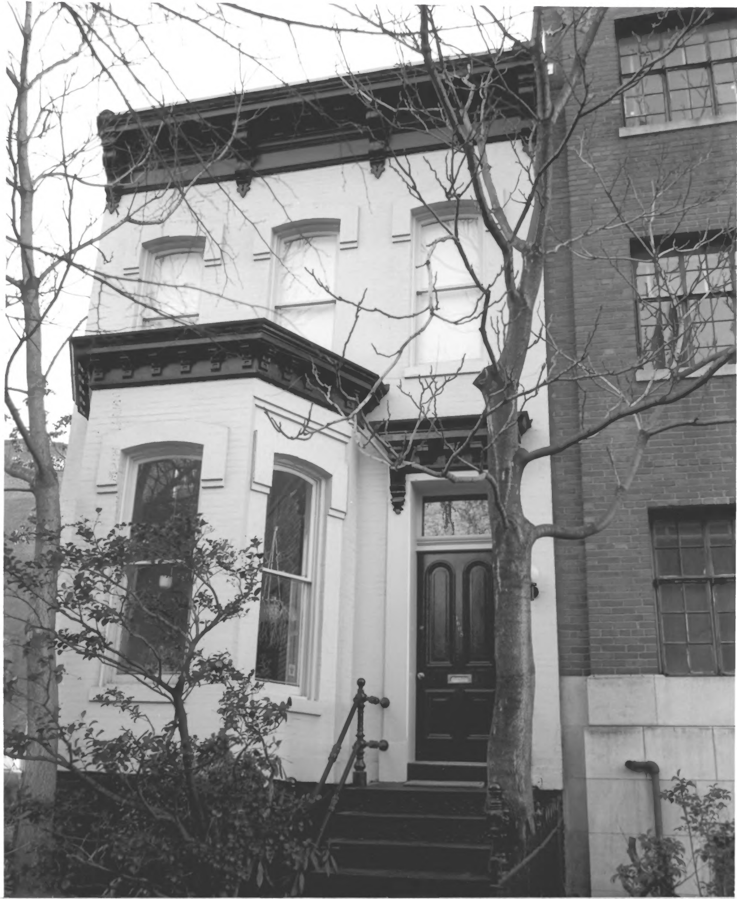
Charlotte Forten Grimke' House, Washington, D.C. Photo by W. Curtis Martin for the ABC North elevation, looking south 1976
