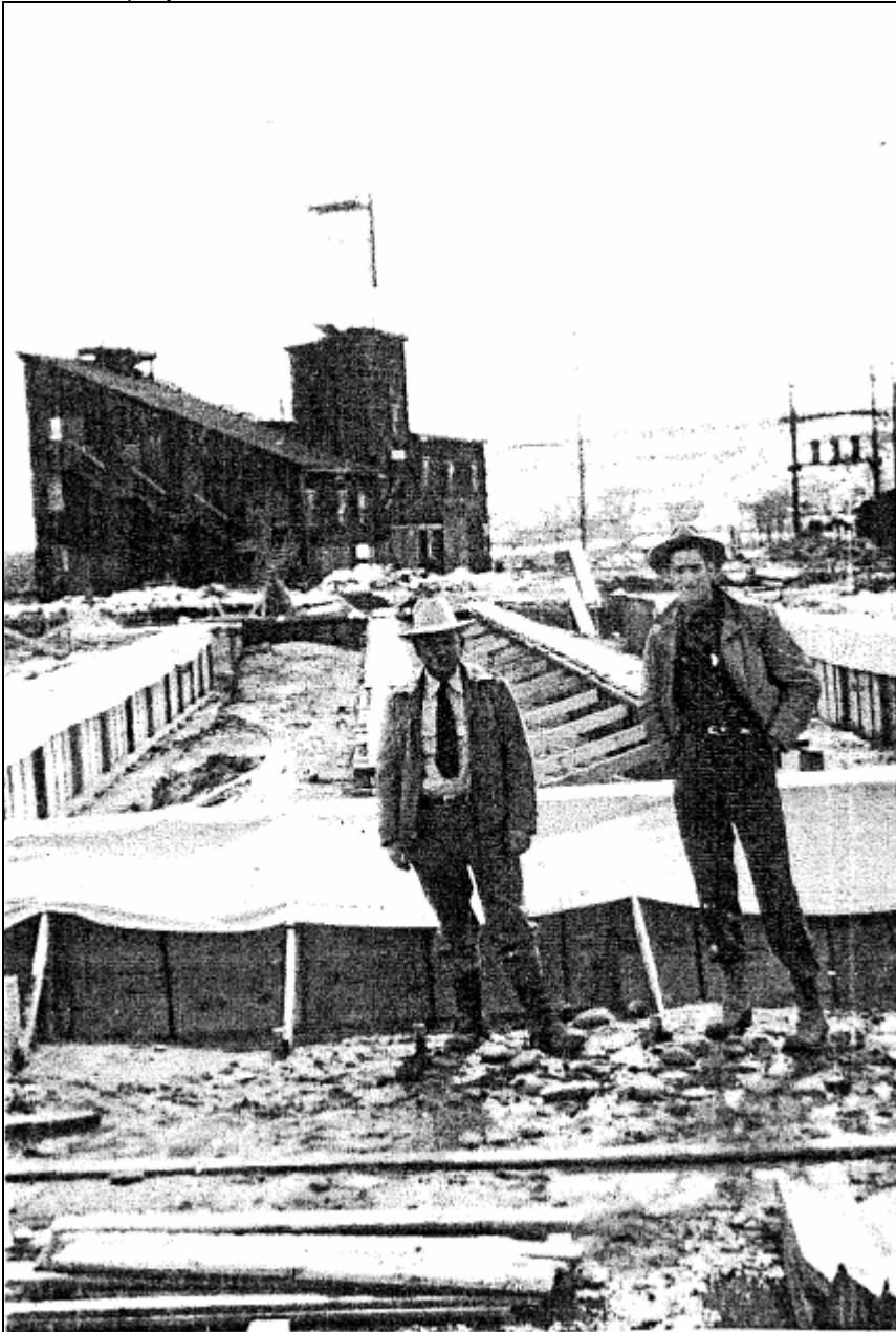
Historic Photo 3 1948 photograph of Building 12 under construction with the shell of the Manhattan Project refinery in the background.
