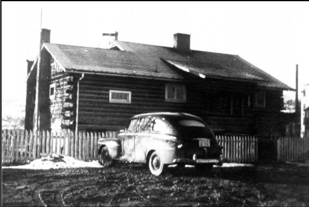
Historic Photo 1. Circa 1943 photograph of the log cabin office building surrounded by a picket fence. Note that the raised foundation can be seen through the fence. Photographer unknown, on file at the DOE Grand Junction Office, Grand Junction, Colorado.
