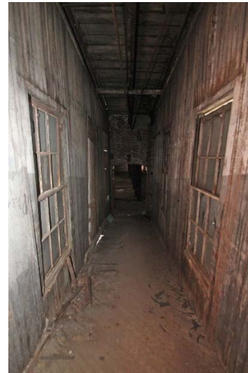
Photo 21 (left): Second floor of Mill #2, loft door on east elevation. As shown in this view, limited areas of the original diagonal wood floors have been patched with plywood and other materials. All other materials, such as the brick walls and heavy timber columns and ceiling, are original.
