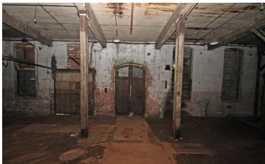
Photo 21 (left): Second floor of Mill #2, loft door on east elevation. As shown in this view, limited areas of the original diagonal wood floors have been patched with plywood and other materials. All other materials, such as the brick walls and heavy timber columns and ceiling, are original.
