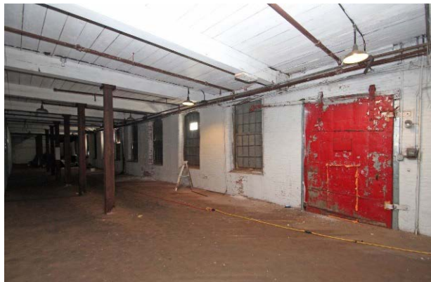
Photo 6 (left): First floor of Mill #1, view southeast. This view shows an area of partial replacement of the diagonally laid wood floors. All other materials, including the brick walls and heavy timber columns and beams are original (it is unknown when any of the walls and ceilings were painted). The original twelve-over-twelve windows are also visible in this view.
