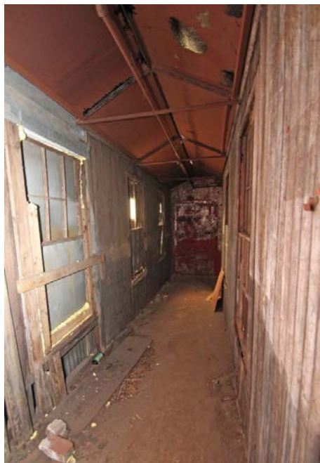
Photo 25 (left): Bridge between Mill #1 and Mill #2, fourth floor, view south. The original six-over-six, double-hung wood windows are visible in this view.
