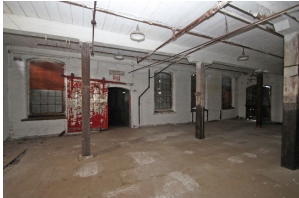
Photo 11 (left): Fourth floor of Mill #1, view northeast. In this view and in Photos 12-14, the wood floors, brick walls and heavy timber columns and beams are all original. Photo 12 (right): Fourth floor of Mill #1, view southwest. This view shows the arched openings into the bridges between Mill #1 and Mill #2. The openings contain period metal fire doors on each floor as seen in this image.
