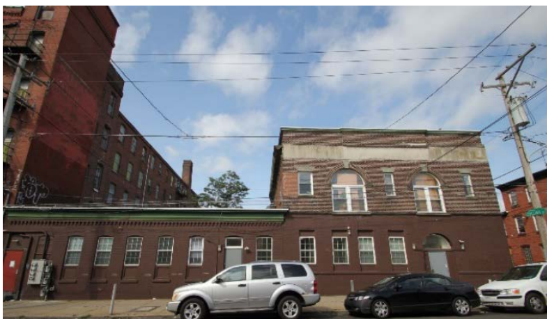
Photo 30: North elevation of the Warehouse, and the abutting Office. The stucco band above the second floor windows was historically the location of a cornice as seen in Figure E.
