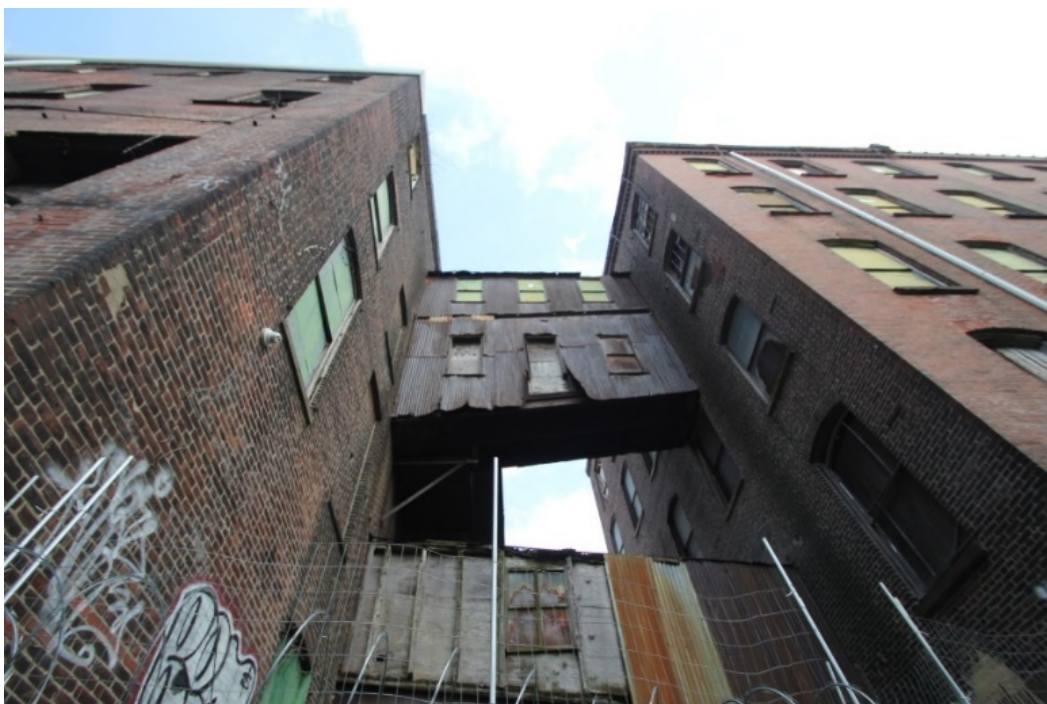
Photo 5: Bridges between Mill #1 (right) and Mill #2 (left), view west.
