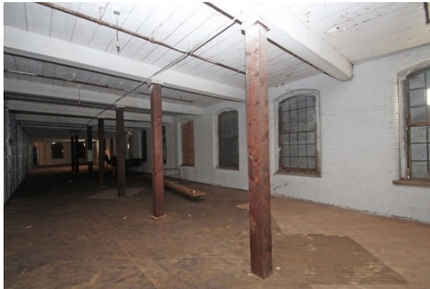
Photo 11 (left): Fourth floor of Mill #1, view northeast. In this view and in Photos 12-14, the wood floors, brick walls and heavy timber columns and beams are all original. Photo 12 (right): Fourth floor of Mill #1, view southwest. This view shows the arched openings into the bridges between Mill #1 and Mill #2. The openings contain period metal fire doors on each floor as seen in this image.
