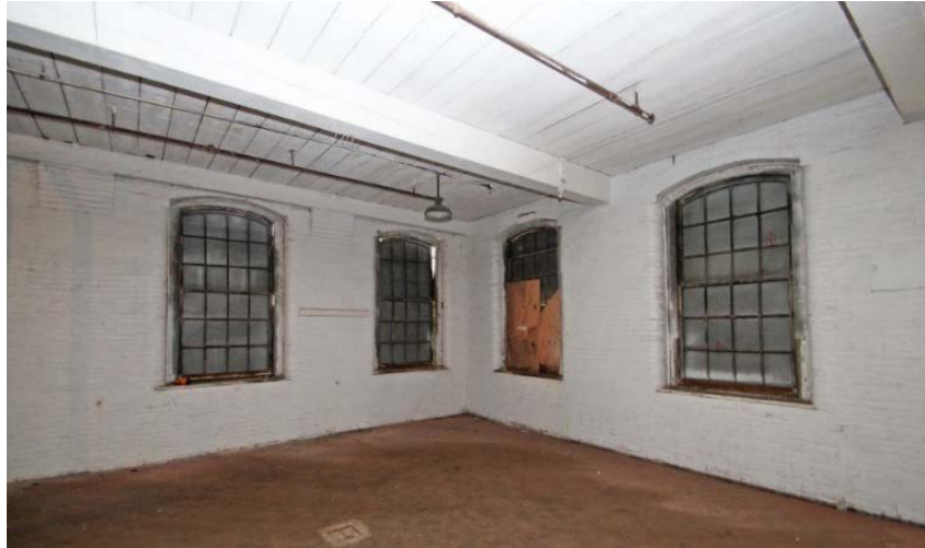
Photo 9 (left): Stair at the northeast corner of Mill #1, fourth floor, view south. This stair is original to Mill #1. Photo 10 (right): Fourth floor of Mill #1, view northeast. The wood floors, brick walls and heavy timber beams in this view are all original.
