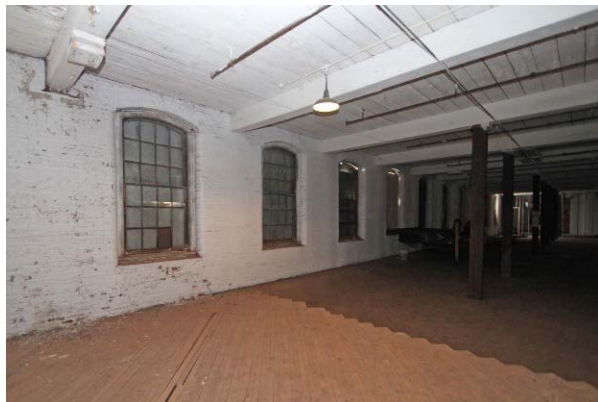
Photo 6 (left): First floor of Mill #1, view southeast. This view shows an area of partial replacement of the diagonally laid wood floors. All other materials, including the brick walls and heavy timber columns and beams are original (it is unknown when any of the walls and ceilings were painted). The original twelve-over-twelve windows are also visible in this view.
