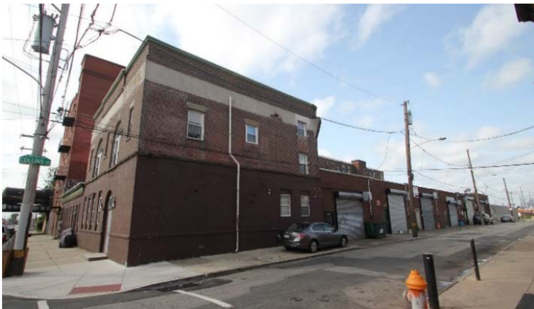
Photo 32: The Warehouse and garages, view southeast, from the Tioga-Collins Street corner.
