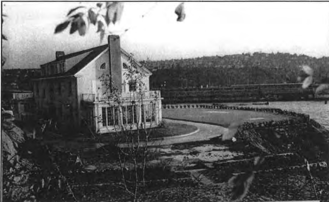
Photo B-6: The west elevation and garden, probably during landscape restoration following 1964 slide. (US Navy)
