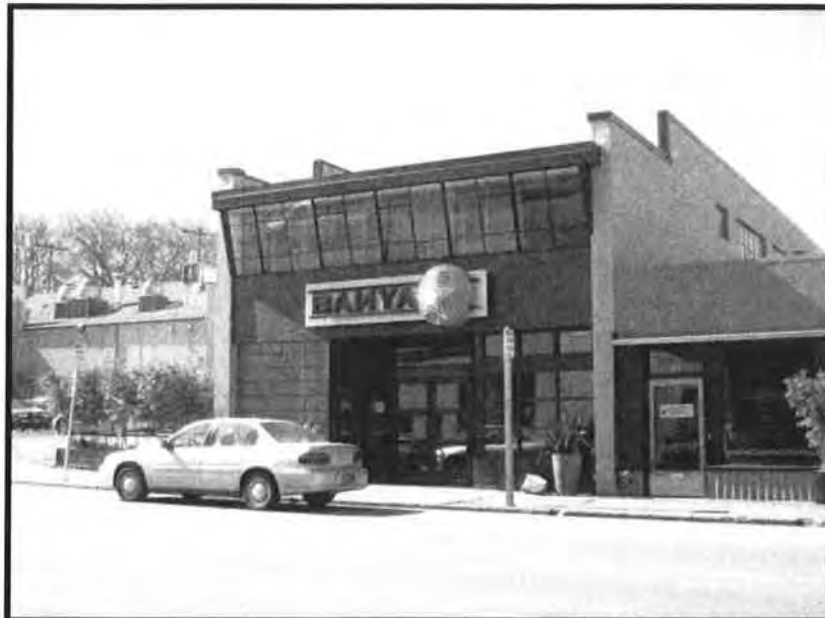
Photo C-36: The small building above (217 9 th Avenue N.), designed as an upholstery shop, has a notable Modernistic feature in the angled upper story glass. Gotteland designed this in 1946, shortly after the completion of Admiral's House.
