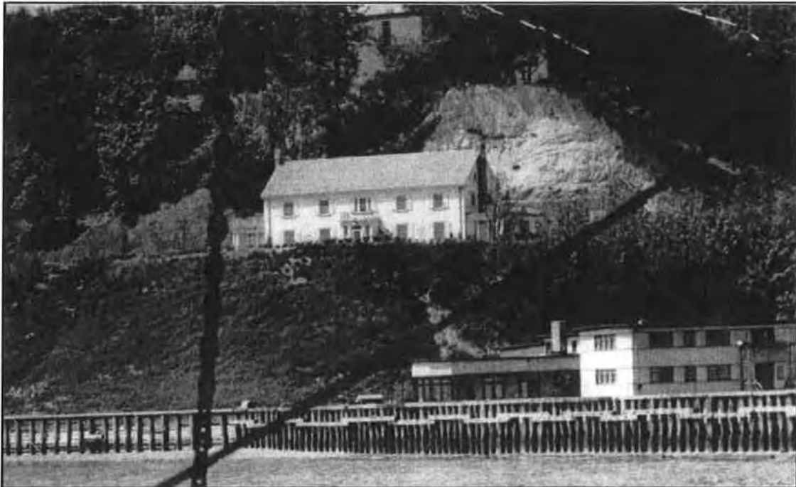
Photo B-7: Main facade, showing bare hillside following landslide; below are Navy buildings on the current park property, before W. Marina Place was constructed. (US Navy)
