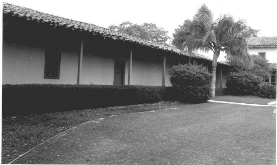
Los Cerritos Ranch House, 1844 South elevation of North Service Wing and West (Rear) elevation of Main House (Right)
