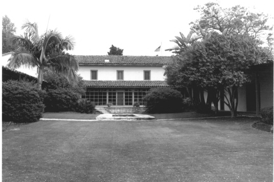
Los Cerritos Ranch House, 1844 West (Rear) Elevation of Main House, Patio and South Service Wing (Right)
