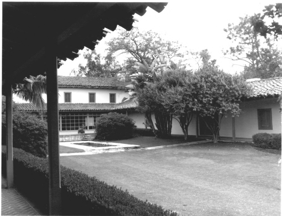
Los Cerritos Ranch House, 1844 West (Rear) Elevation of main house and north elevation of south service wing
