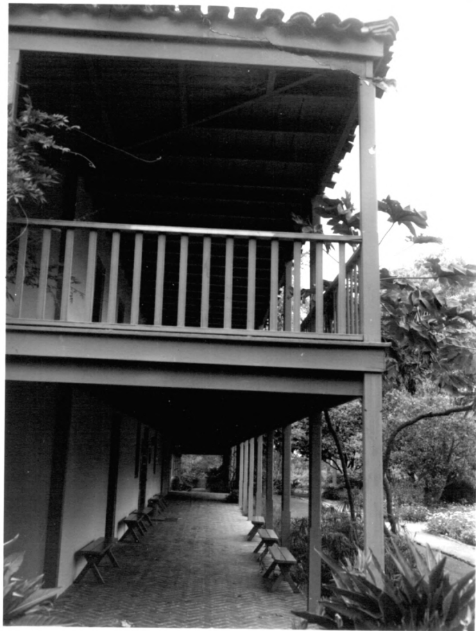
Los Cerritos Ranch House, 1844 East (front) elevation, looking north along veranda
