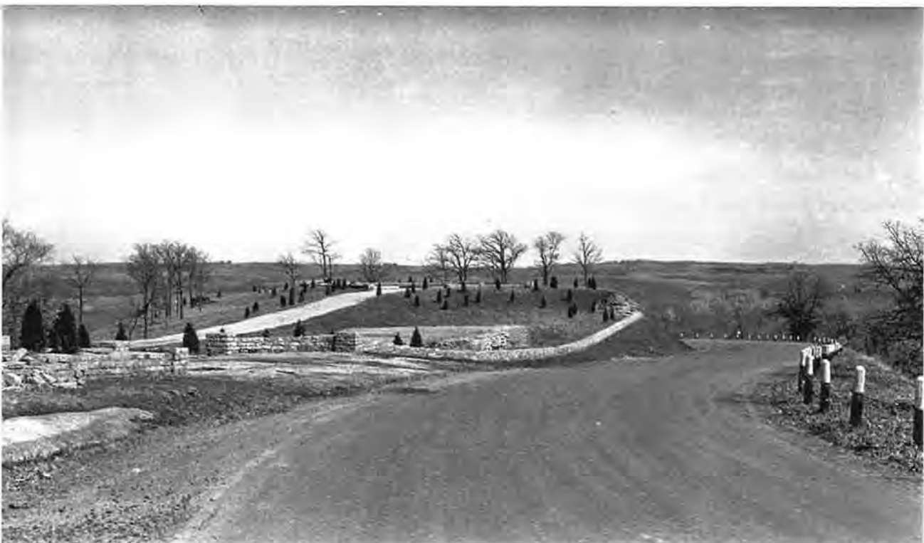
Figure 5. By approximately spring 1937 when this photo was taken by A. R. Nichols the South Wall had been reconstructed to be continuous and to skirt the outcrop rather than being interrupted by it. (Compare to Figure 3.) The change required removing about 10 feet from the south edge of the outcrop and tearing out and rebuilding about 25 feet of wall immediately west of the outcrop to make the two wall pieces meet. Note that part of the west segment of the South Wall is awaiting reconstruction at the left edge of the photo. (Minnesota Department of Transportation collection, Audio-Visual Materials (neg. 41-17), Minnesota Historical Society, St. Paul.)
