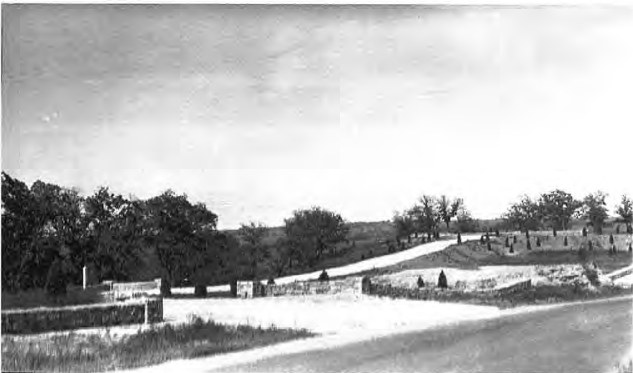
Figure 3. Photo of the wayside rest taken circa 1936, in about mid-summer, by designer A. R. Nichols. (The photo in Figure 4 is approximately the same age.) The Parking Bay, with a surveyor's rod, is at left. The South Wall east of the entrance has been built to incorporate a preserved stone outcrop. This was evidently unsatisfactory (note, for example, the elevation difference in the two wall segments) and was redesigned (see Figure 4). It is believed the trees were installed in the spring of either 1935 or 1936. (Minnesota Department of Transportation collection, Audio-Visual Materials (neg. 41-12), Minnesota Historical Society, St. Paul.)
