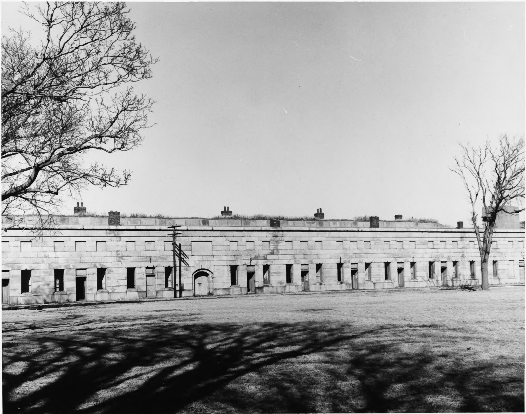
Fort Warren, interior looking toward Front No. 2, Massachusetts
