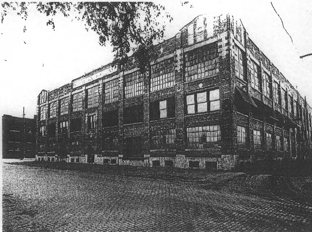
CHERRY-BURRELL BUILDINGS, (LEFT) WAREHOUSE, (RIGHT) FACTORY
