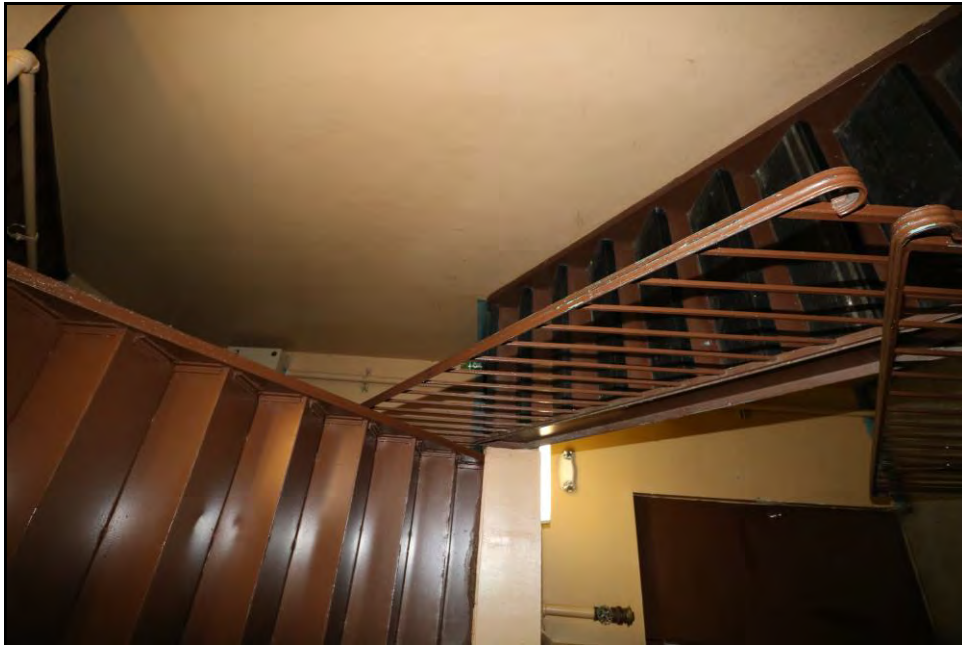
Photo 8. Everett Court Apartments, Second Floor, Typical Stairwell, view looking north.
