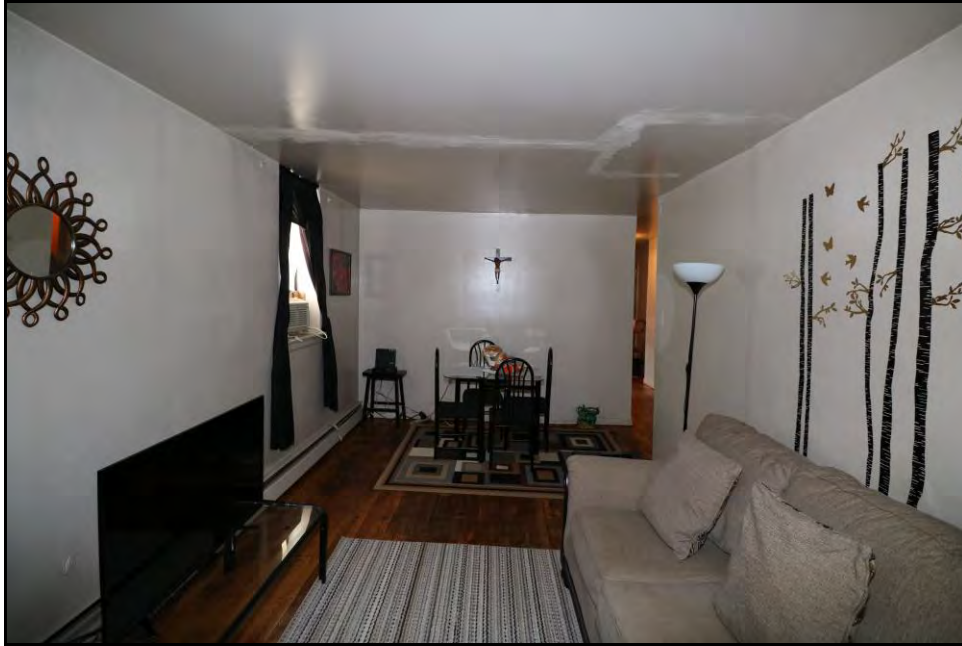
Photo 9. Everett Court Apartments, Fourth Floor, Typical Apartment, view looking south.
