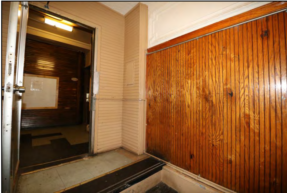
Photo 6. Everett Court Apartments, First Floor, Entrance Vestibule, view looking northeast.
