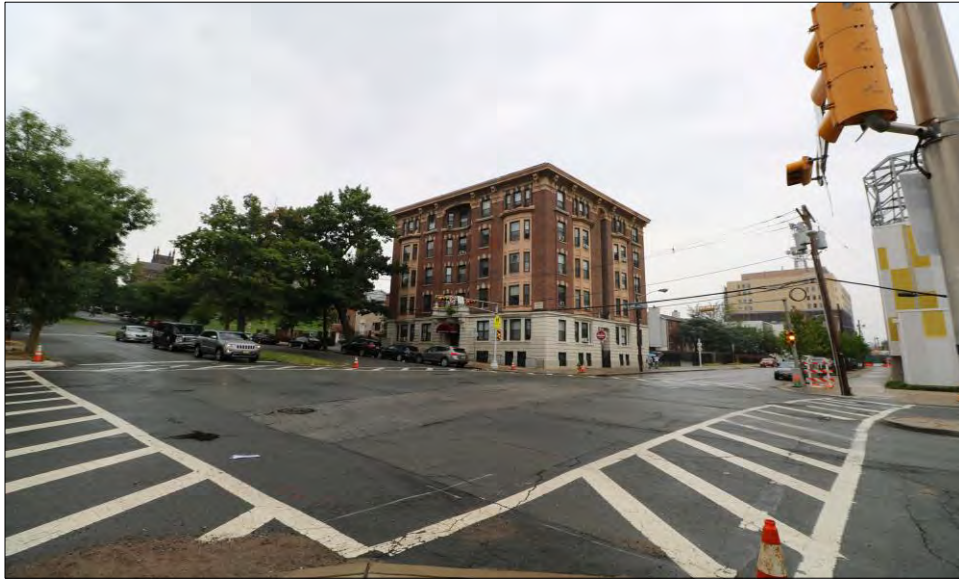
Photo 1. Everett Court Apartments, South and East Elevations, view looking northwest.
