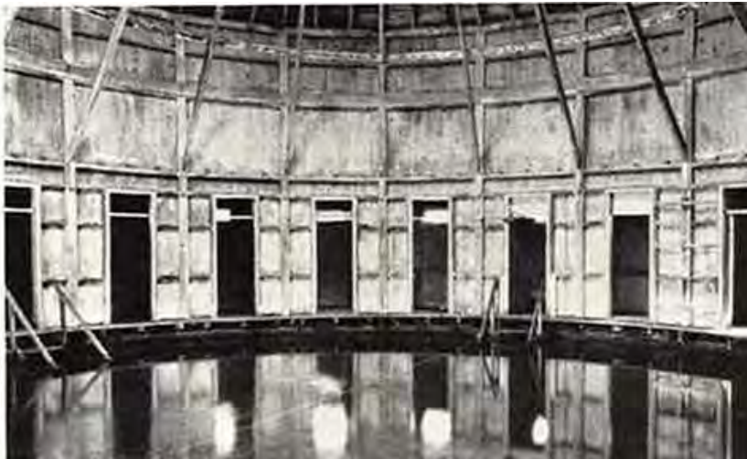
Interior of Ladies’ Bath before repairs, no date, from hotel brochure.
