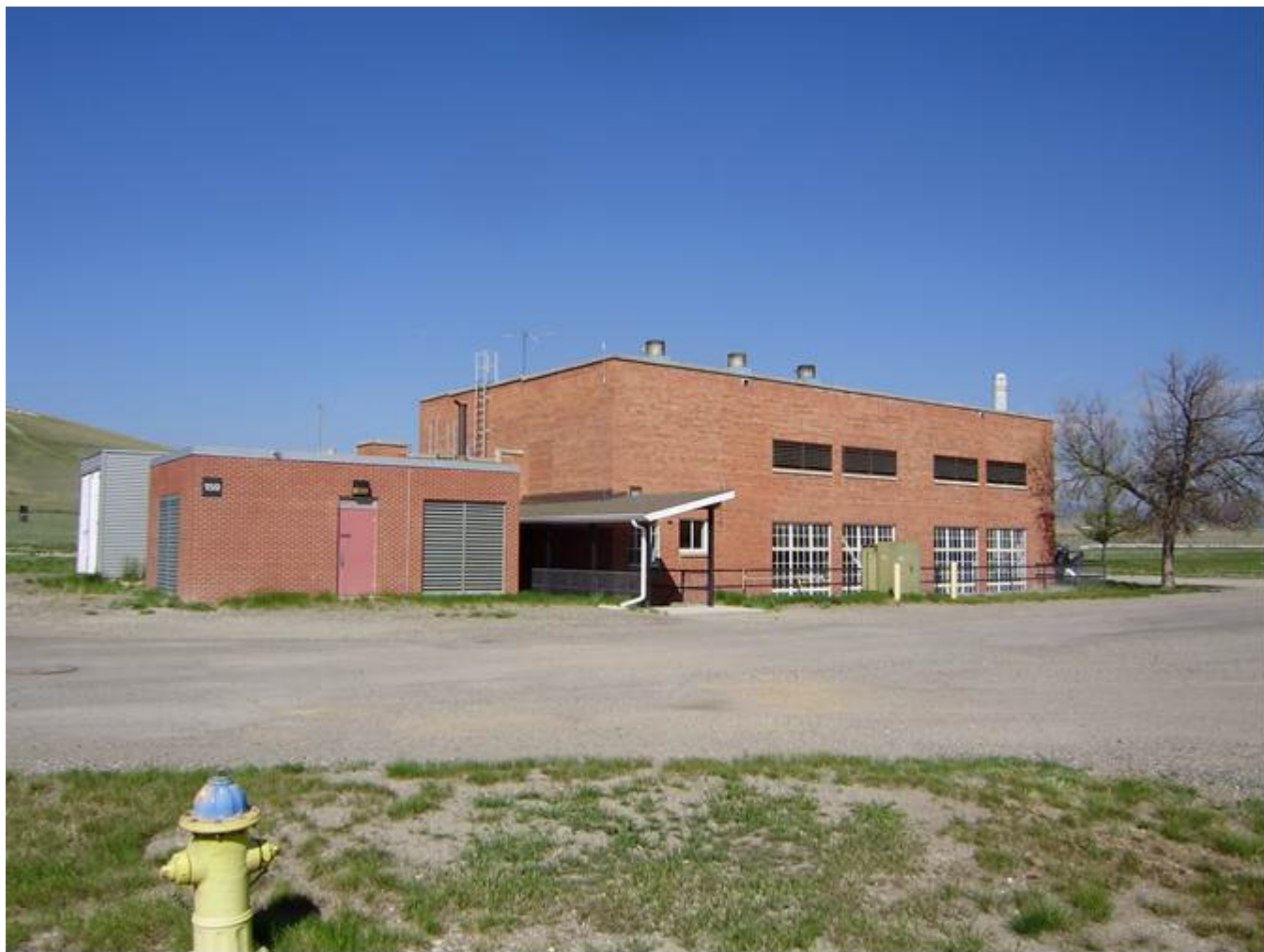
MT_LewisandClarkCounty_FortHarrisonVAHospitalHistoricDistrict_0056. Building 142. View to the northwest.
