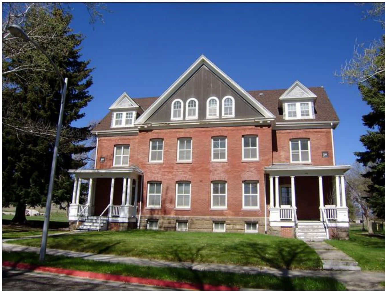
MT_LewisandClarkCounty_FortHarrisonVAHospitalHistoricDistrict_0010. Building 5. View to the west.
