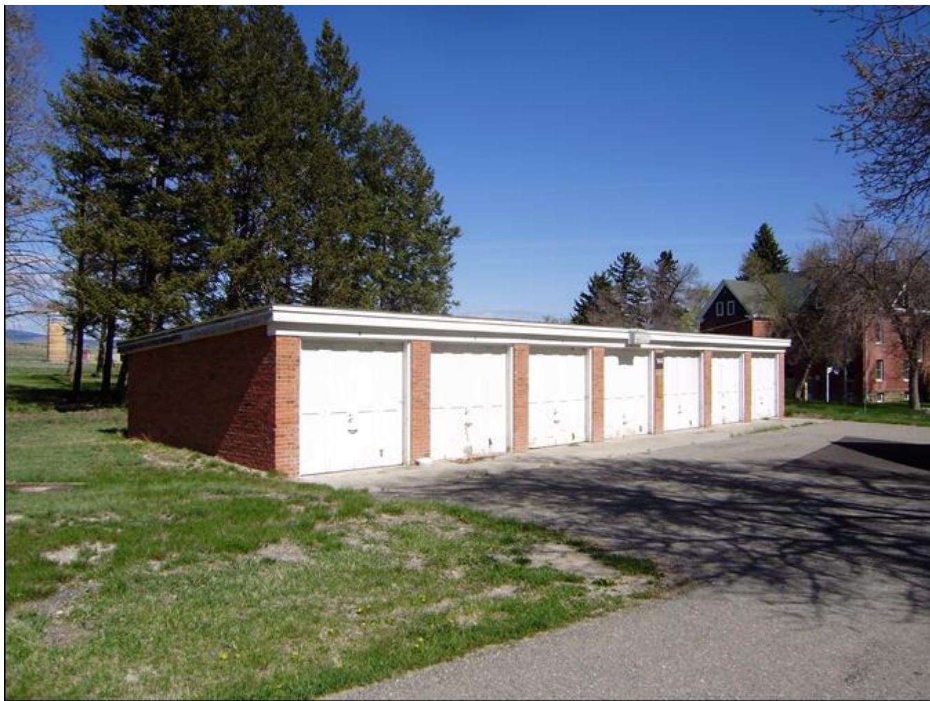
MT_LewisandClarkCounty_FortHarrisonVAHospitalHistoricDistrict_0058. Building 144. View to the north.
