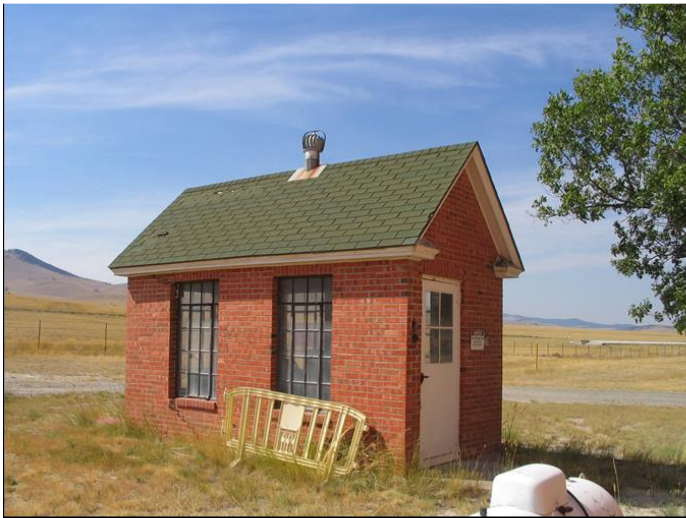
MT_LewisandClarkCounty_FortHarrisonVAHospitalHistoricDistrict_0064. Building 151. View to the northwest.
