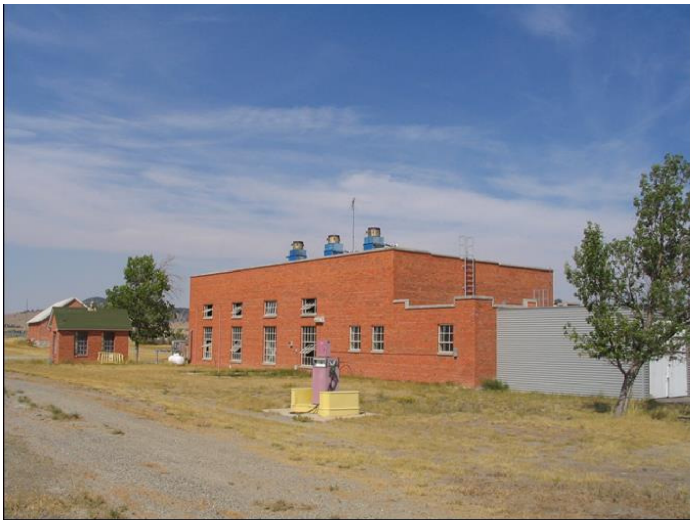
MT_LewisandClarkCounty_FortHarrisonVAHospitalHistoricDistrict_0057. Building 142. View to the northwest.
