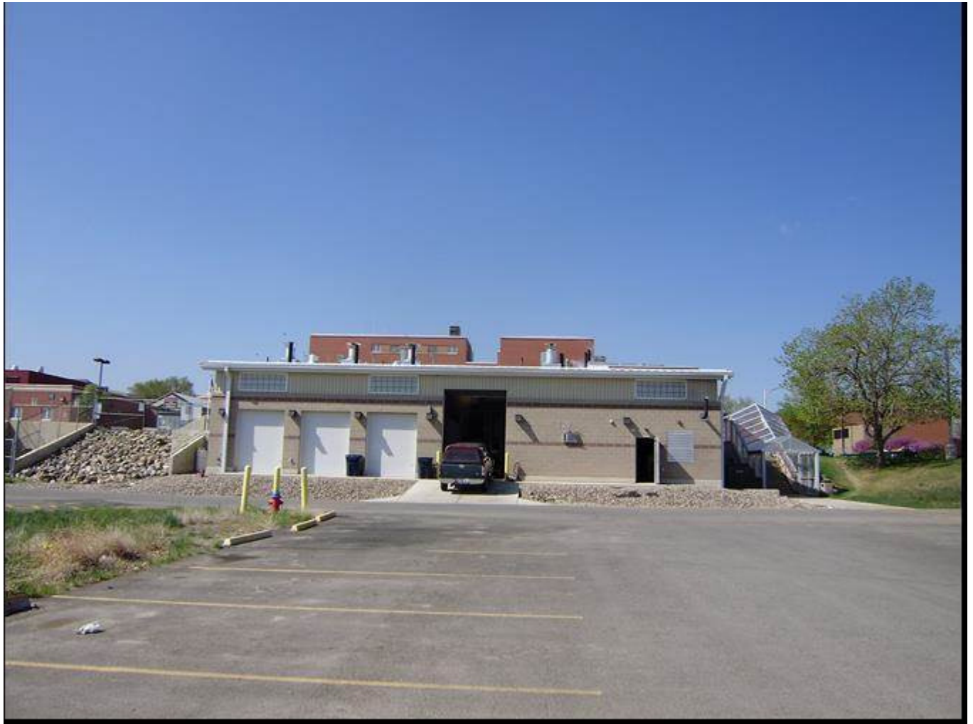
MT_LewisandClarkCounty_FortHarrisonVAHospitalHistoricDistrict_0081. Building 171. View to the south.
