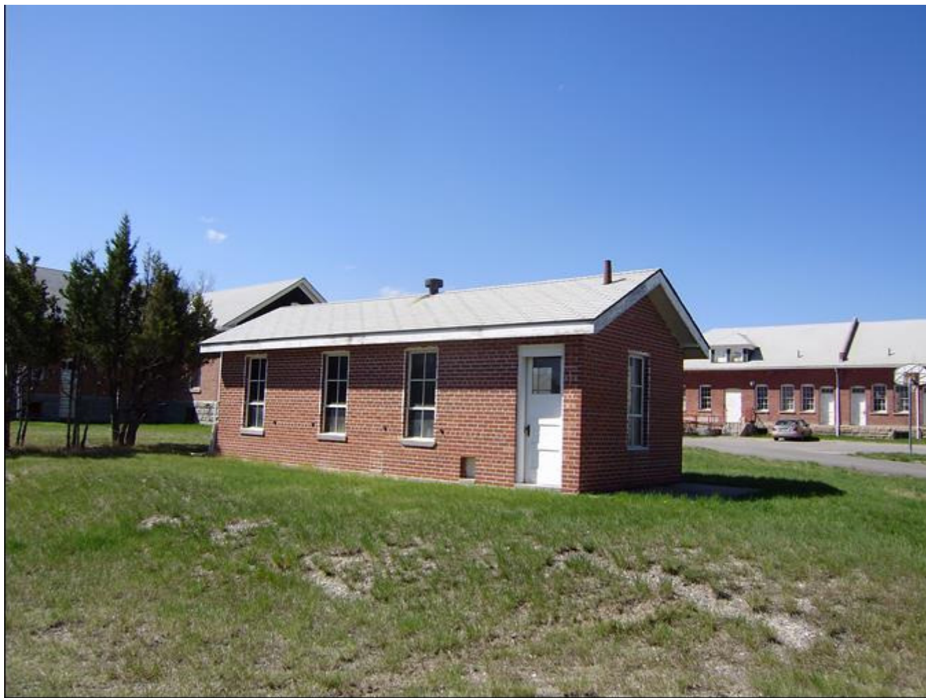
MT_LewisandClarkCounty_FortHarrisonVAHospitalHistoricDistrict_0049. Building 54. View to the southwest.
