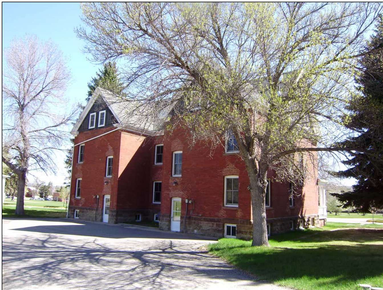
MT_LewisandClarkCounty_FortHarrisonVAHospitalHistoricDistrict_0009. Building 4. View to the northeast.
