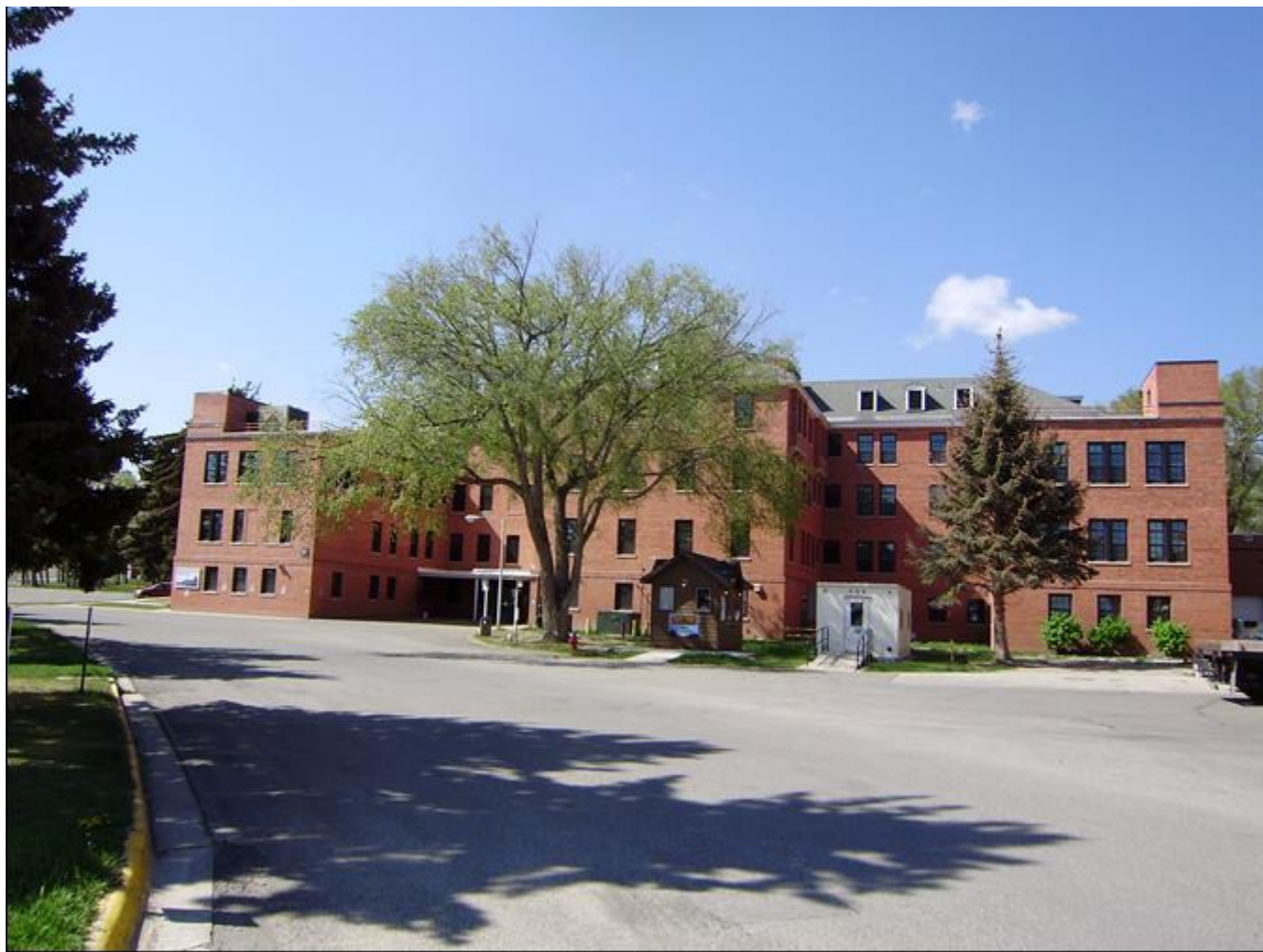
MT_LewisandClarkCounty_FortHarrisonVAHospitalHistoricDistrict_0055. Building 141. View to the south.
