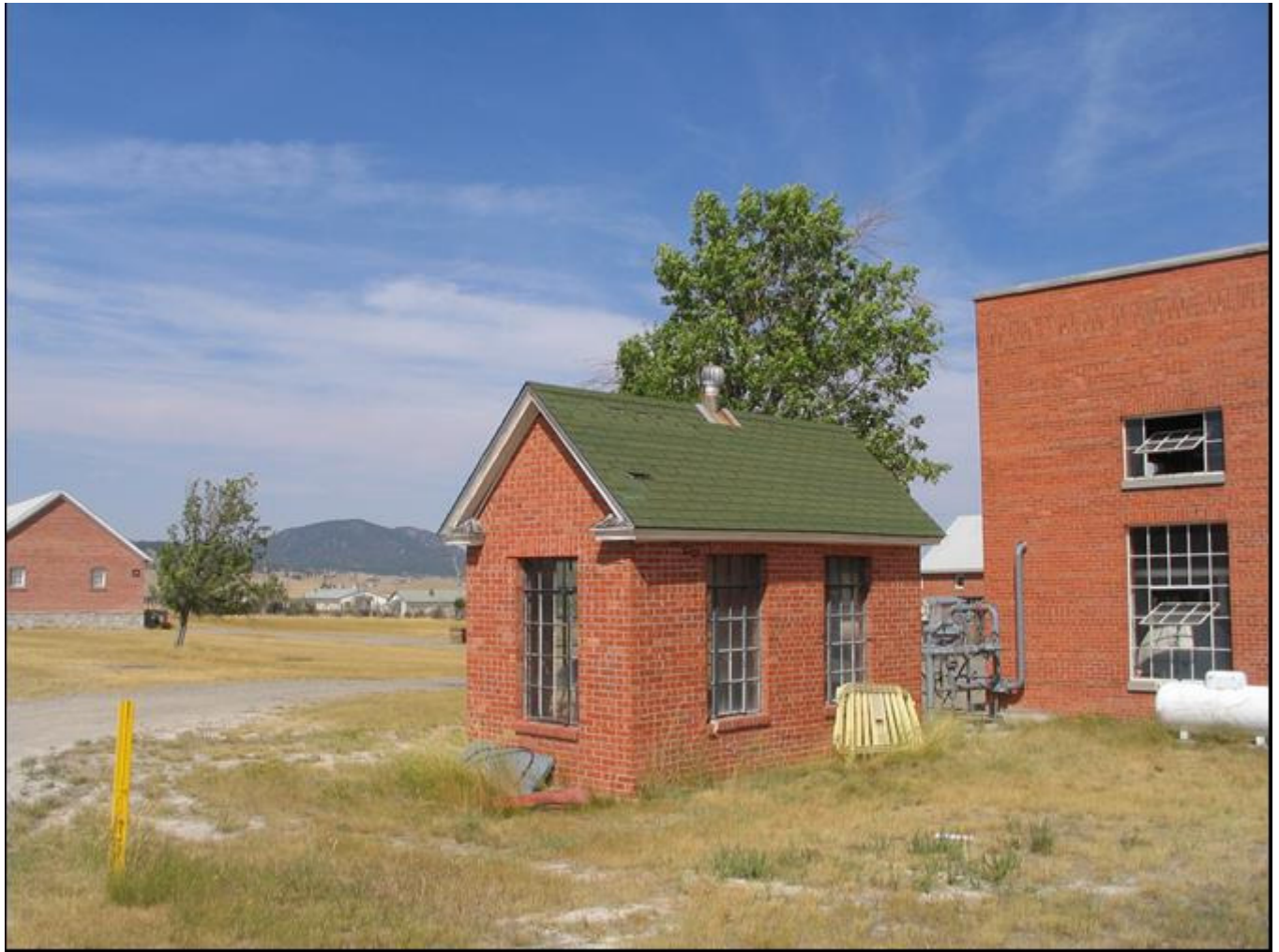
MT_LewisandClarkCounty_FortHarrisonVAHospitalHistoricDistrict_0065. Building 151. View to the northeast.
