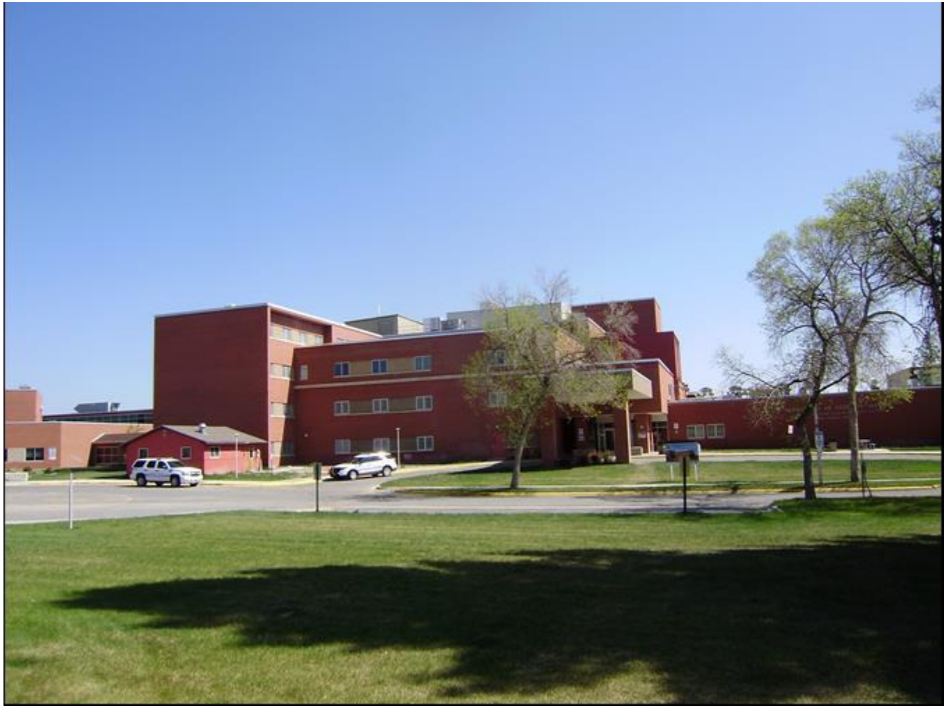
MT_LewisandClarkCounty_FortHarrisonVAHospitalHistoricDistrict_0068. Building 154. View to the north.
