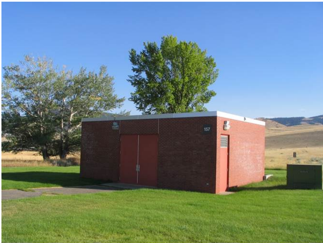
MT_LewisandClarkCounty_FortHarrisonVAHospitalHistoricDistrict_0071. Building 157. View to the south.
