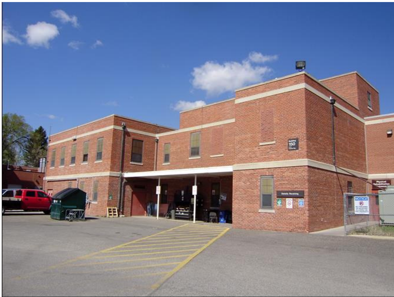
MT_LewisandClarkCounty_FortHarrisonVAHospitalHistoricDistrict_0063. Building 150. View to the southwest.
