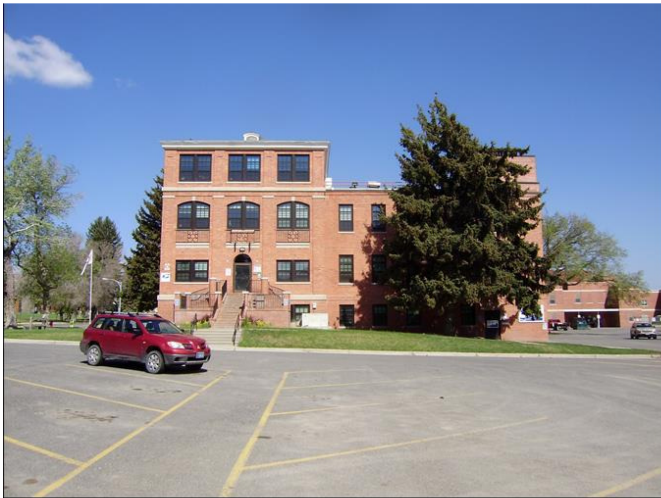
MT_LewisandClarkCounty_FortHarrisonVAHospitalHistoricDistrict_0053. Building 141. View to the west.
