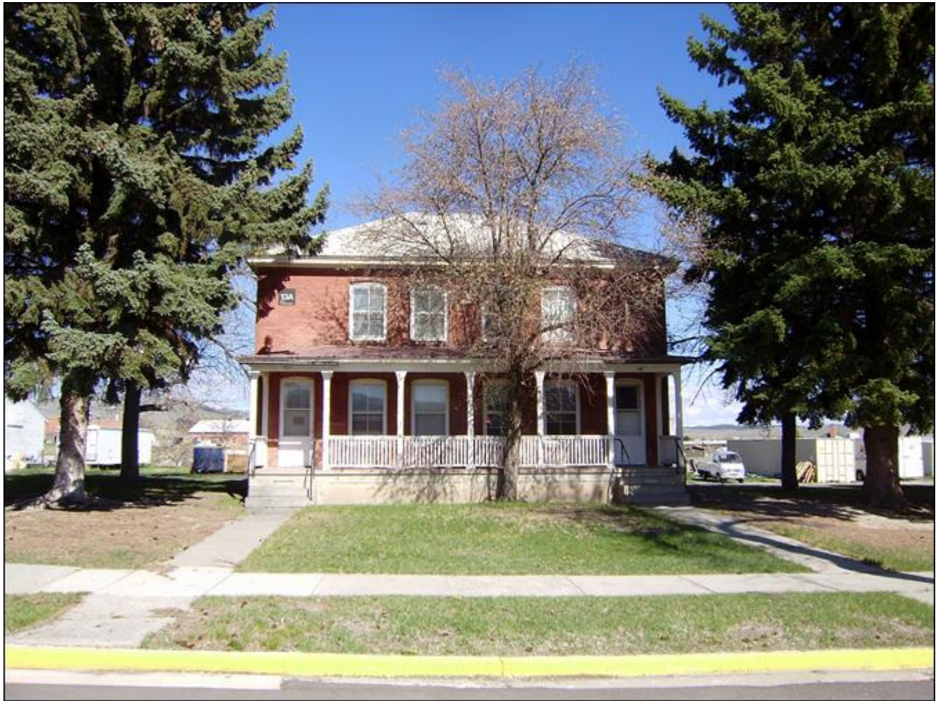
MT_LewisandClarkCounty_FortHarrisonVAHospitalHistoricDistrict_0016. Building 13. View to the west.
