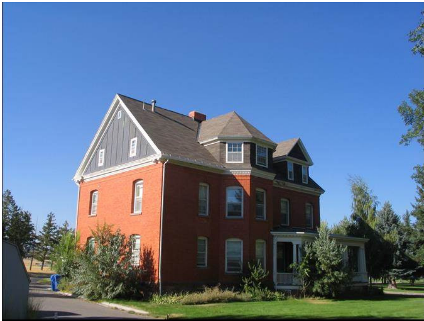
MT_LewisandClarkCounty_FortHarrisonVAHospitalHistoricDistrict_0031. Building 35. View to the northwest.
