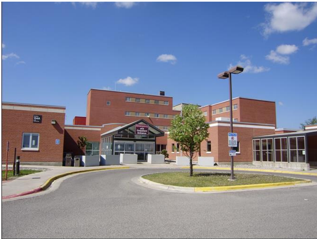
MT_LewisandClarkCounty_FortHarrisonVAHospitalHistoricDistrict_0070. Building 154A. View to the south.
