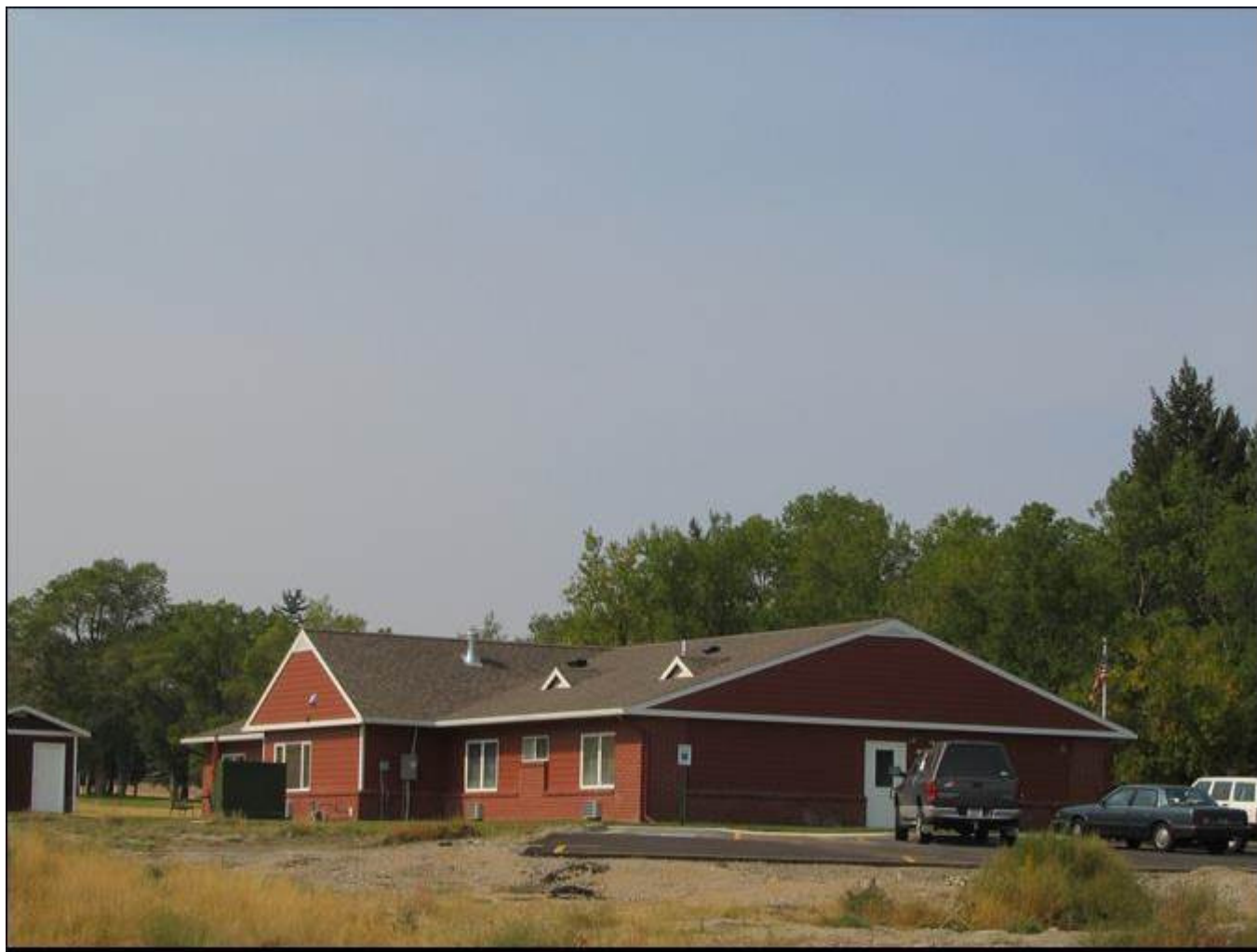
MT_LewisandClarkCounty_FortHarrisonVAHospitalHistoricDistrict_0077. Building 168. View to the WNW.
