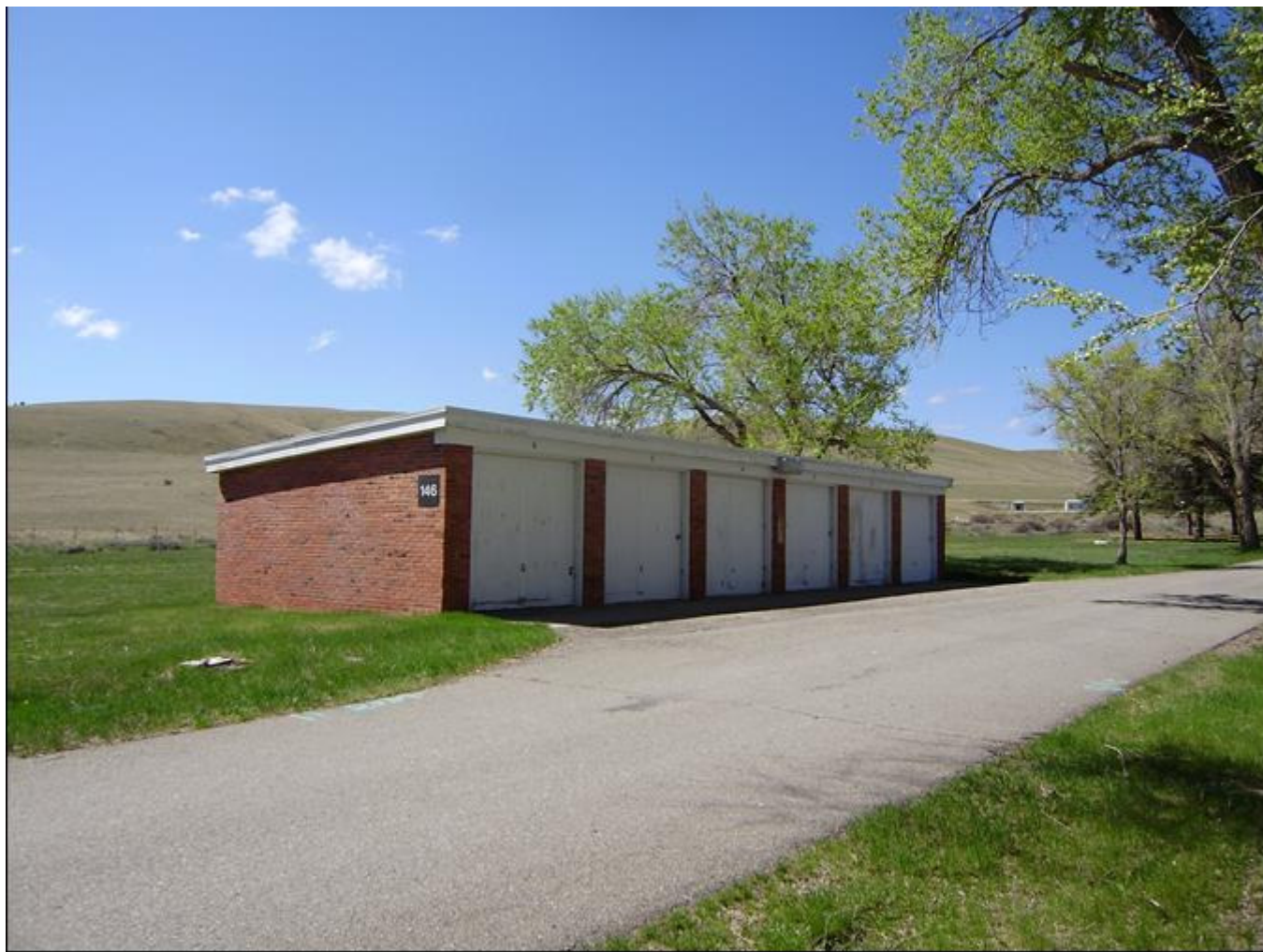
MT_LewisandClarkCounty_FortHarrisonVAHospitalHistoricDistrict_0060. Building 146. View to the southwest.
