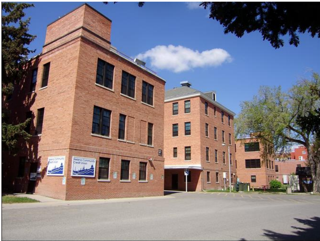
MT_LewisandClarkCounty_FortHarrisonVAHospitalHistoricDistrict_0054. Building 141. View to the southwest.
