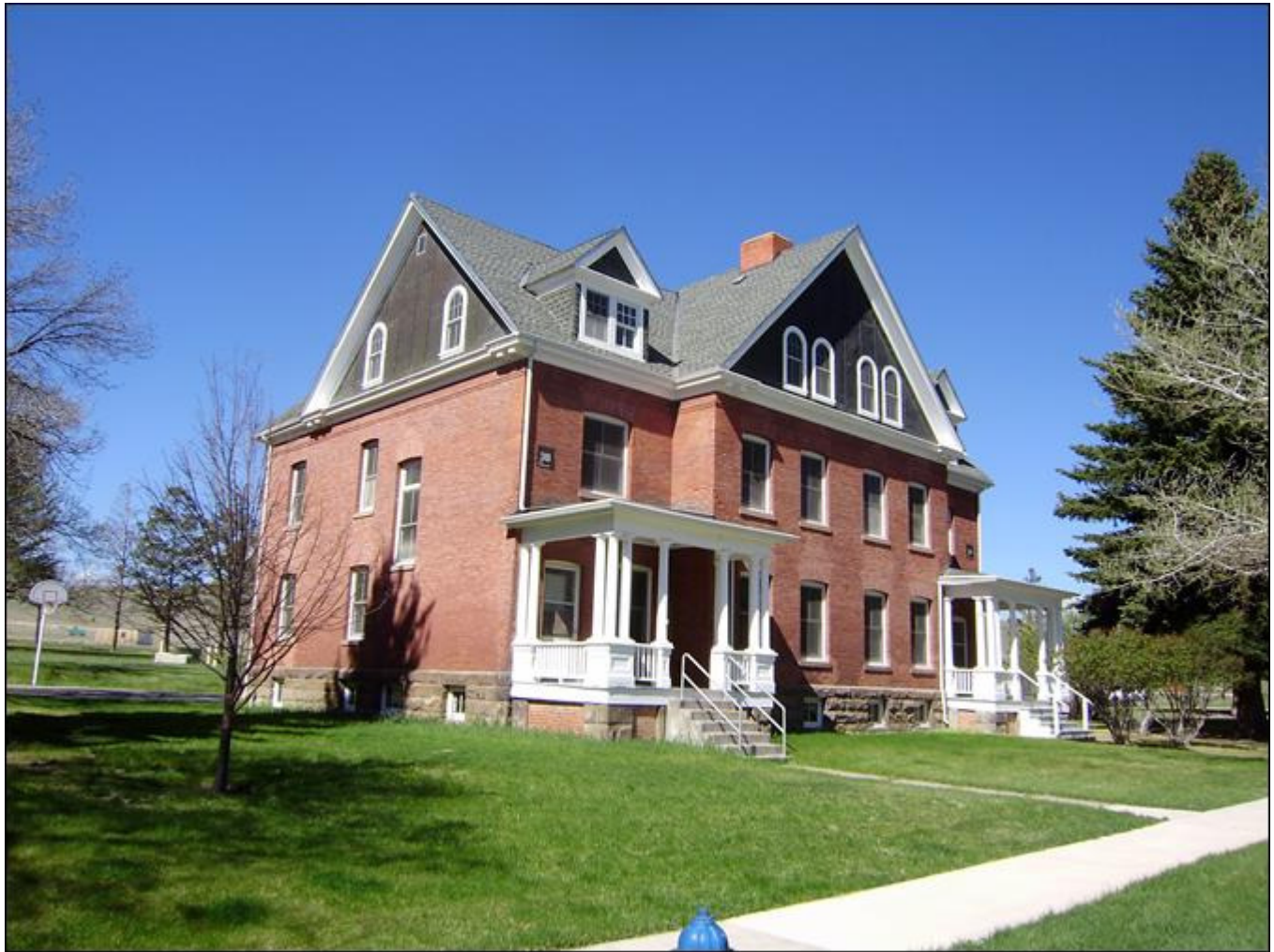
MT_LewisandClarkCounty_FortHarrisonVAHospitalHistoricDistrict_0006. Building 3. View to the NNW.
