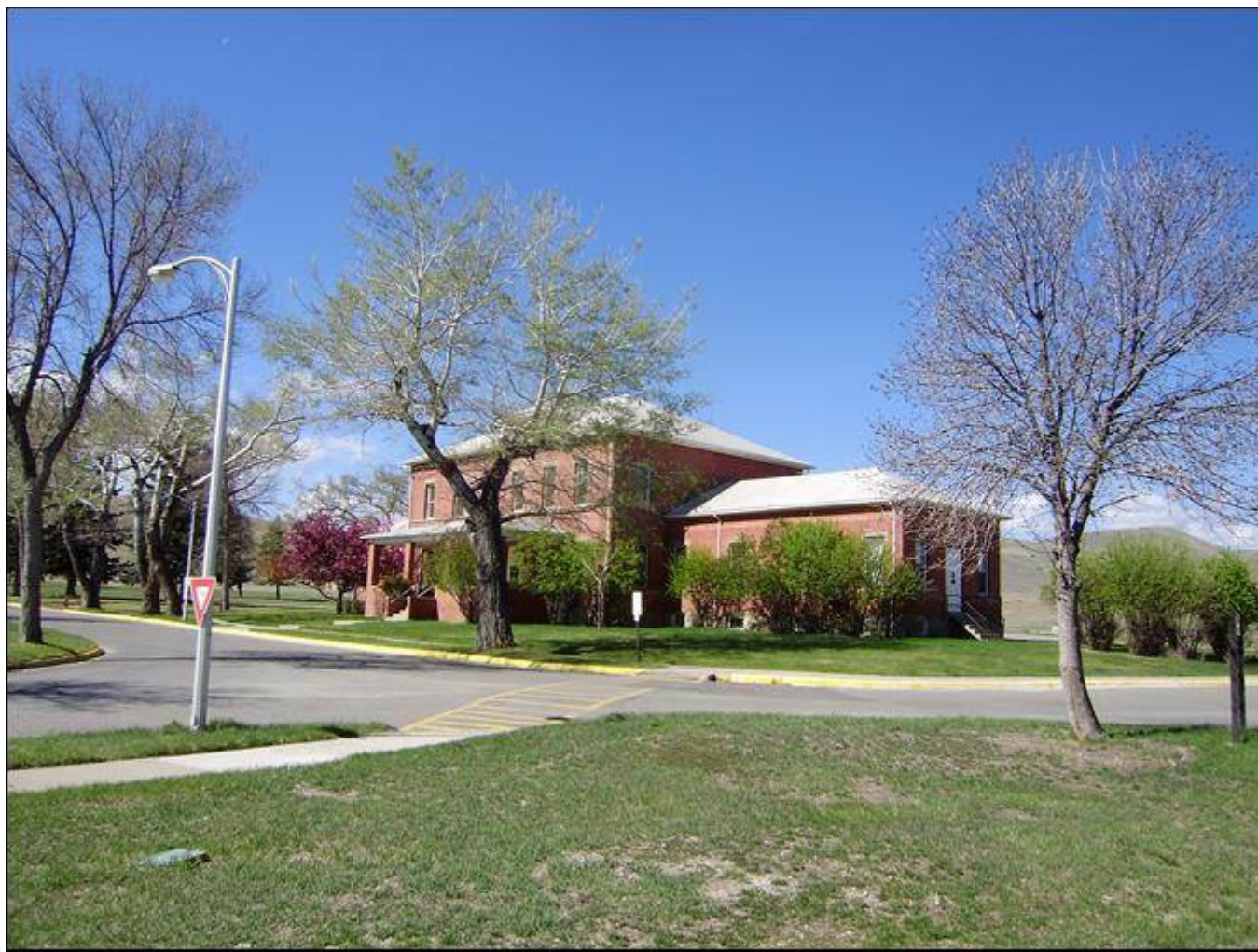
MT_LewisandClarkCounty_FortHarrisonVAHospitalHistoricDistrict_0001. Building 2. View to the southwest.
