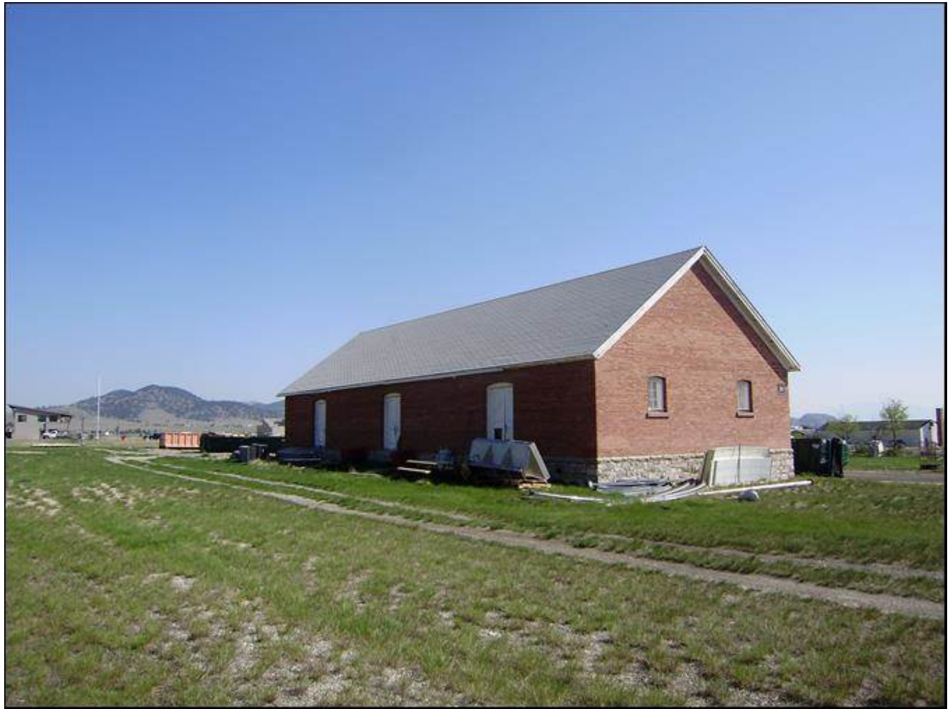
MT_LewisandClarkCounty_FortHarrisonVAHospitalHistoricDistrict_0029. Building 31. View to the northeast.
