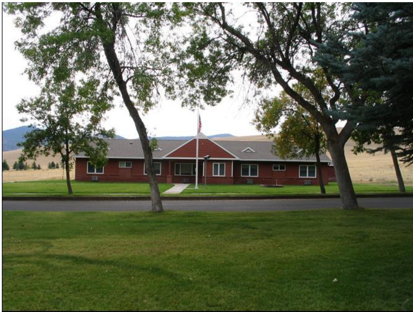
MT_LewisandClarkCounty_FortHarrisonVAHospitalHistoricDistrict_0078. Building 168. View to the south.
