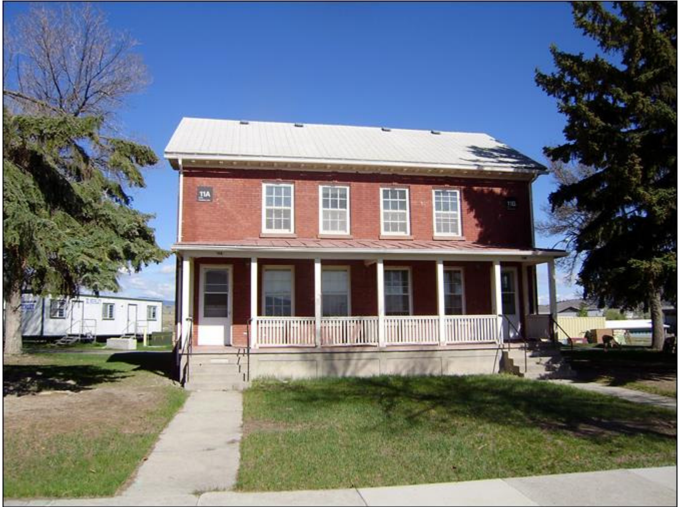
MT_LewisandClarkCounty_FortHarrisonVAHospitalHistoricDistrict_0012. Building 11. View to the west.
