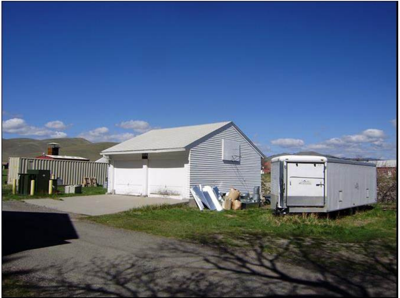
MT_LewisandClarkCounty_FortHarrisonVAHospitalHistoricDistrict_0082. Building 604. View to the southwest.
