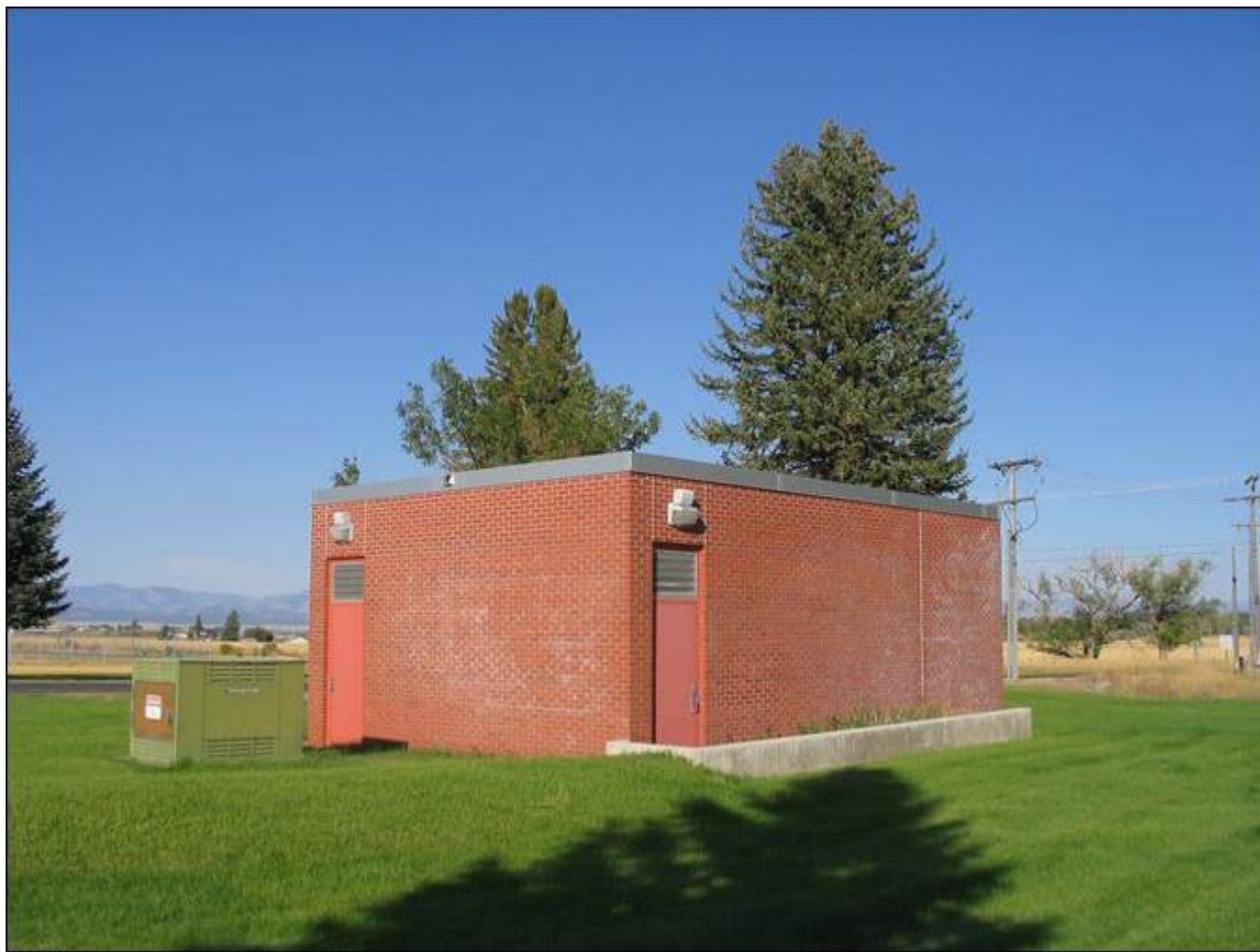
MT_LewisandClarkCounty_FortHarrisonVAHospitalHistoricDistrict_0072. Building 157. View to the northeast.
