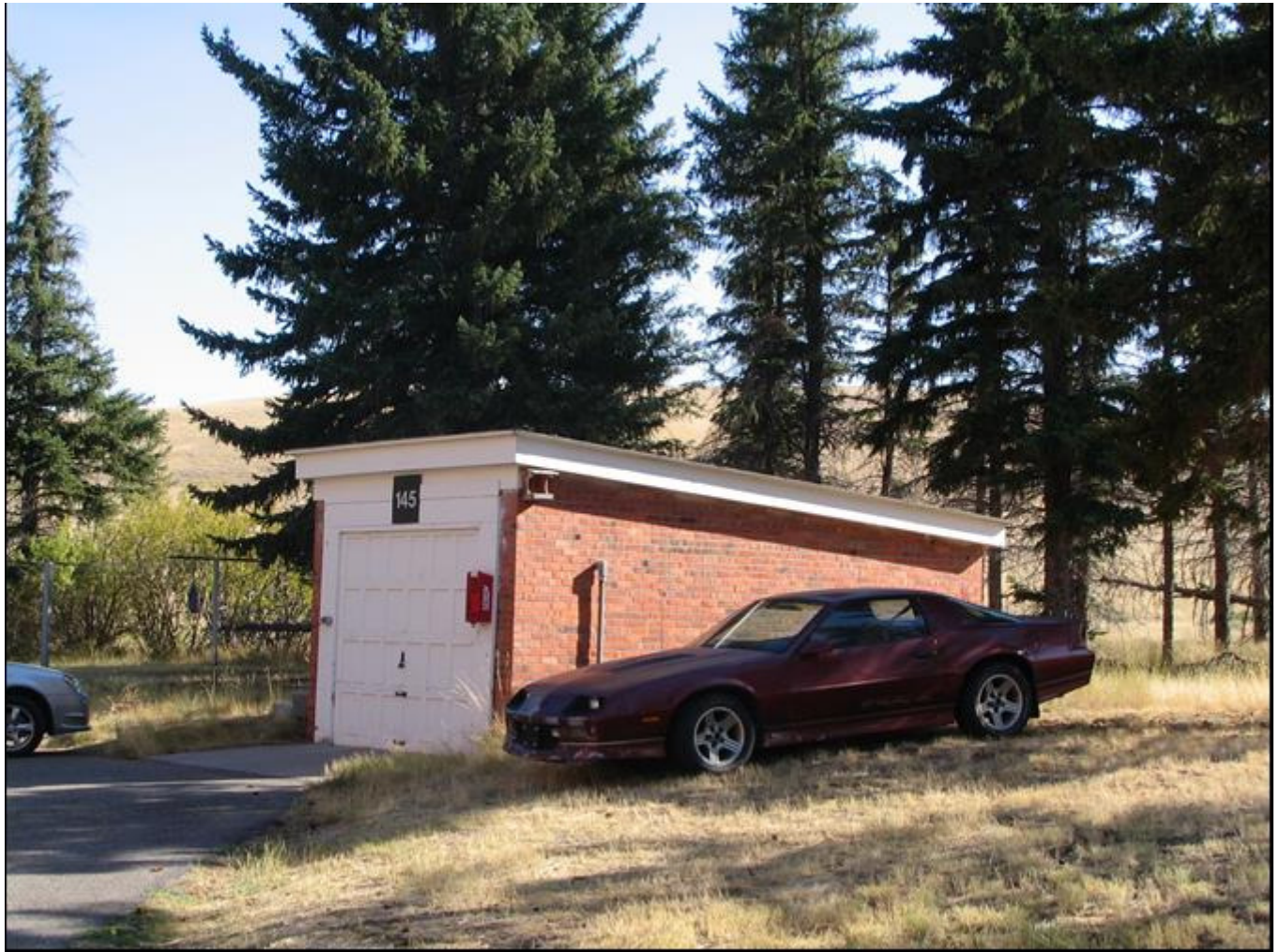
MT_LewisandClarkCounty_FortHarrisonVAHospitalHistoricDistrict_0059. Building 145. View to the south.
