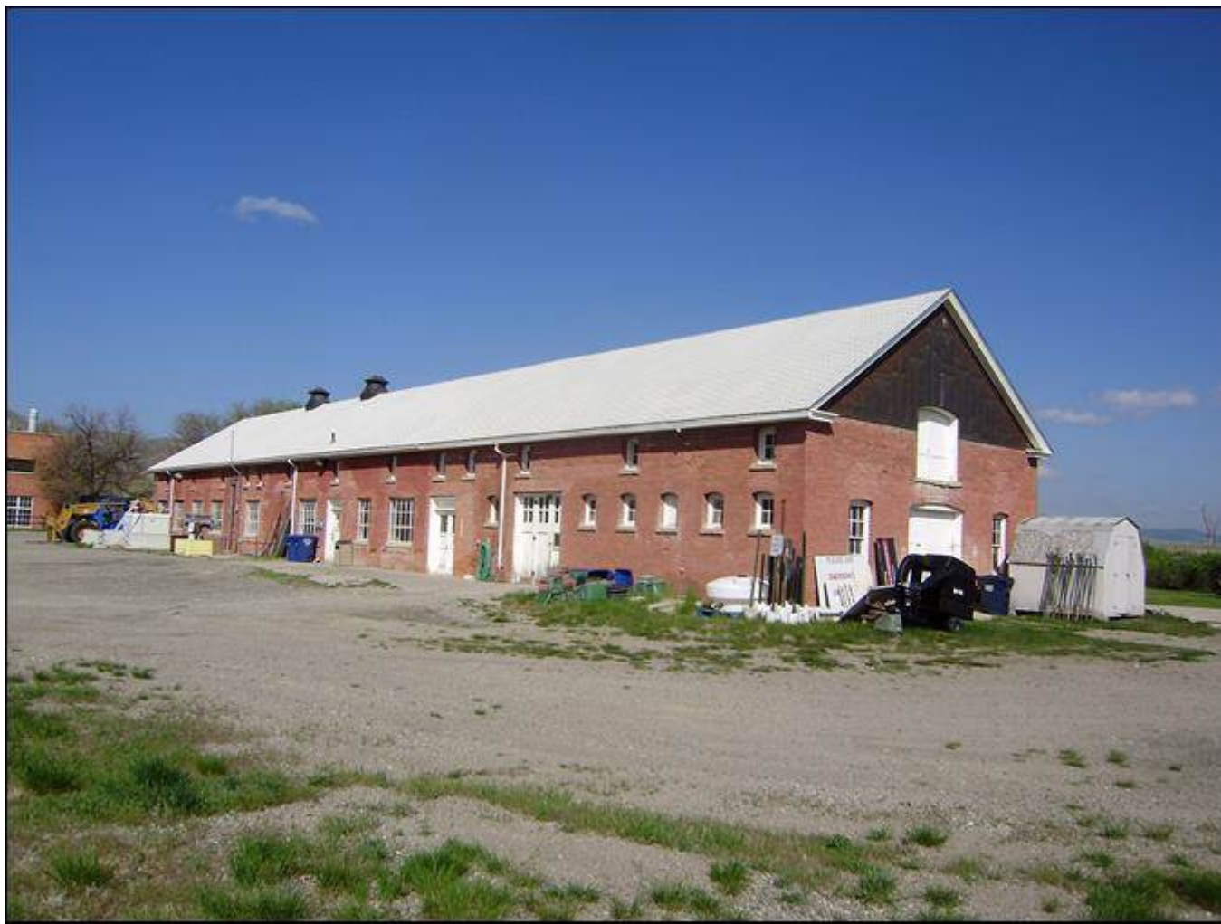
MT_LewisandClarkCounty_FortHarrisonVAHospitalHistoricDistrict_0026. Building 20. View to the northwest.
