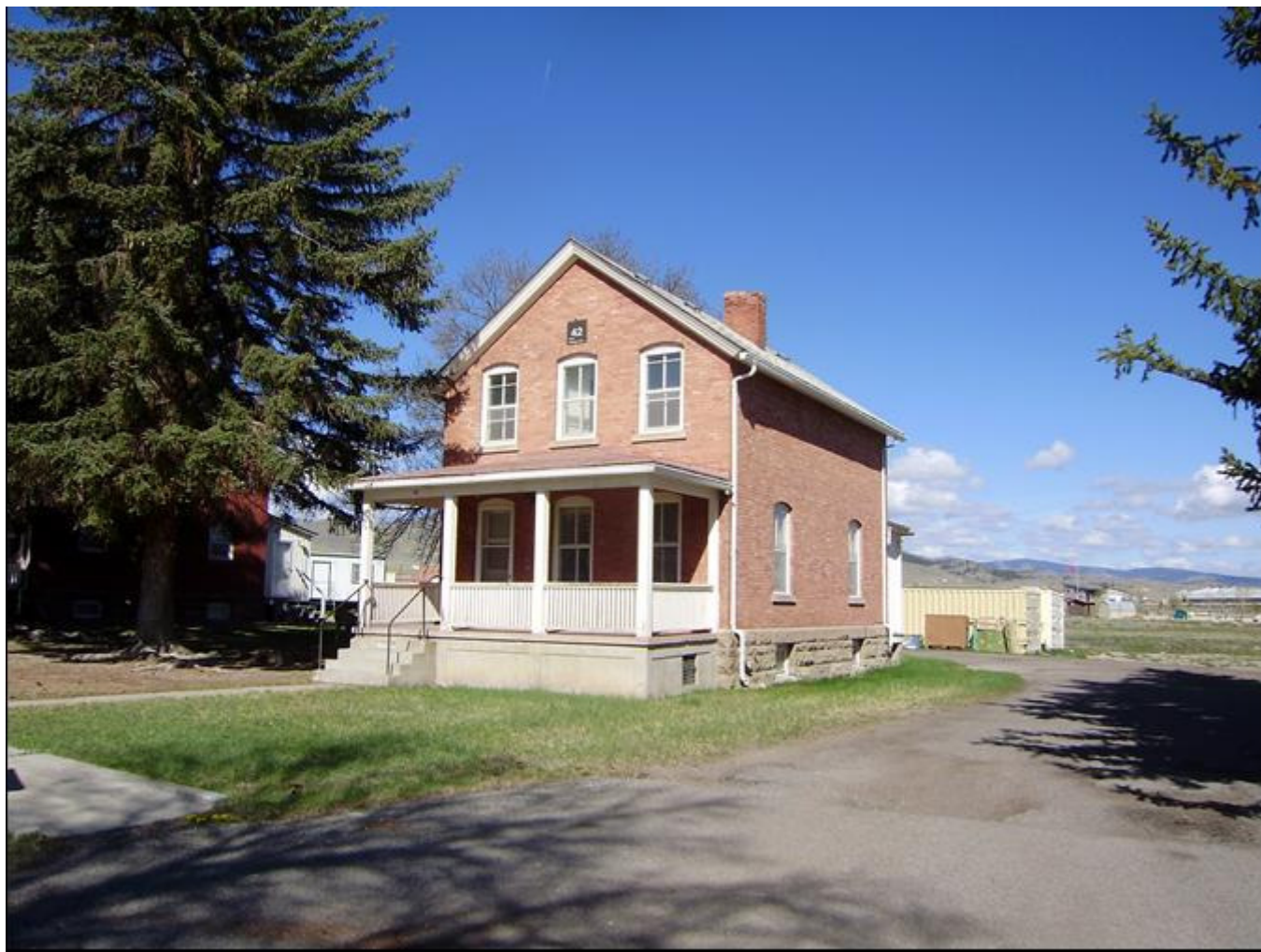
MT_LewisandClarkCounty_FortHarrisonVAHospitalHistoricDistrict_0036. Building 42. View to the WSW.
