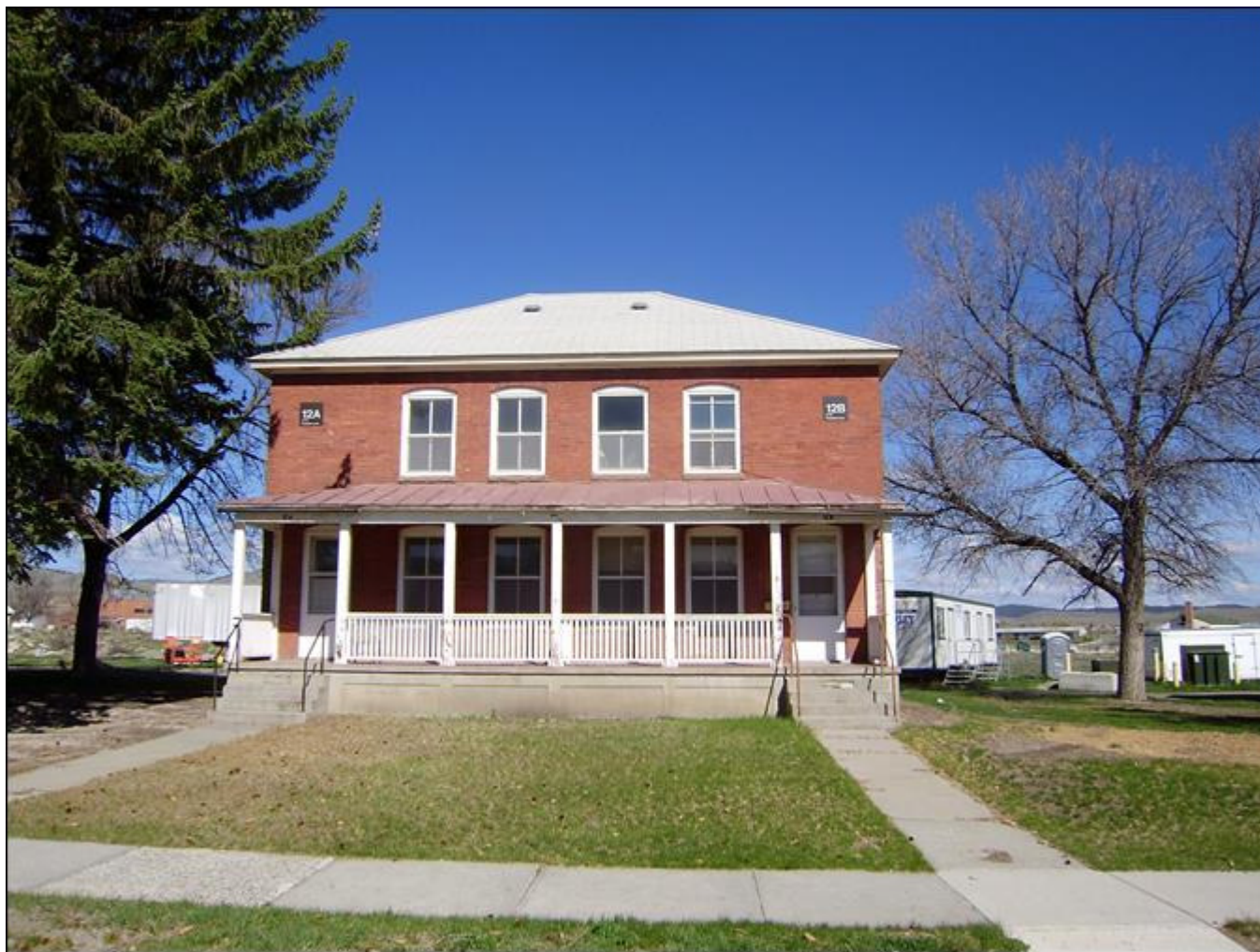
MT_LewisandClarkCounty_FortHarrisonVAHospitalHistoricDistrict_0014. Building 12. View to the west.
