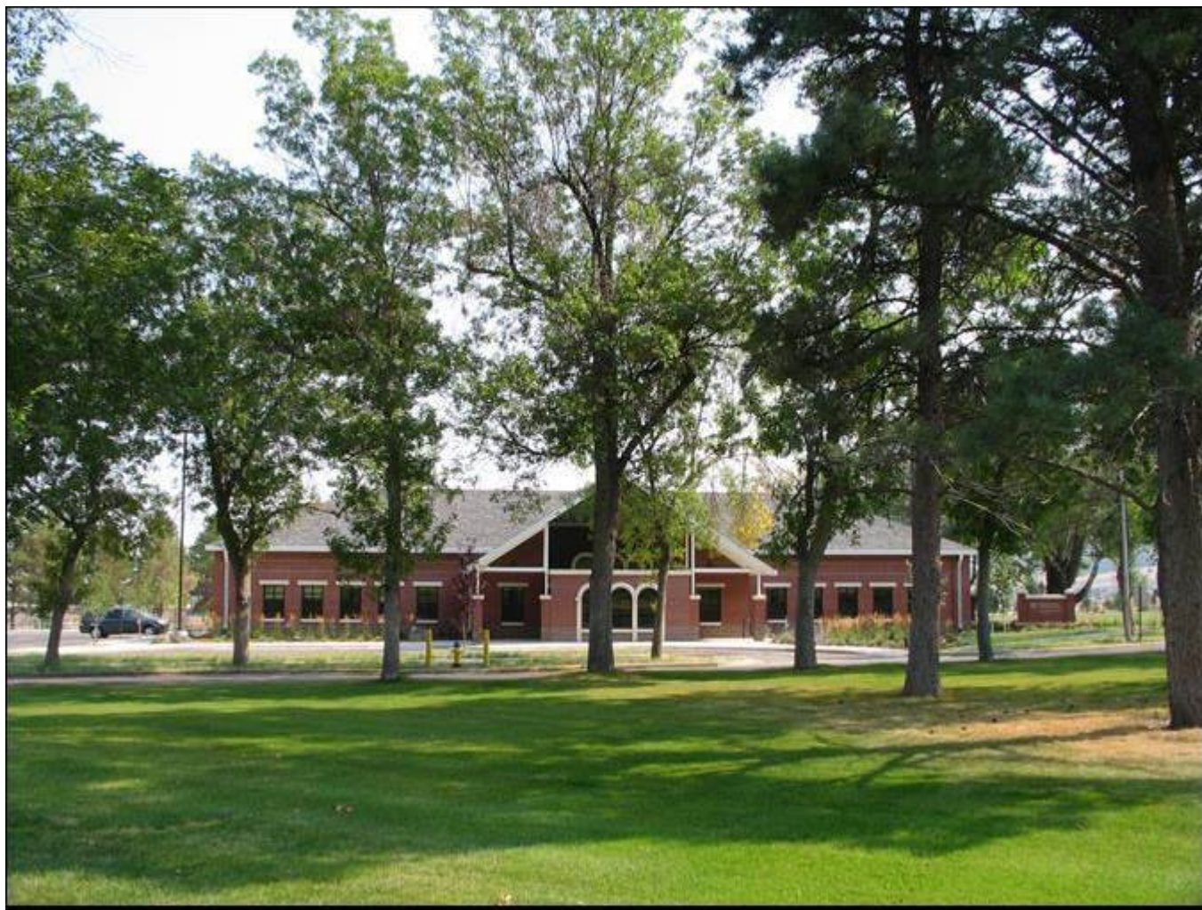
MT_LewisandClarkCounty_FortHarrisonVAHospitalHistoricDistrict_0076. Building 167. View to the east.
