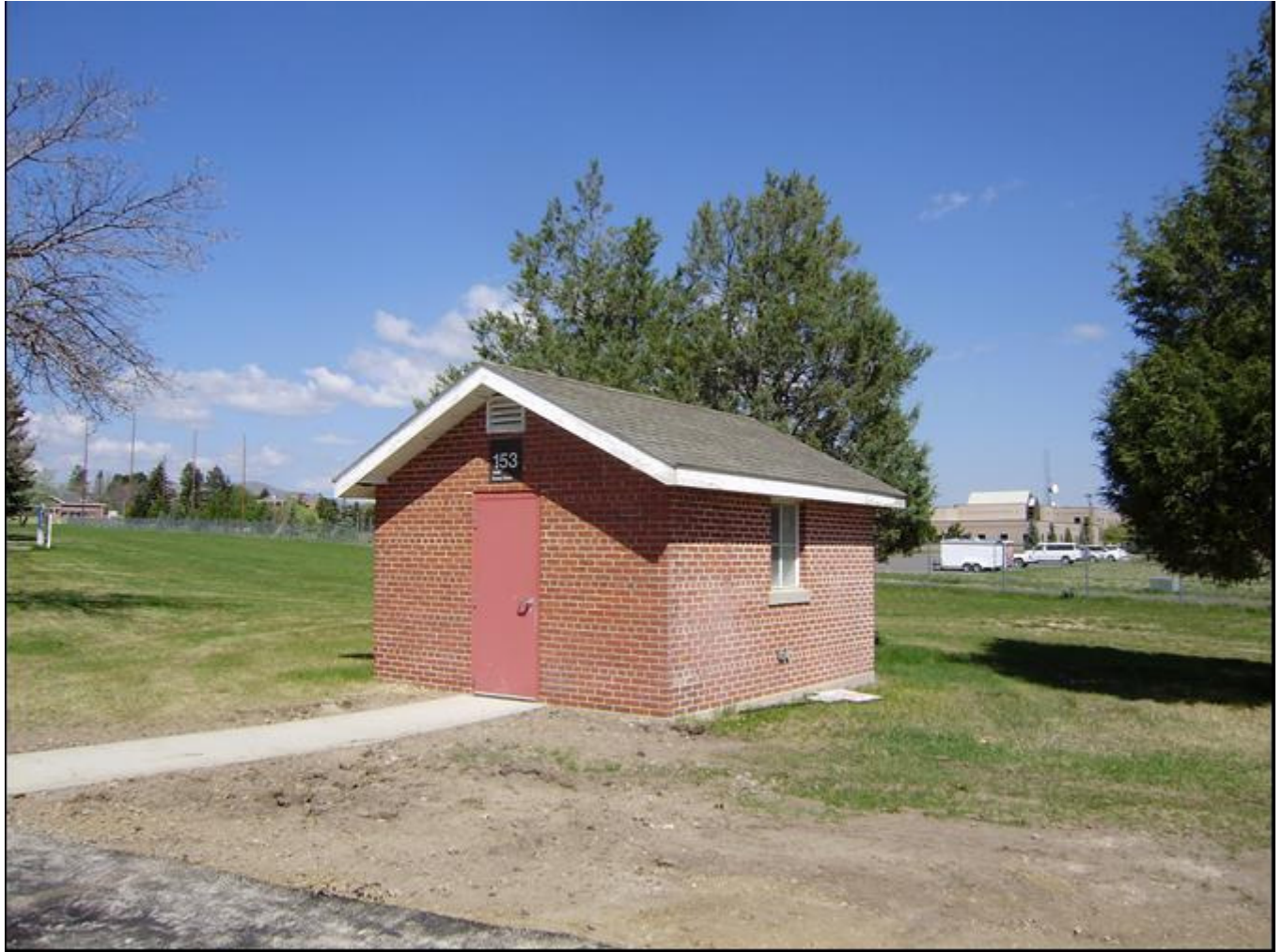
MT_LewisandClarkCounty_FortHarrisonVAHospitalHistoricDistrict_0066. Building 154. View to the northeast.
