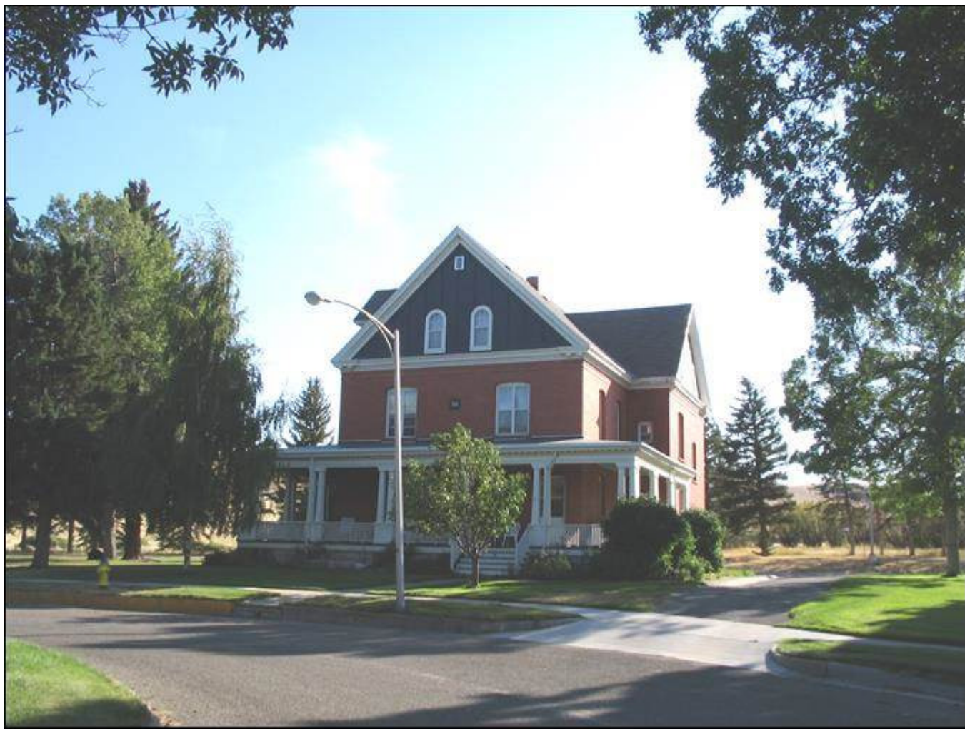
MT_LewisandClarkCounty_FortHarrisonVAHospitalHistoricDistrict_0030. Building 35. View to the south.
