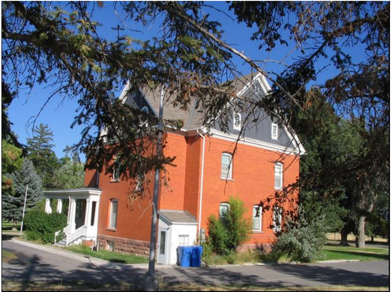
MT_LewisandClarkCounty_FortHarrisonVAHospitalHistoricDistrict_0032. Building 35. View to the northeast.
