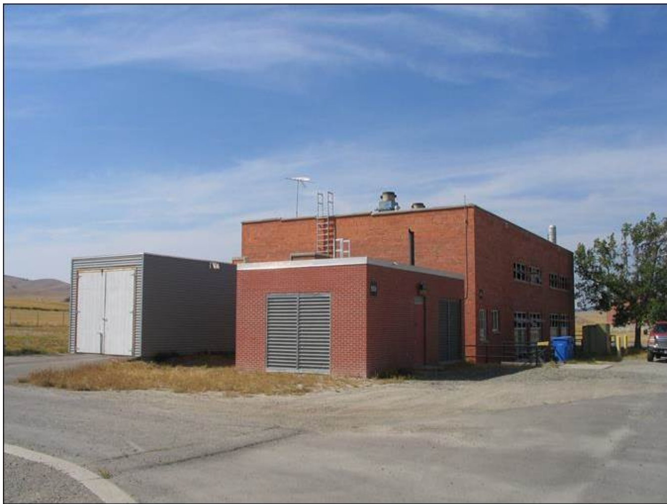
MT_LewisandClarkCounty_FortHarrisonVAHospitalHistoricDistrict_0073. Building 159. View to the WNW.
