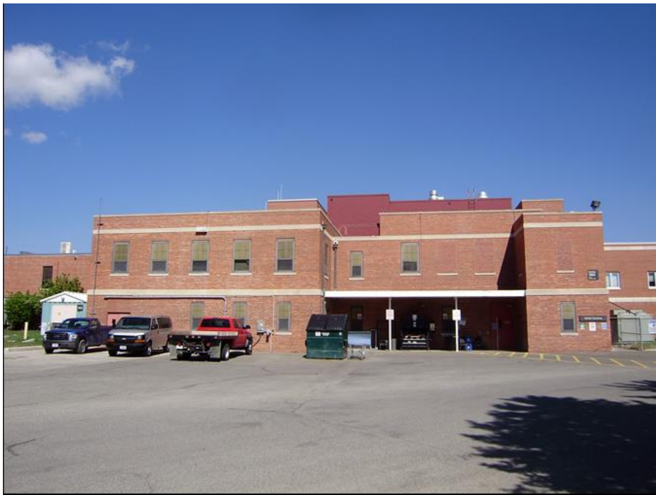
MT_LewisandClarkCounty_FortHarrisonVAHospitalHistoricDistrict_0062. Building 150. View to the west.
