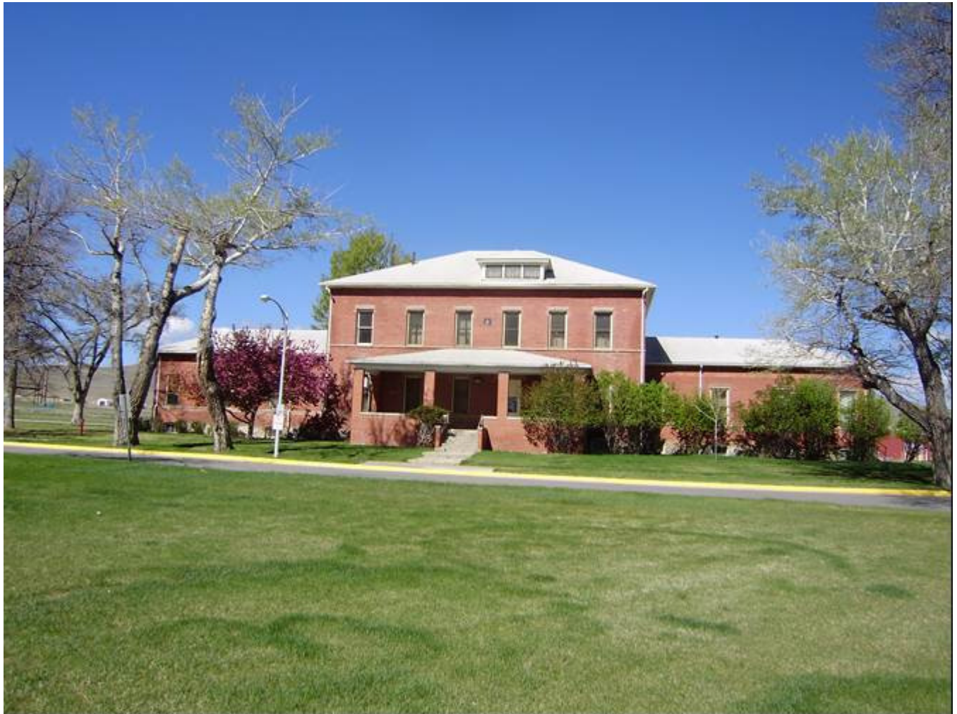
MT_LewisandClarkCounty_FortHarrisonVAHospitalHistoricDistrict_0002. Building 2. View to the west.
