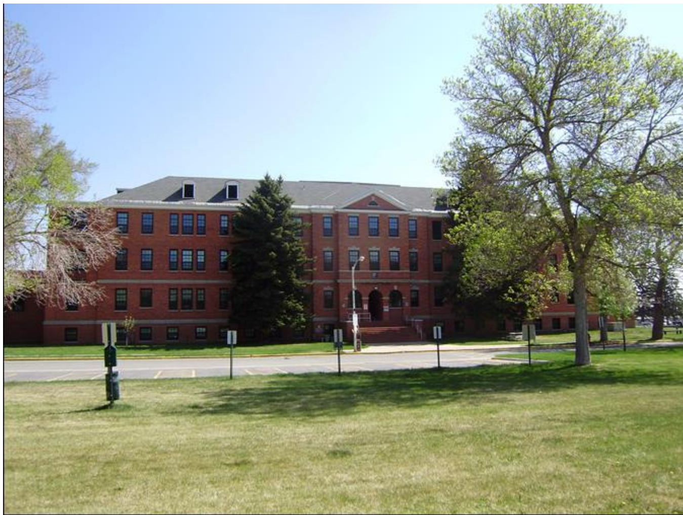
MT_LewisandClarkCounty_FortHarrisonVAHospitalHistoricDistrict_0051. Building 141. View to the north.
