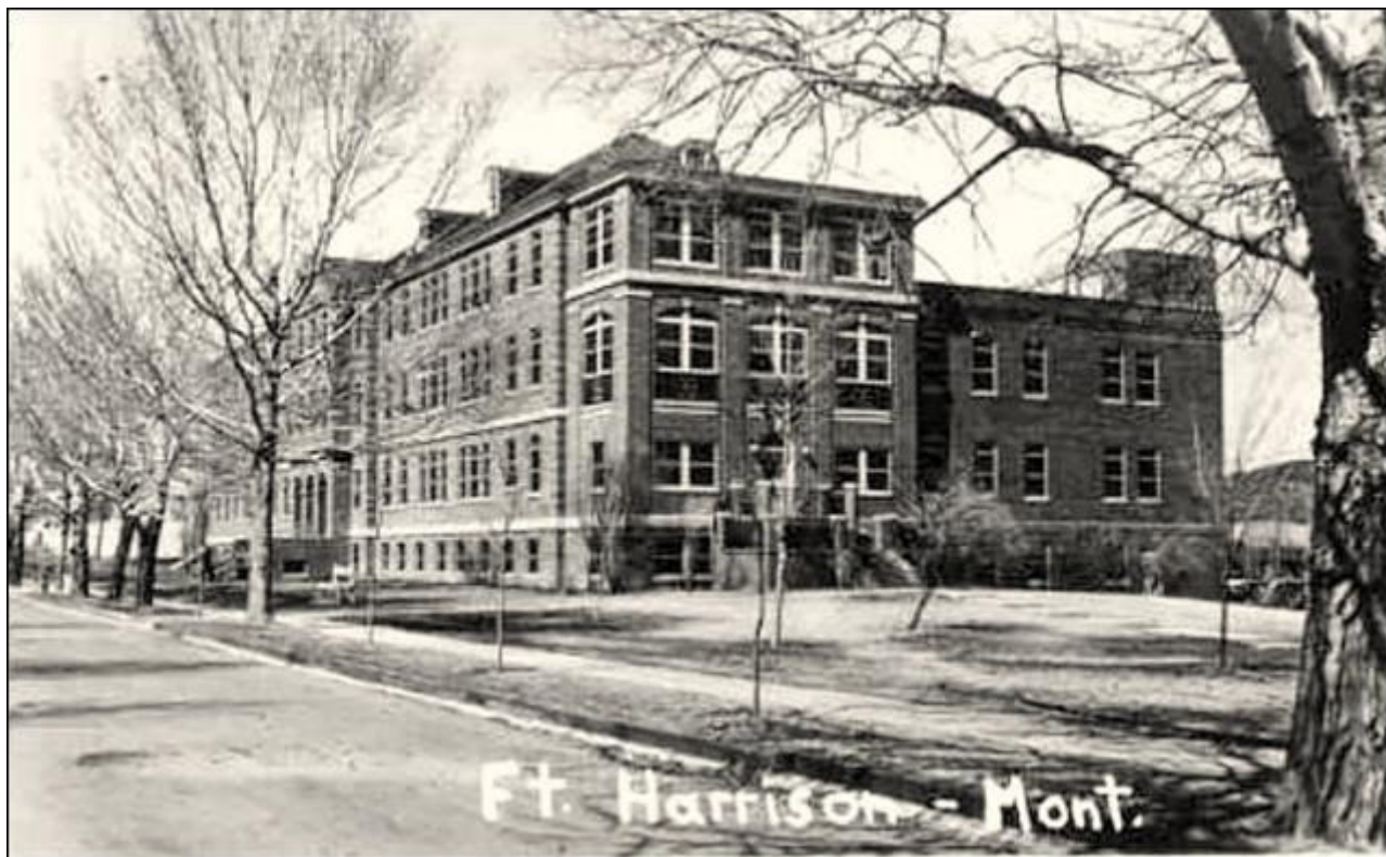
Photograph of 1932 hospital building (Building #141). View to the Northwest.
