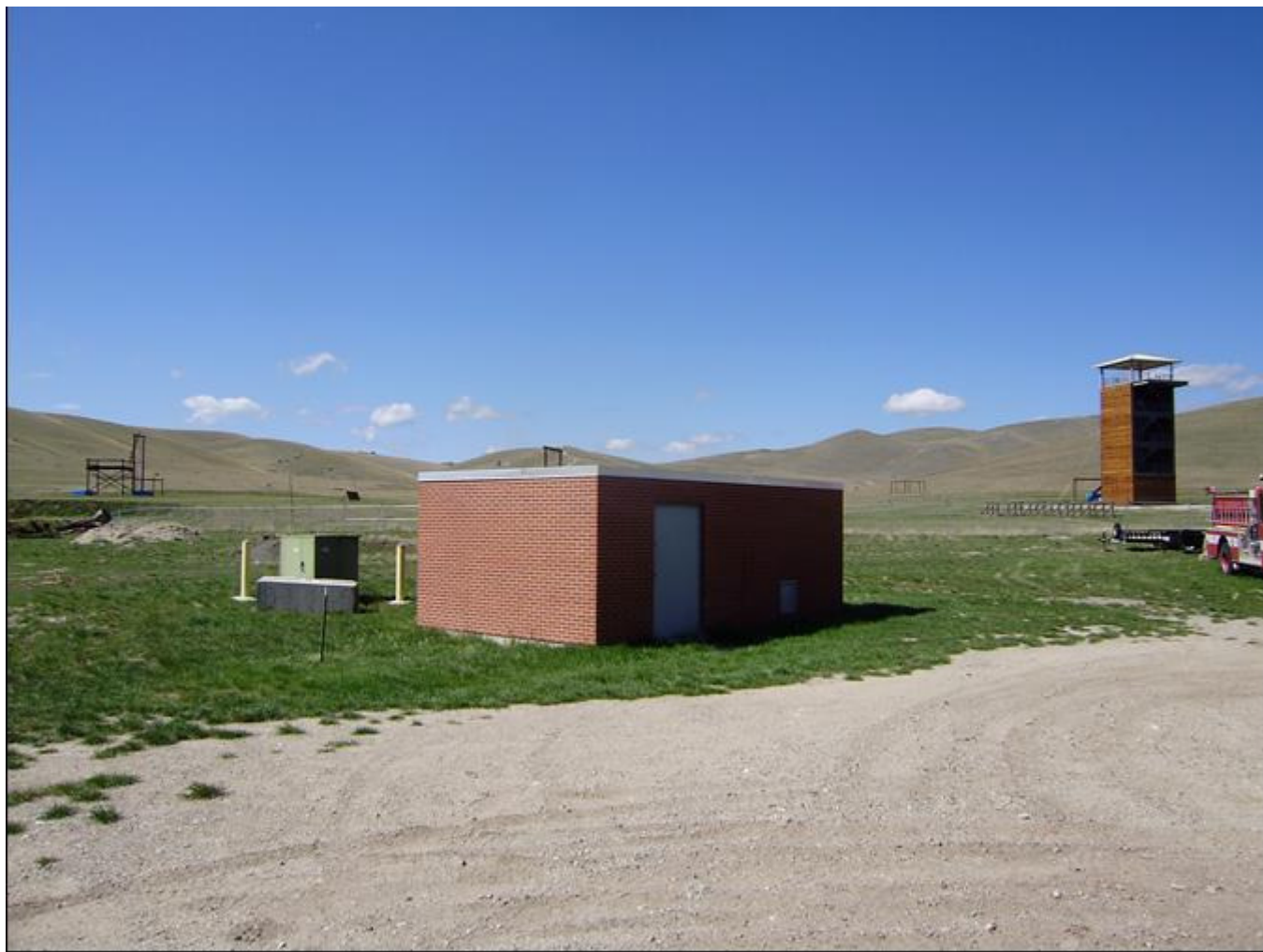
MT_LewisandClarkCounty_FortHarrisonVAHospitalHistoricDistrict_0074. Building 160. View to the northwest.
