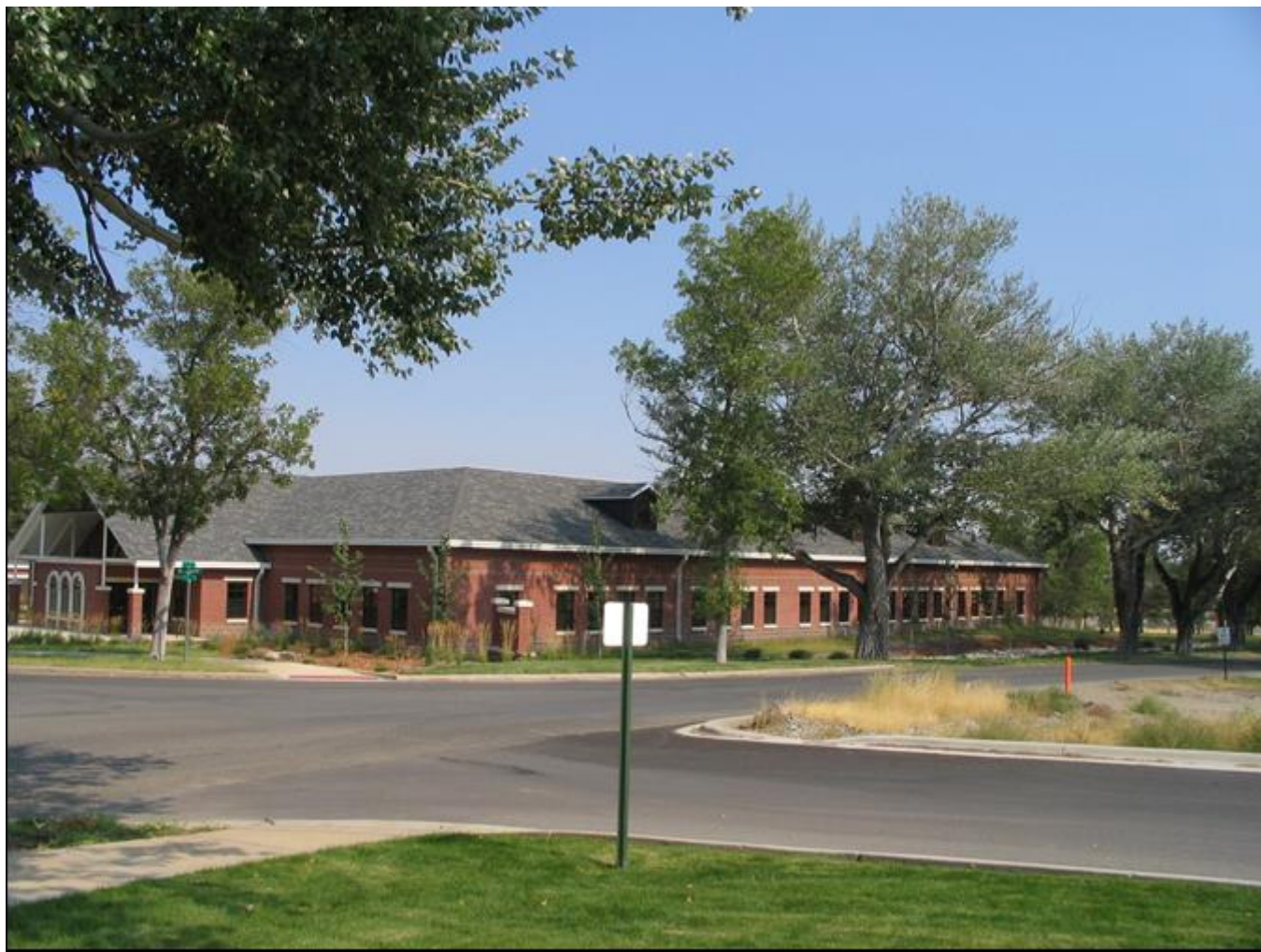
MT_LewisandClarkCounty_FortHarrisonVAHospitalHistoricDistrict_0075. Building 167. View to the northeast.
