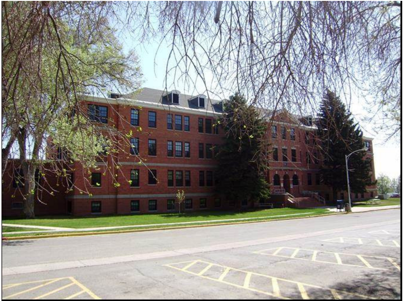
MT_LewisandClarkCounty_FortHarrisonVAHospitalHistoricDistrict_0050. Building 141. View to the northeast.
