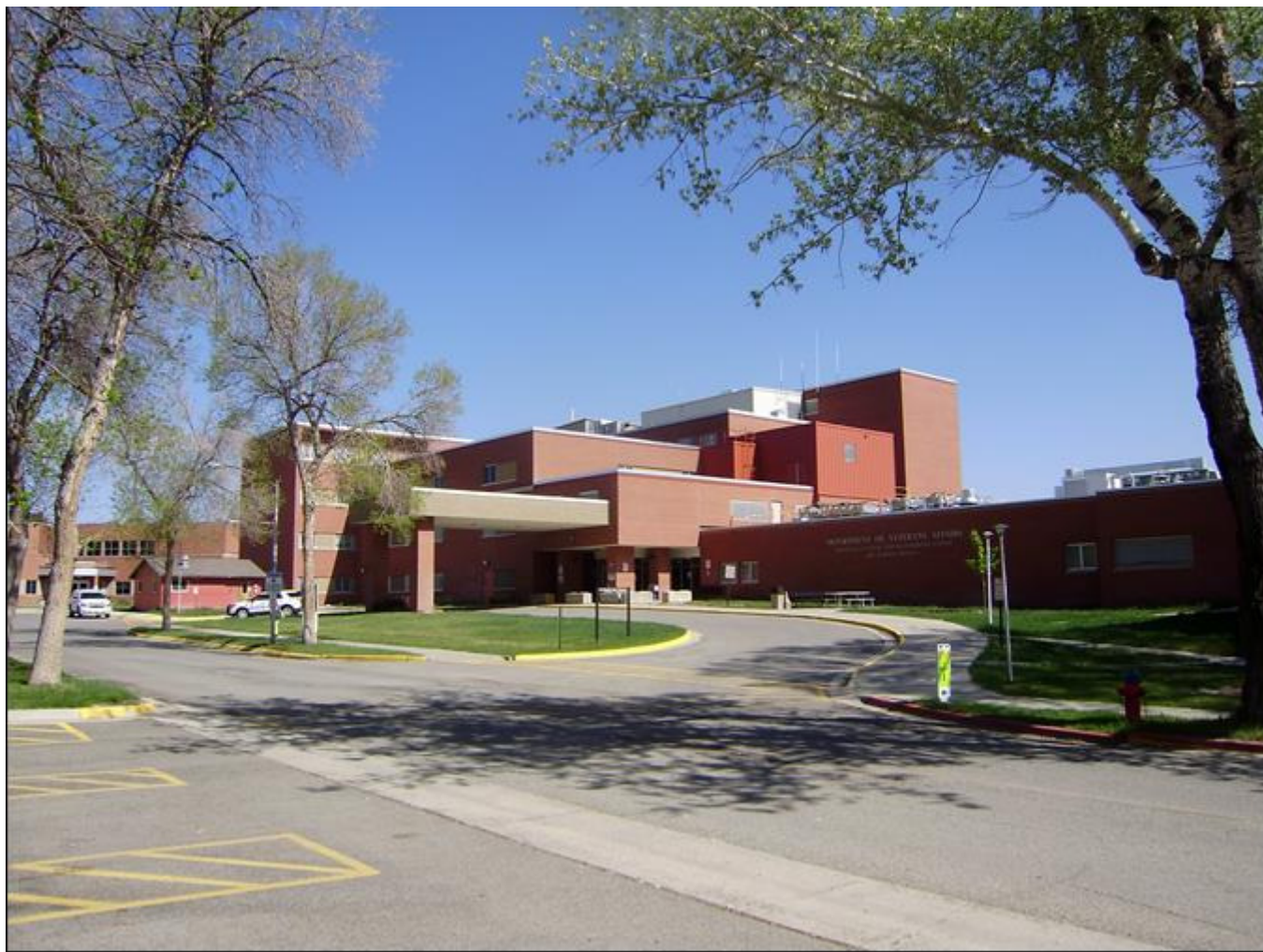
MT_LewisandClarkCounty_FortHarrisonVAHospitalHistoricDistrict_0067. Building 154. View to the north.
