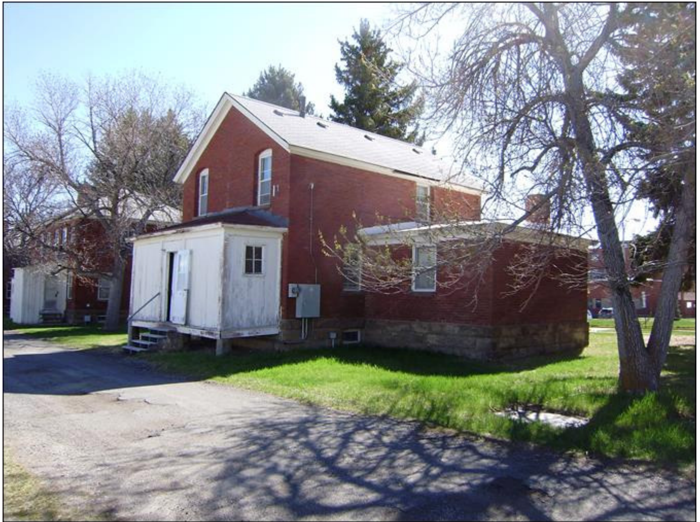
MT_LewisandClarkCounty_FortHarrisonVAHospitalHistoricDistrict_0019. Building 14. View to the northeast.
