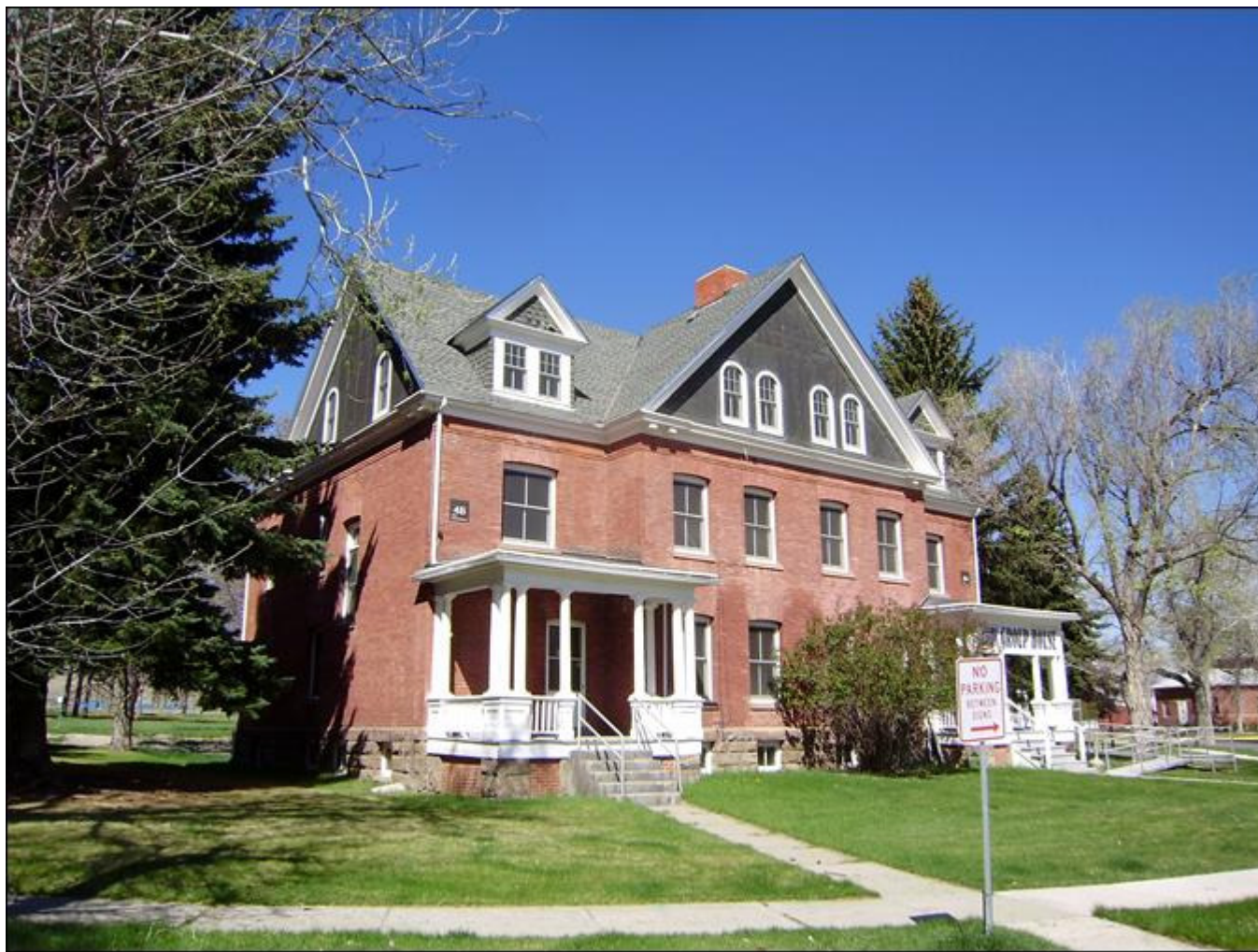
MT_LewisandClarkCounty_FortHarrisonVAHospitalHistoricDistrict_0008. Building 4. View to the NNW.
