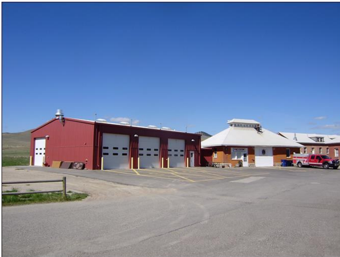
MT_LewisandClarkCounty_FortHarrisonVAHospitalHistoricDistrict_0020. Building 16. View to the NNW.
