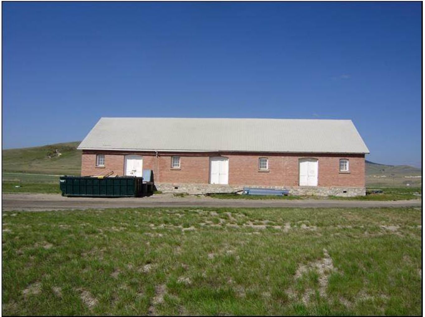
MT_LewisandClarkCounty_FortHarrisonVAHospitalHistoricDistrict_0028. Building 31. View to the west.
