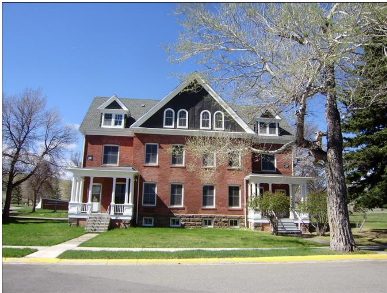
MT_LewisandClarkCounty_FortHarrisonVAHospitalHistoricDistrict_0005. Building 3. View to the west.
