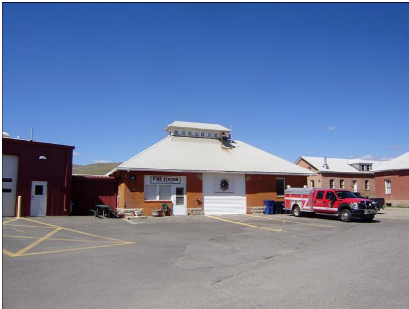
MT_LewisandClarkCounty_FortHarrisonVAHospitalHistoricDistrict_0021. Building 16. View to the WNW.
