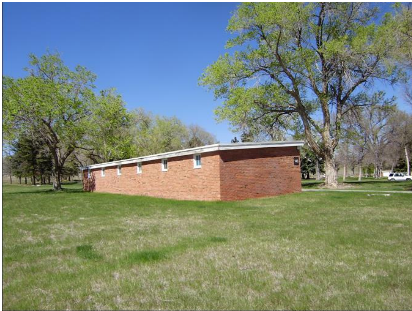
MT_LewisandClarkCounty_FortHarrisonVAHospitalHistoricDistrict_0061. Building 146. View to the northwest.
