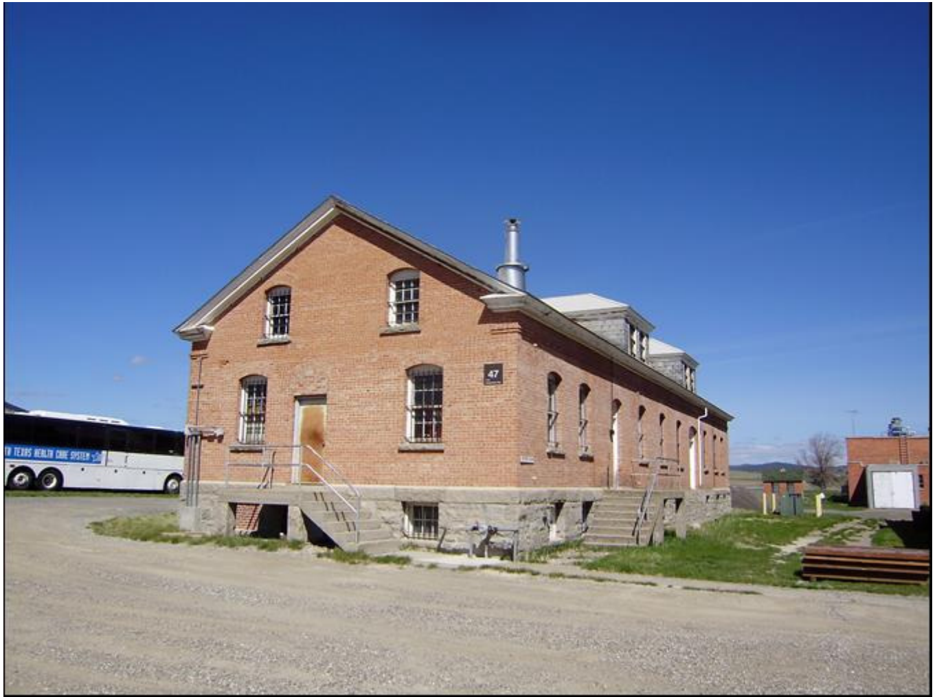
MT_LewisandClarkCounty_FortHarrisonVAHospitalHistoricDistrict_0041. Building 47. View to the NNW.
