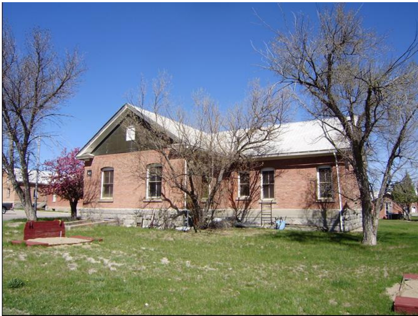
MT_LewisandClarkCounty_FortHarrisonVAHospitalHistoricDistrict_0039. Building 43. View to the northwest.
