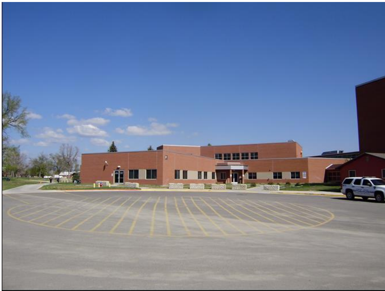
MT_LewisandClarkCounty_FortHarrisonVAHospitalHistoricDistrict_0079. Building 169. View to the northwest.
