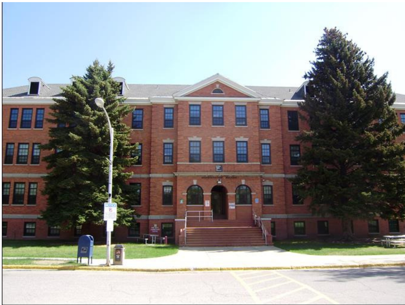
MT_LewisandClarkCounty_FortHarrisonVAHospitalHistoricDistrict_0052. Building 141. View to the north.
