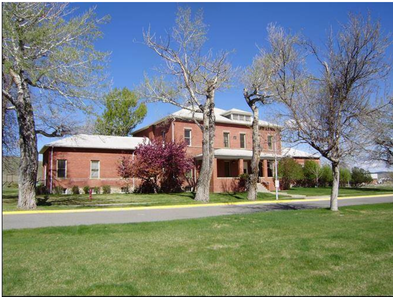
MT_LewisandClarkCounty_FortHarrisonVAHospitalHistoricDistrict_0003. Building 2. View to the NNW.
