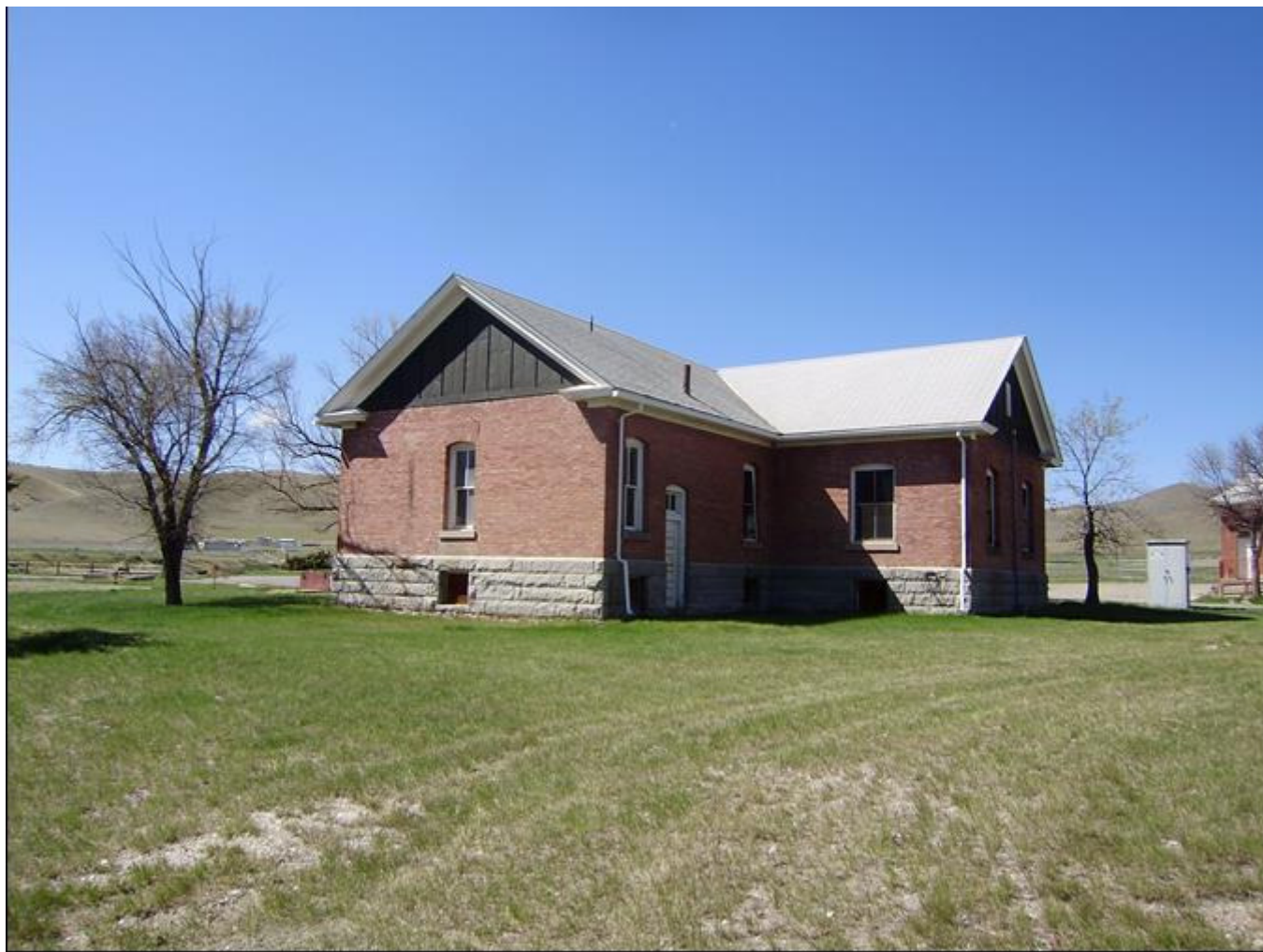
MT_LewisandClarkCounty_FortHarrisonVAHospitalHistoricDistrict_0040. Building 43. View to the WSW.
