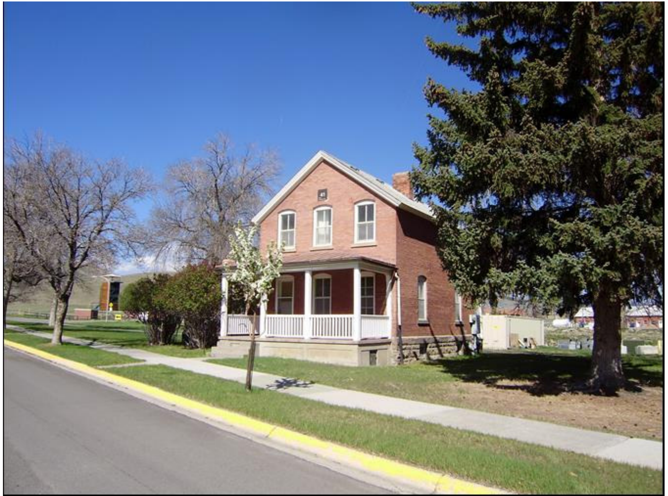
MT_LewisandClarkCounty_FortHarrisonVAHospitalHistoricDistrict_0033. Building 41. View to the southwest.
