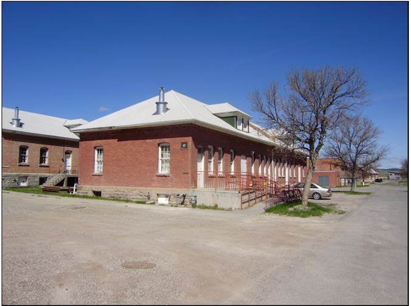
MT_LewisandClarkCounty_FortHarrisonVAHospitalHistoricDistrict_0023. Building 17. View to the NNW.
