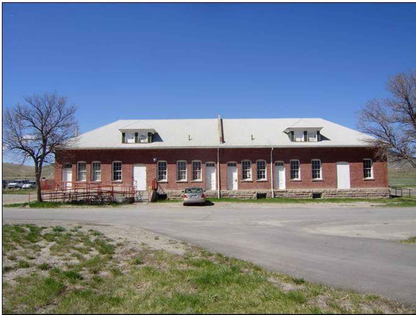
MT_LewisandClarkCounty_FortHarrisonVAHospitalHistoricDistrict_0024. Building 17. View to the west.
