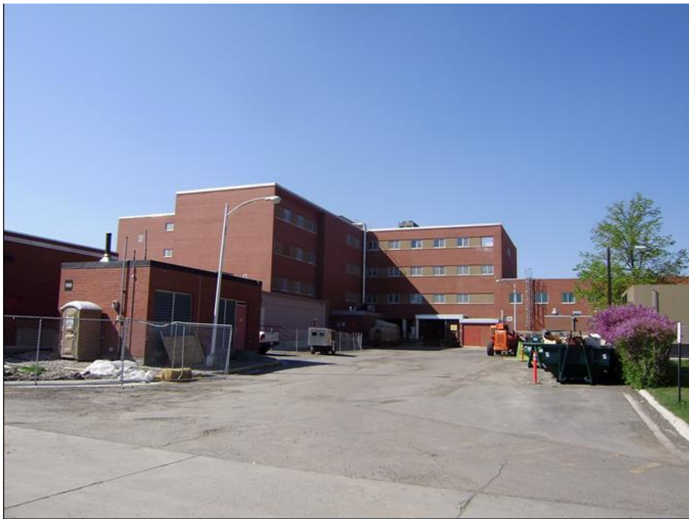
MT_LewisandClarkCounty_FortHarrisonVAHospitalHistoricDistrict_0069. Building 154. View to the south.
