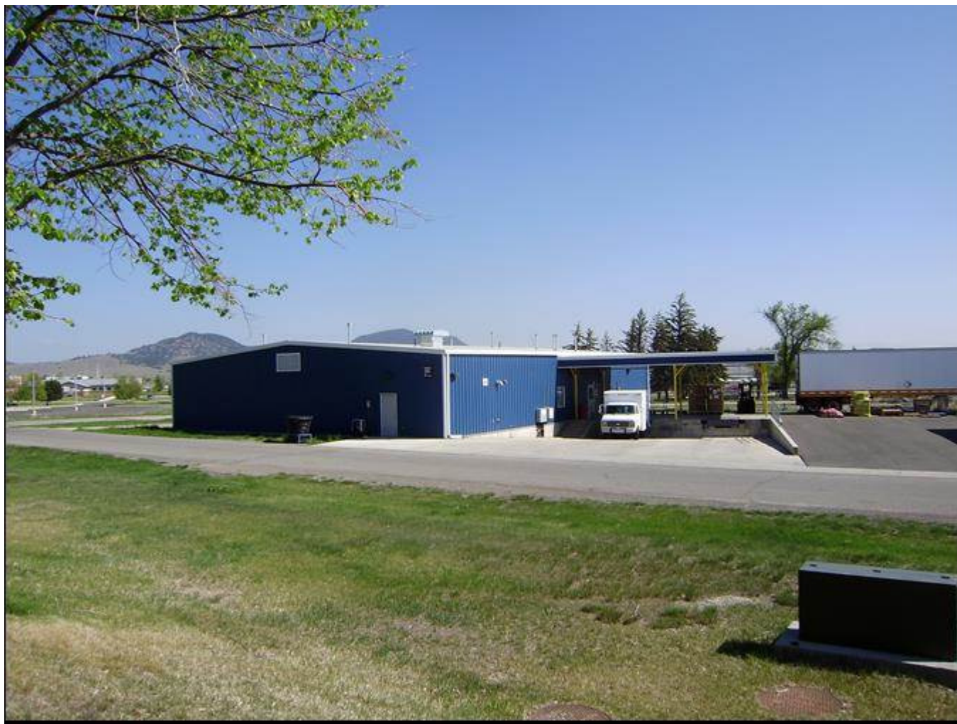
MT_LewisandClarkCounty_FortHarrisonVAHospitalHistoricDistrict_0080. Building 170. View to the NNW.
