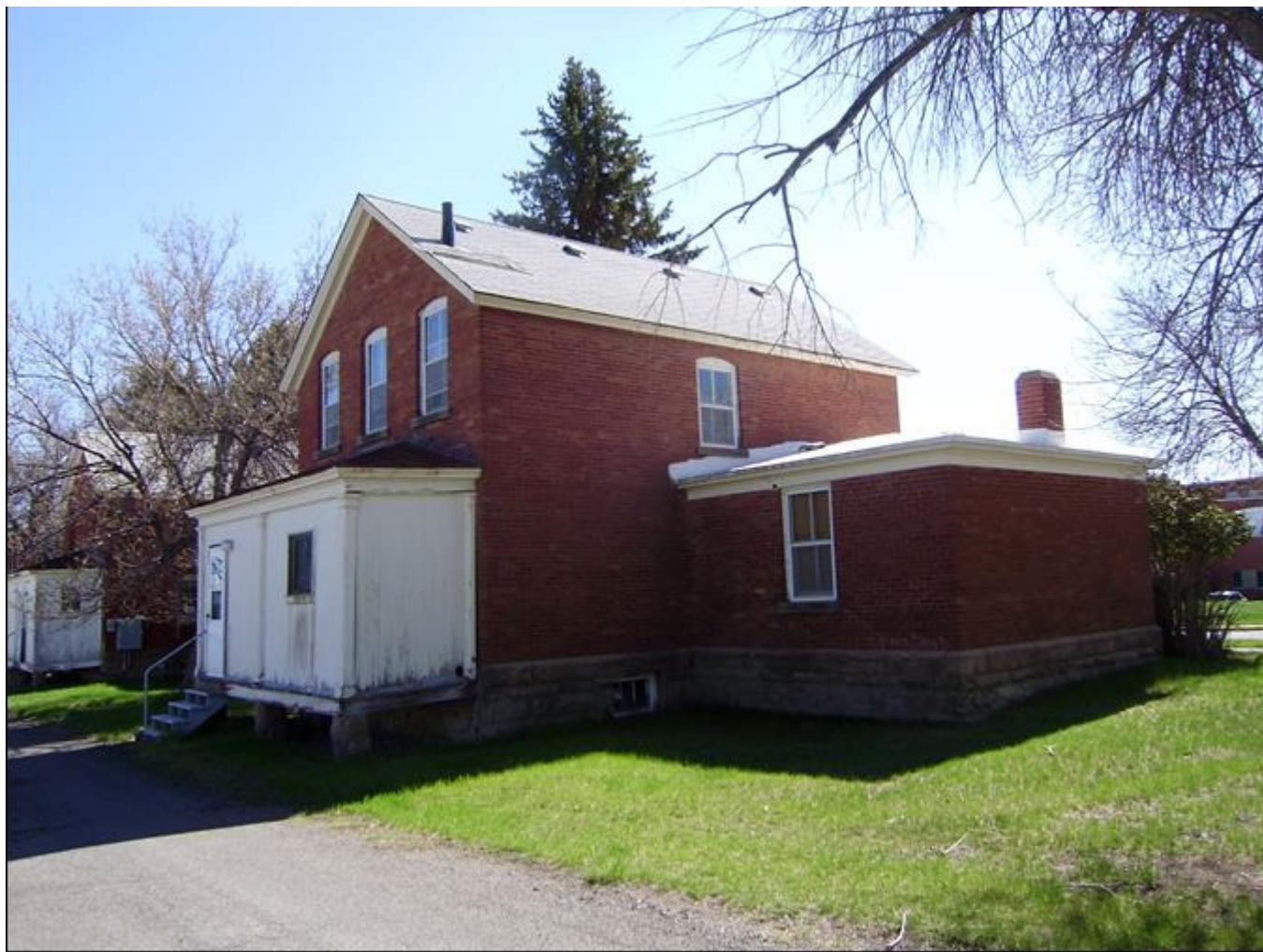
MT_LewisandClarkCounty_FortHarrisonVAHospitalHistoricDistrict_0034. Building 41. View to the northeast.
