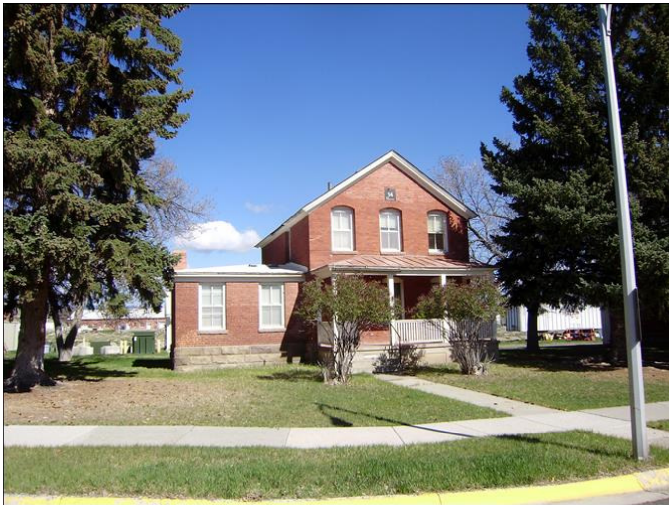
MT_LewisandClarkCounty_FortHarrisonVAHospitalHistoricDistrict_0018. Building 14. View to the west.
