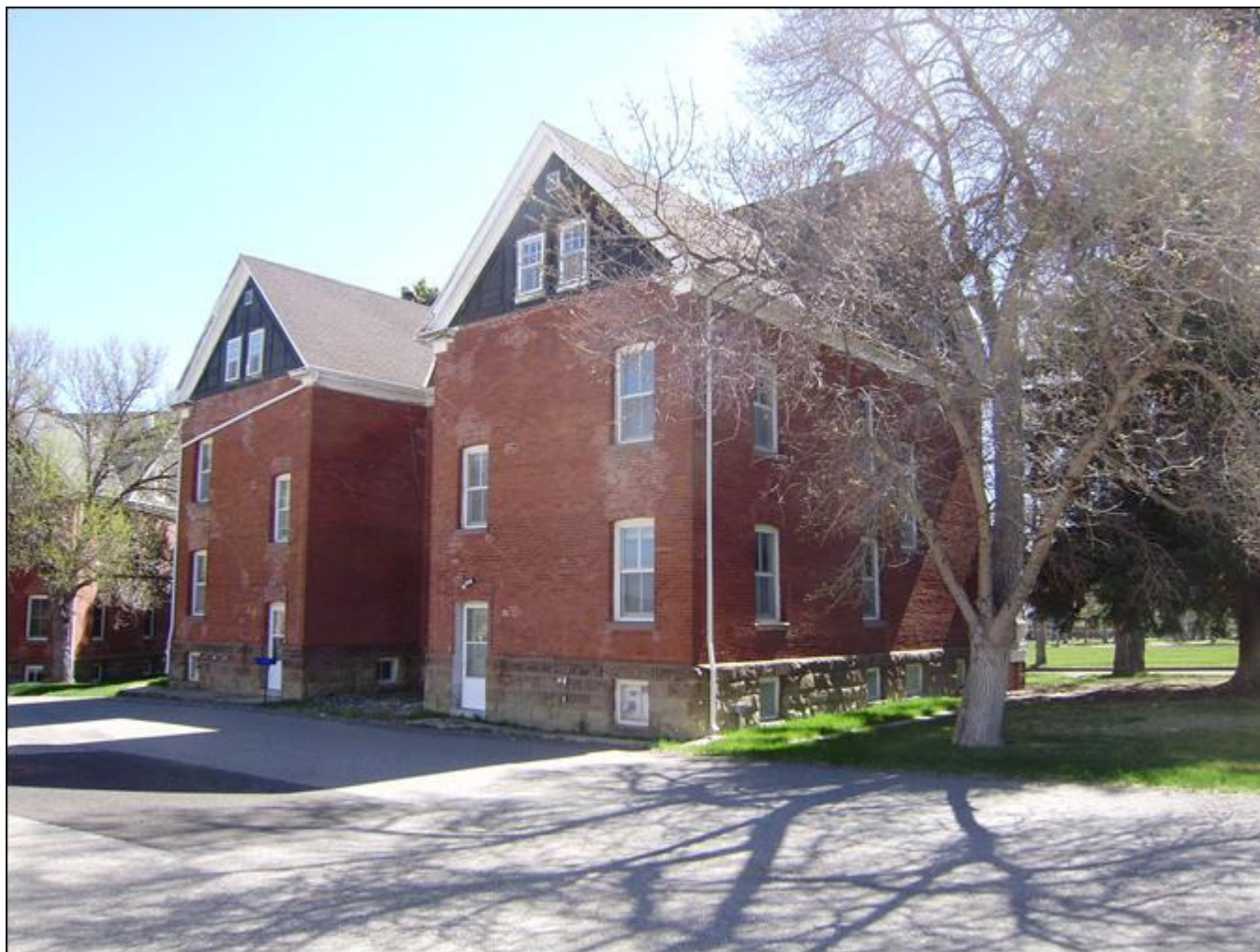
MT_LewisandClarkCounty_FortHarrisonVAHospitalHistoricDistrict_0011. Building 5. View to the northeast.
