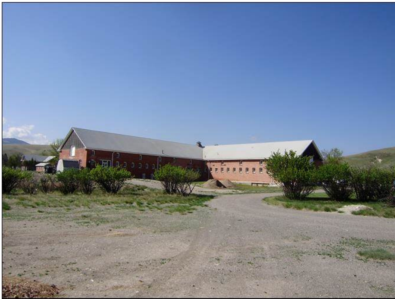
MT_LewisandClarkCounty_FortHarrisonVAHospitalHistoricDistrict_0027. Building 20. View to the southwest.
