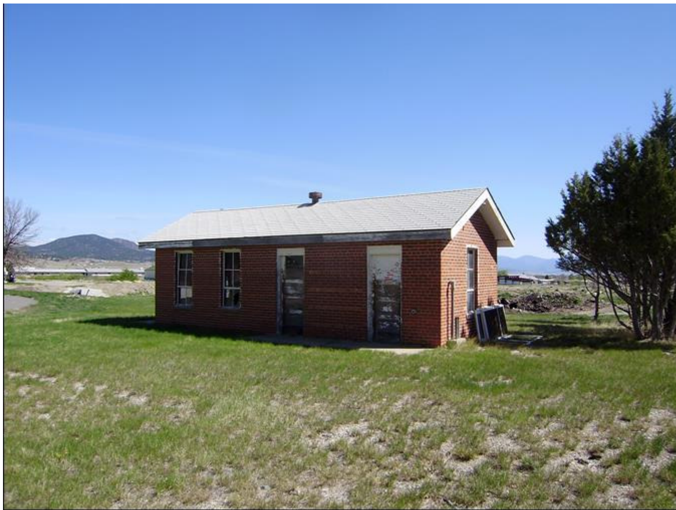
MT_LewisandClarkCounty_FortHarrisonVAHospitalHistoricDistrict_0048. Building 54. View to the northeast.
