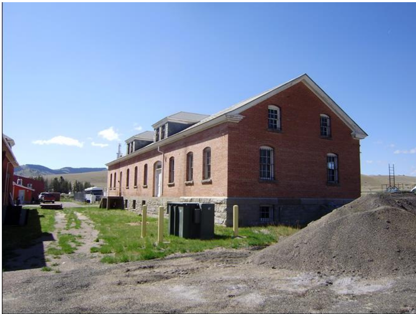
MT_LewisandClarkCounty_FortHarrisonVAHospitalHistoricDistrict_0042. Building 47. View to the southwest.
