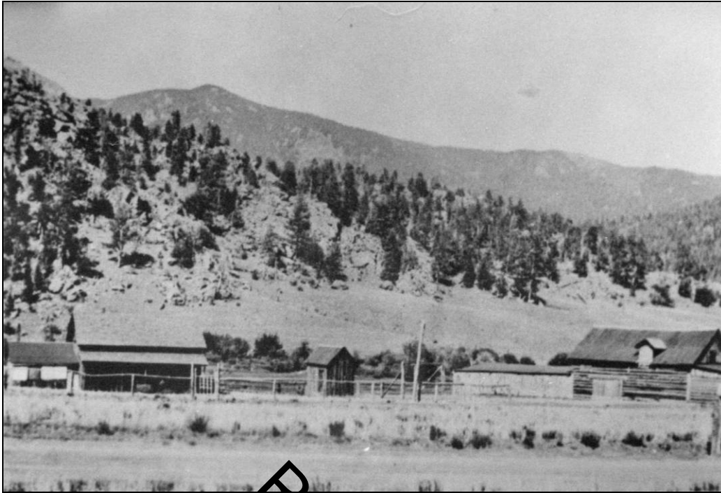
Figure 11. This pre-1940s view of the Derby/Terhune/Eavenson Ranch shows the main house to the left and the 1880s barn erected by William A. Derby to the right. Courtesy of Park County Local History Archives, photographic collection.
