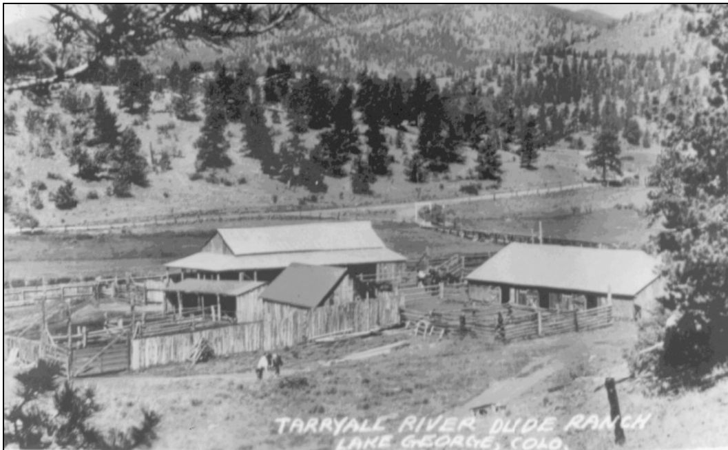
Figure 12. This ca. 1940s postcard for the Tarryall River Dude Ranch (view west) shows the main barn and other animal support buildings near Tarryall Creek. Courtesy of Park County Local History Archives, photographic collection, image 1359, Margaret Howell McArthur collection.
