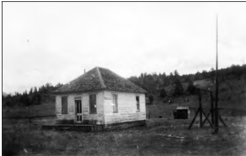
Figure 3. In this 1947 photograph Hayman school is shown in its second location, along Tarryall Road, after its days as an educational facility ended. Note the swing set to the right and a probable outhouse to the rear. Courtesy of Western History and Genealogy Department, Denver Public Library, Muriel Sibell Wolle photograph, image number X-5819, 1947.
