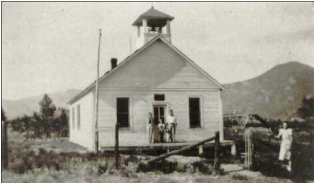
Figure 13. Listed in the National Register of Historic Places, the 1921 Tarryall School is representative of the one-room schools once found in rural areas throughout Colorado. Courtesy of Park County Local History Archives, image 300, provided by Sydney Johnson, 1941.
