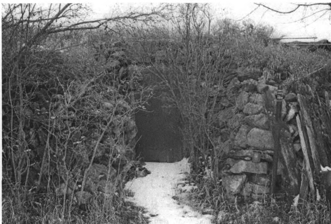
NR Photo #0010 – Root Cellar, view from east.
