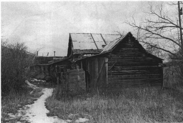
NR Photo #0006 – Main House, view from east.
