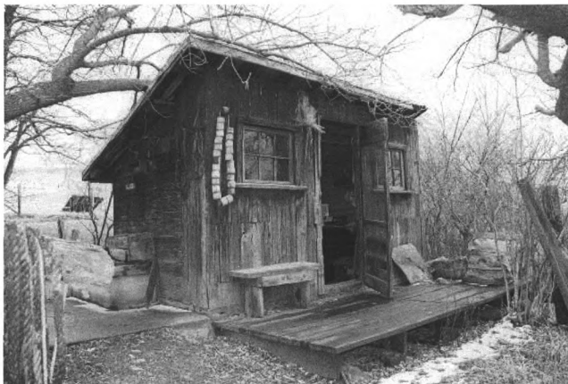
NR Photo #0014 – Milk House, view from northeast.
