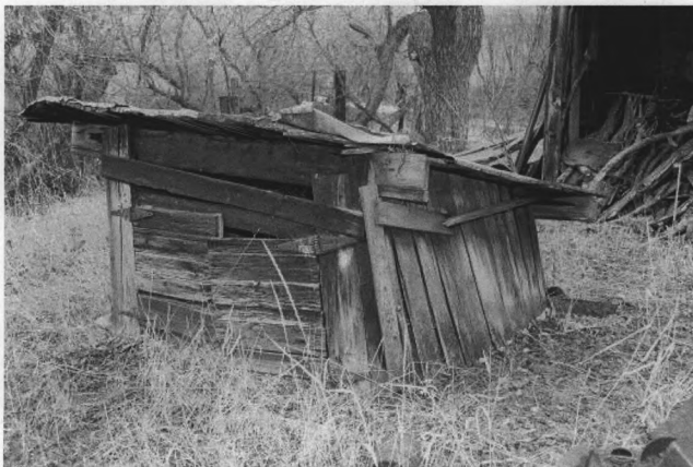
NR Photo #0013 – Domestic Hog Shed, view from southeast.
