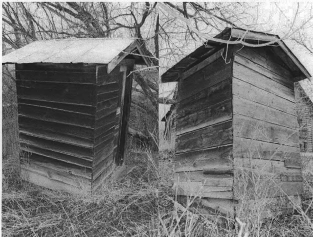
NR Photos #0008 and 0009 – Outhouse, view from southwest (0008) and northeast (0009).
