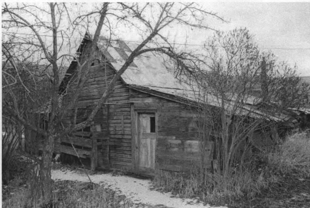
NR Photo #0007 – Main House, view from northwest.
