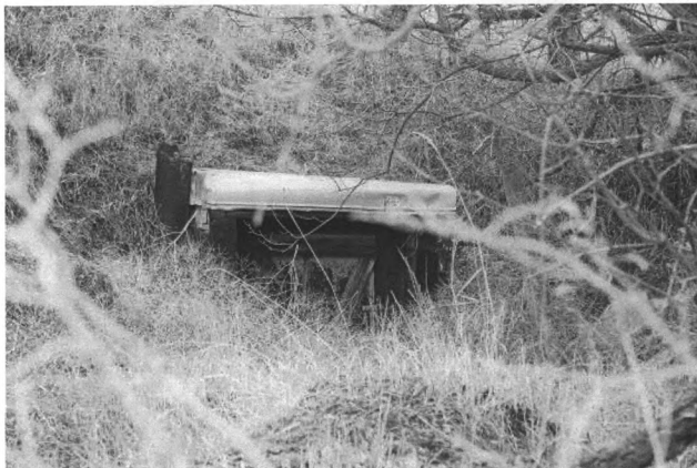
NR Photo #0028 – Mine adit portal, view from west.
