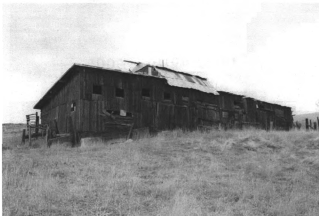
NR Photo #0024 – Barn – view from southwest.
