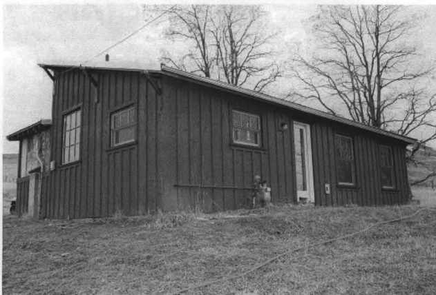
NR Photo #0017 – 1946 Residence/converted chicken coop, view from northeast.
