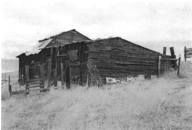
NR Photo #0025 – Barn, view from southeast.
