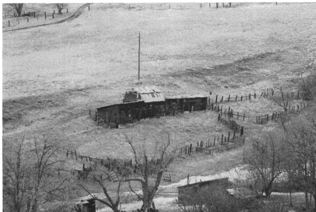
NR Photo #0023 - Barn and Corral System, view from southwest.
