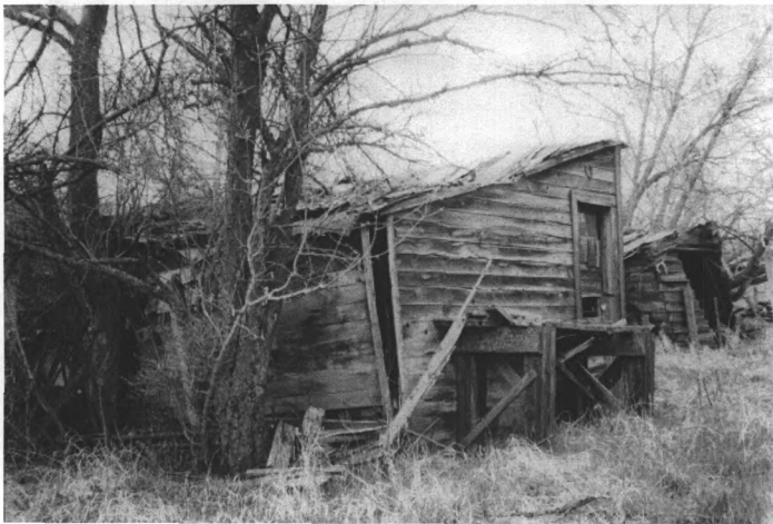
NR Photo #0040 – Moon Claim Cabin 2001, prior to rehabilitation, view from northwest.
