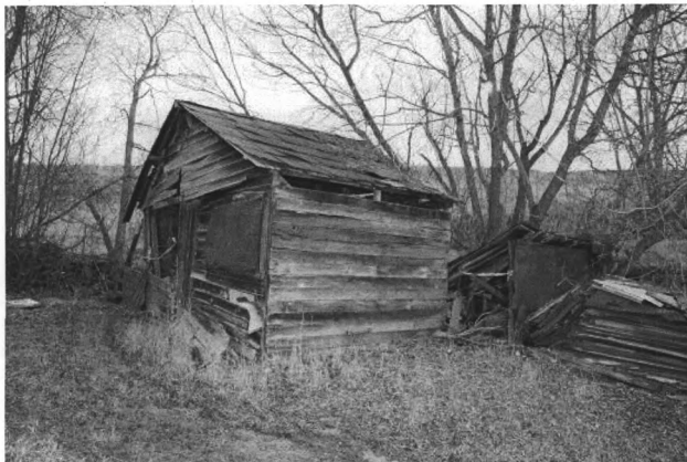
NR Photo #0029 – Winch Shed, view from south.
