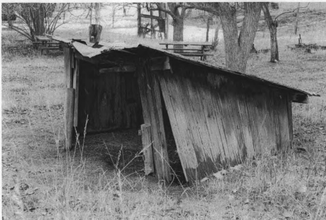
NR Photo #0020 – Orchard Hog shed, view from southeast.
