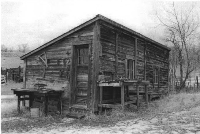
NR Photo #0004 – Moon Claim Cabin, view from southwest.
