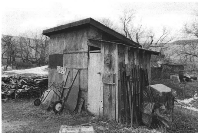
NR Photo #0027 – “Tin Shed” with attached outhouse, view from north.
