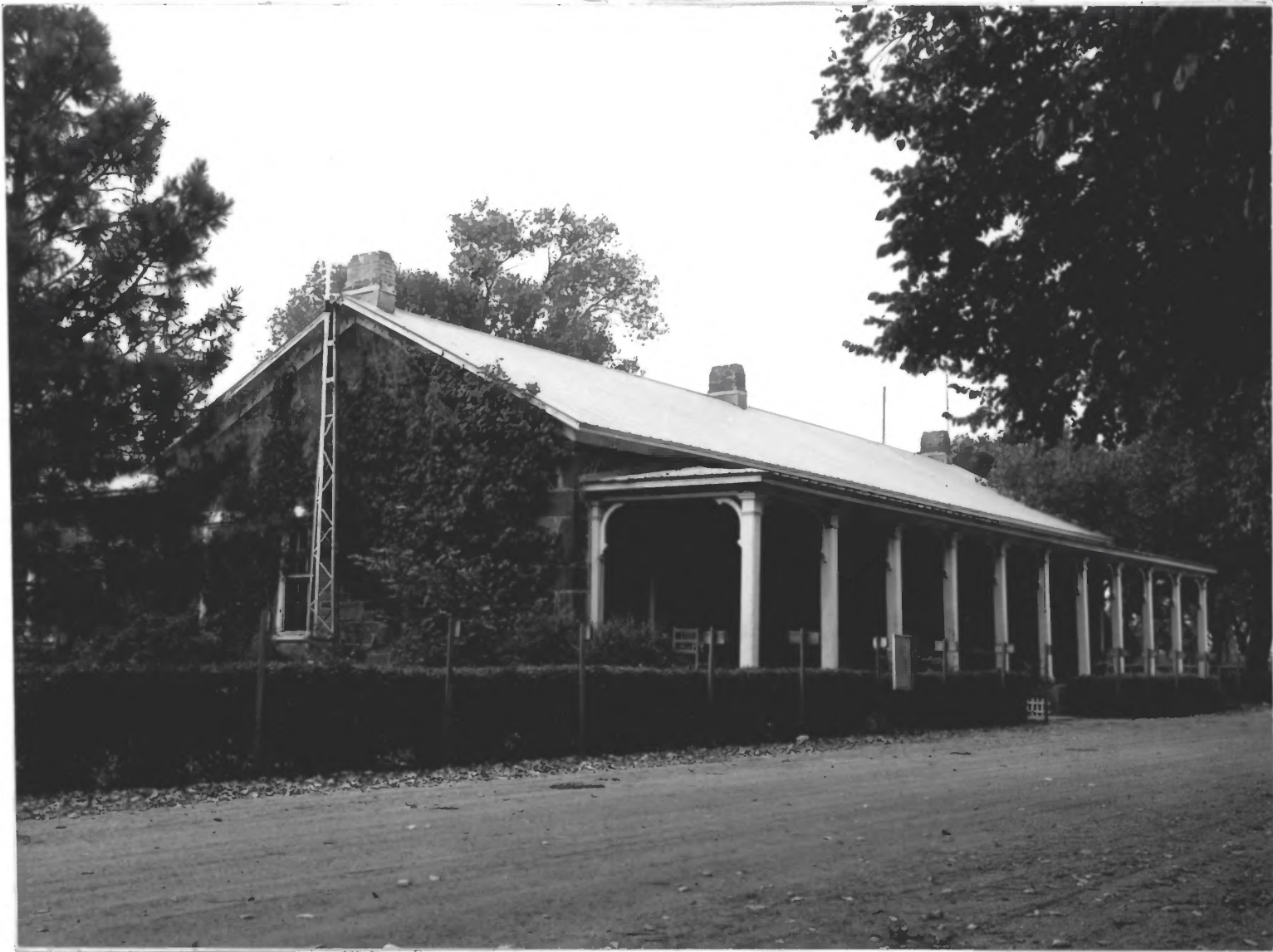
OFFICERS' QUARTERS FORT LARNED. This structure now serves as a museum
