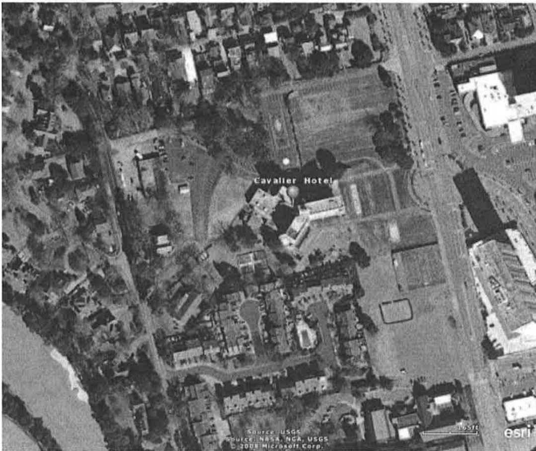
Cavalier Hotel - Aerial View
