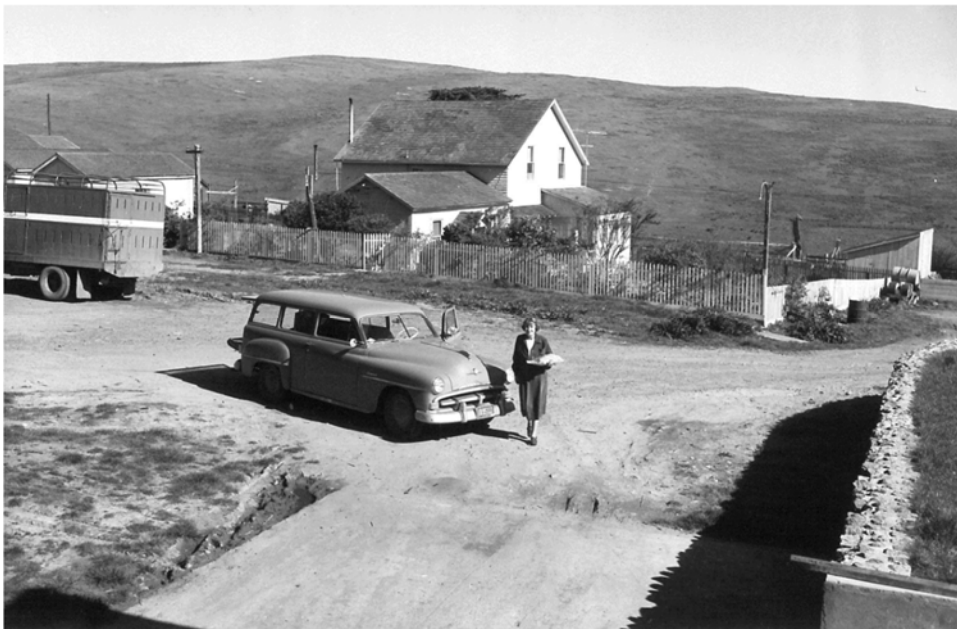
Photograph, dated ca. 1951, showing vegetation growing in the yard of the original main residence, surrounded by a picket fence. Note the rock wall and lawn of the 1951 main residence in the lower right hand corner (Williams Woodbridge Collection, Point Reyes National Seashore Archives, Catalog No. 55910)
