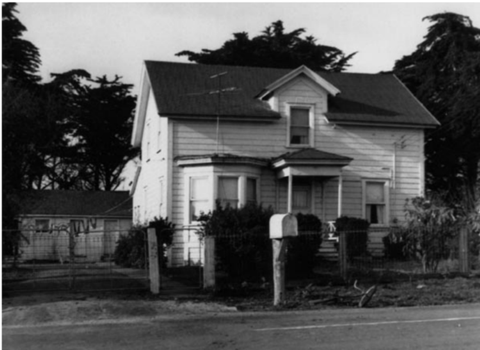
Photograph of the main house used in the 1963 NPS Appraisal of C Ranch. The historic windbreak is visible behind the house. (Point Reyes National Seashore Archives, Catalog No. 54490)
