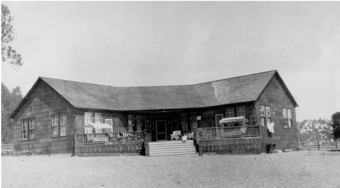
Rapp House after it was constructed in 1923 (Point Reyes National Seashore Archives, Catalog No. 52010)
