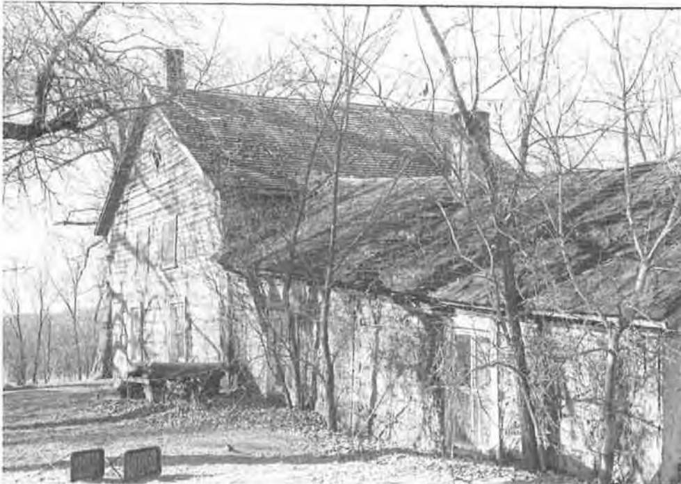
Fig. 16b: 1983 Hillier documentary photo showing condition of before collapse of attached log shed. (digitized from the collections of the Pembina County Historical Society Museum.)
