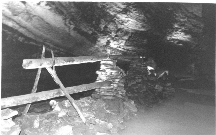
5. pipes near Methodist church, salt petre Mining works Mammoth Cave National Park, Kentucky (H52B)
