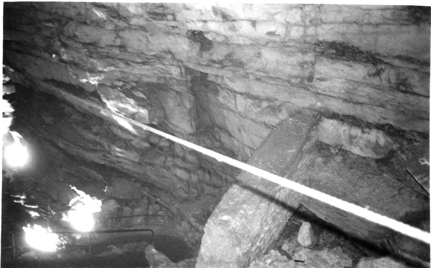
17. Cable at Aerobridge Canyon (IC-04) Mammoth Cave National Park, Kentucky
