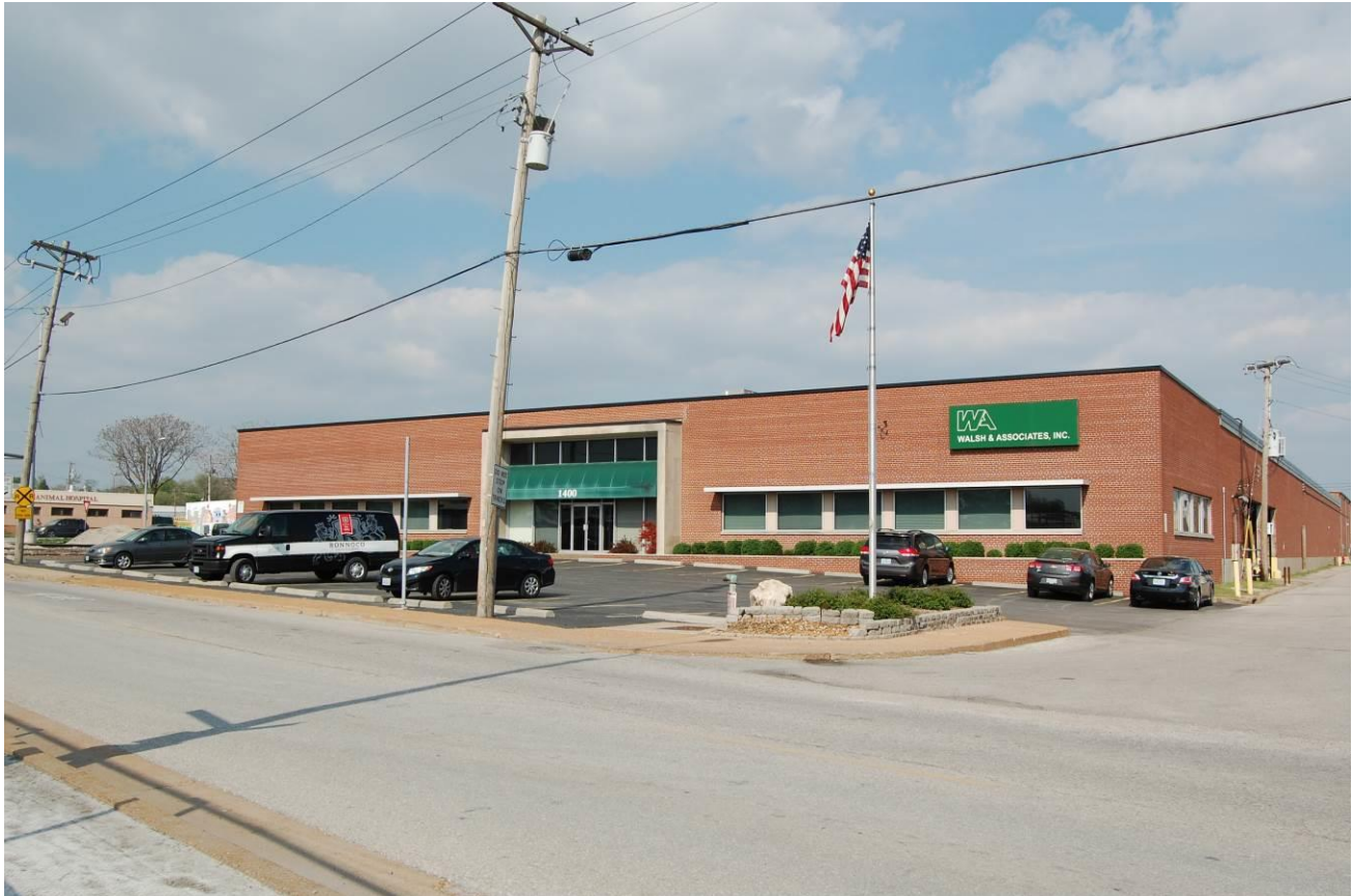
Figure 14. 1400 Macklind Avenue, view is northeast.
