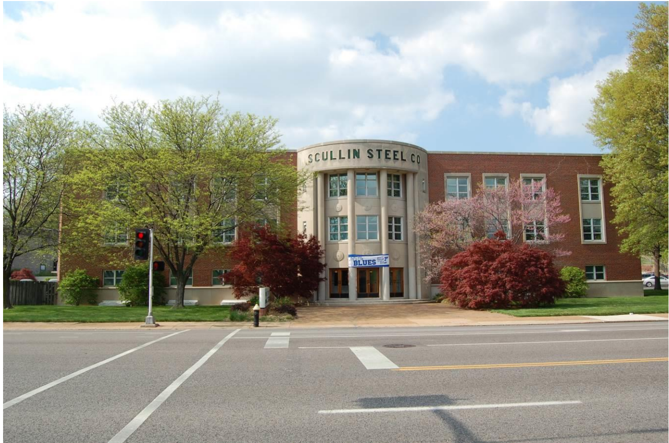
Figure 12. Scullin Steel Administration Building, 6691 Manchester Avenue, view is north.
