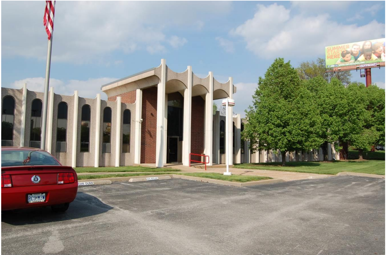
Figure 13. 1720 Sublette Avenue, view is northeast.
