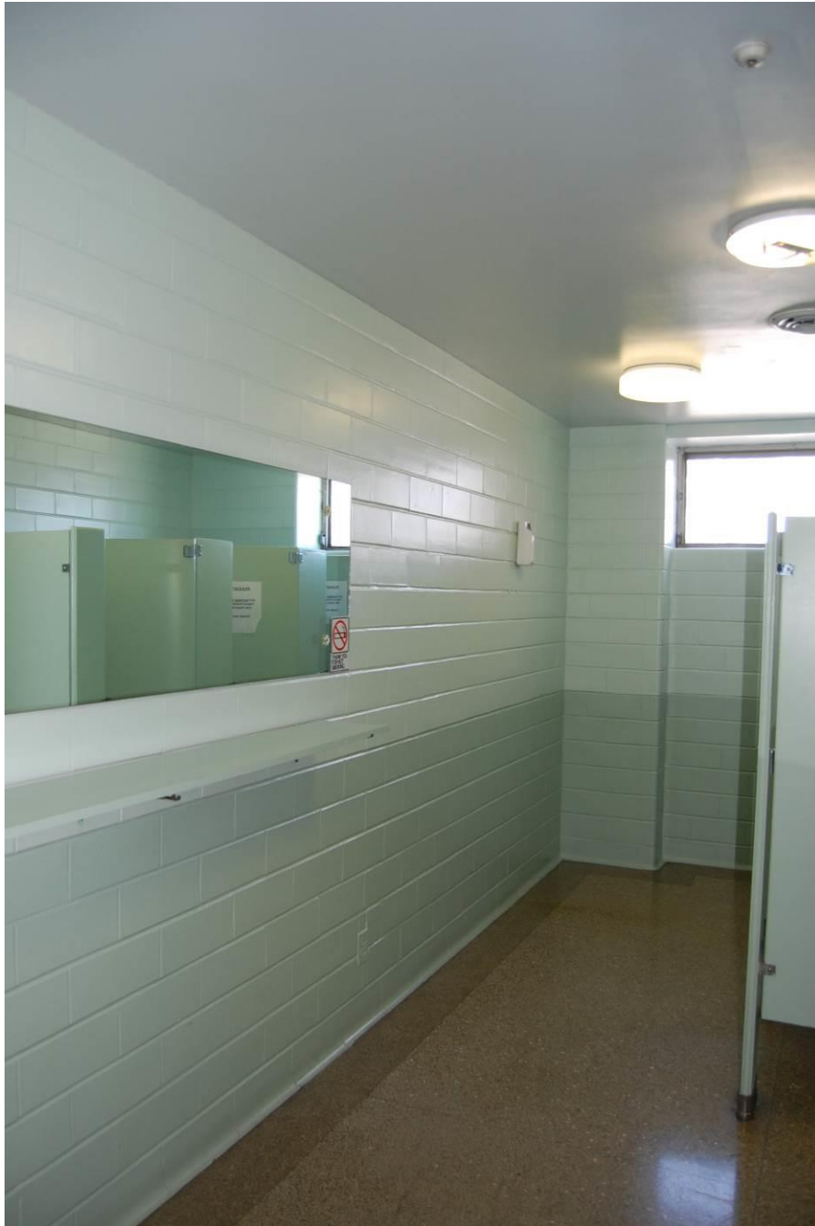
Figure 2. Original finishes in second-floor bathroom include terrazzo and concrete block.
