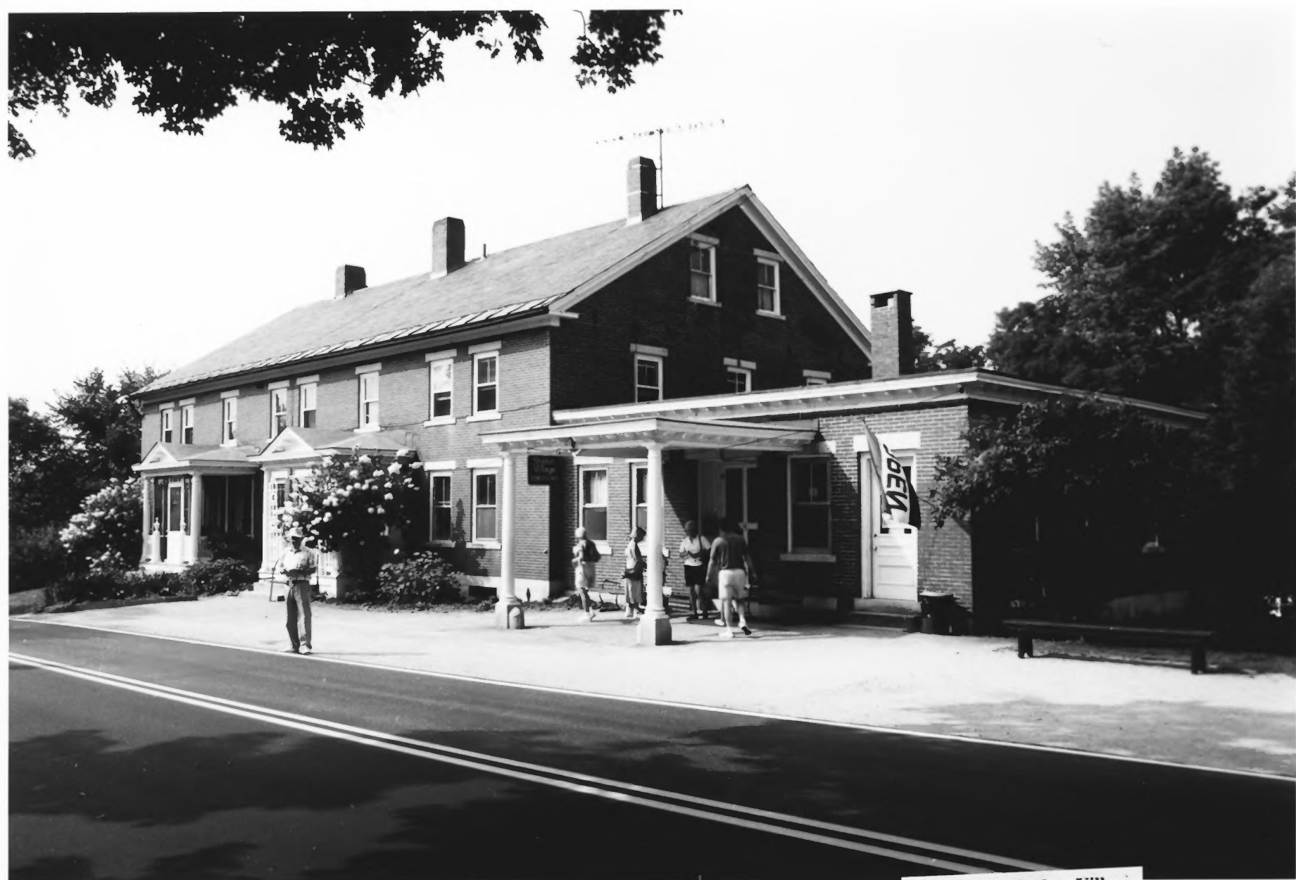
Canterbury Shaker Village Canterbury, N.H. Brick Trustees Office Photo: Lisa Mausolf, 1992
