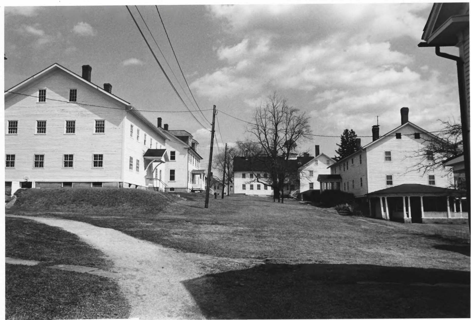
Canterbury Shaker Village Canterbury, N.H. Utility Buildings Photo: Lisa Mausolf, 1992
