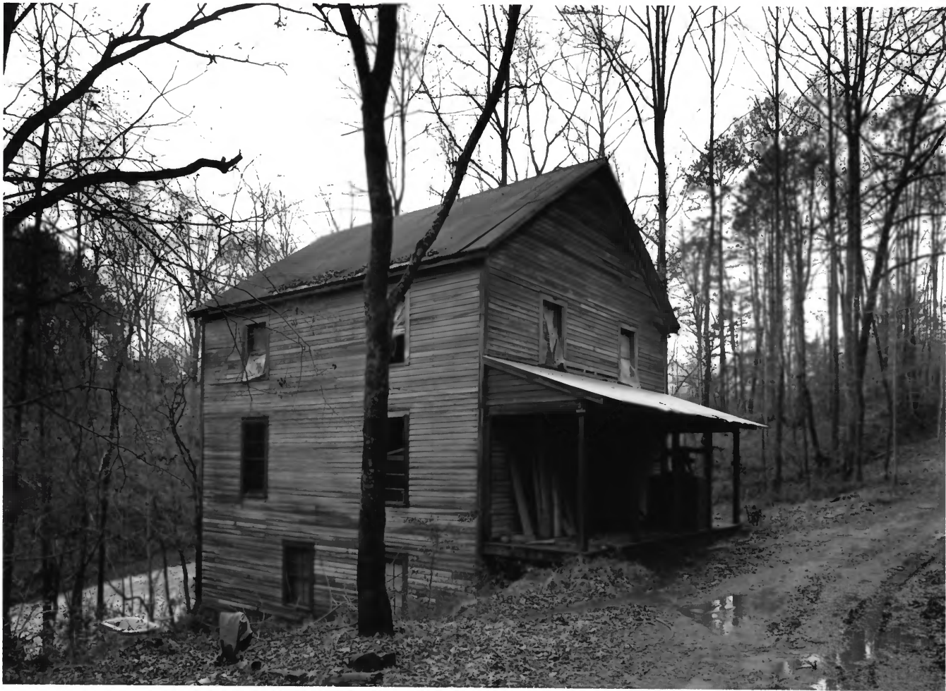
ELDER'S MILL COVERED BRIDGE AND ELDER MILL OCONEE COUNTY, GEORGIA 2 OF 14
