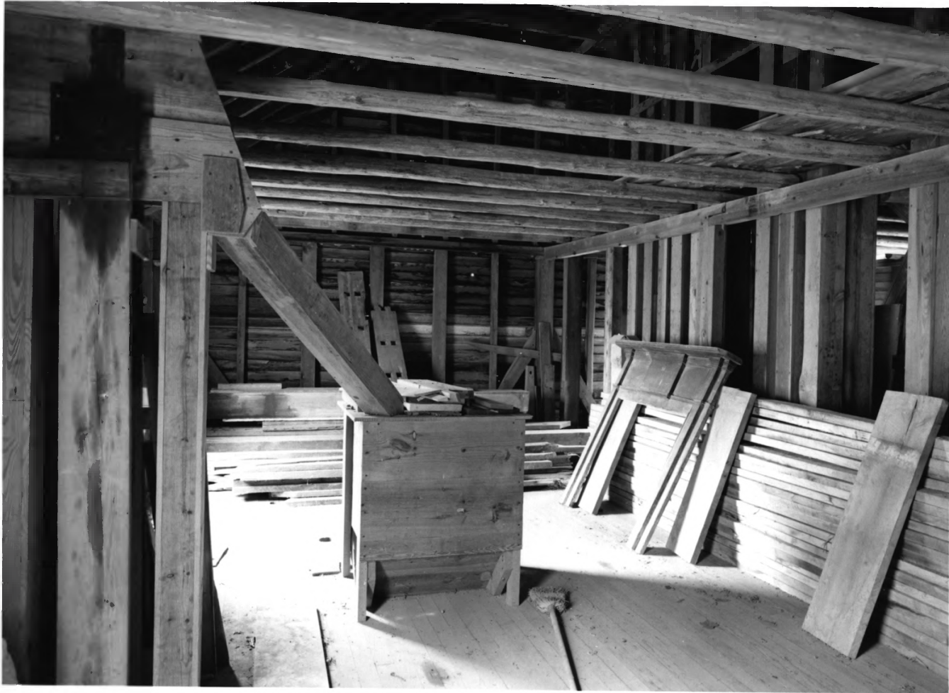
ELDER'S MILL COVERED BRIDGE AND ELDER MILL DCONEE COUNTY, GEORGIA 13 OF 14
