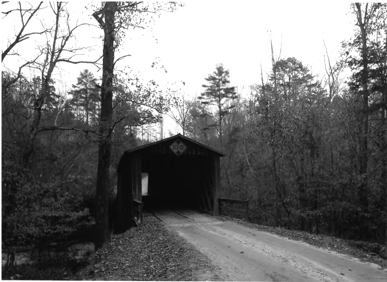
ELDER'S MILL COVERED BRIDGE AND ELDER MILL OCONEE COUNTY, GEORGIA 3 OF 14
