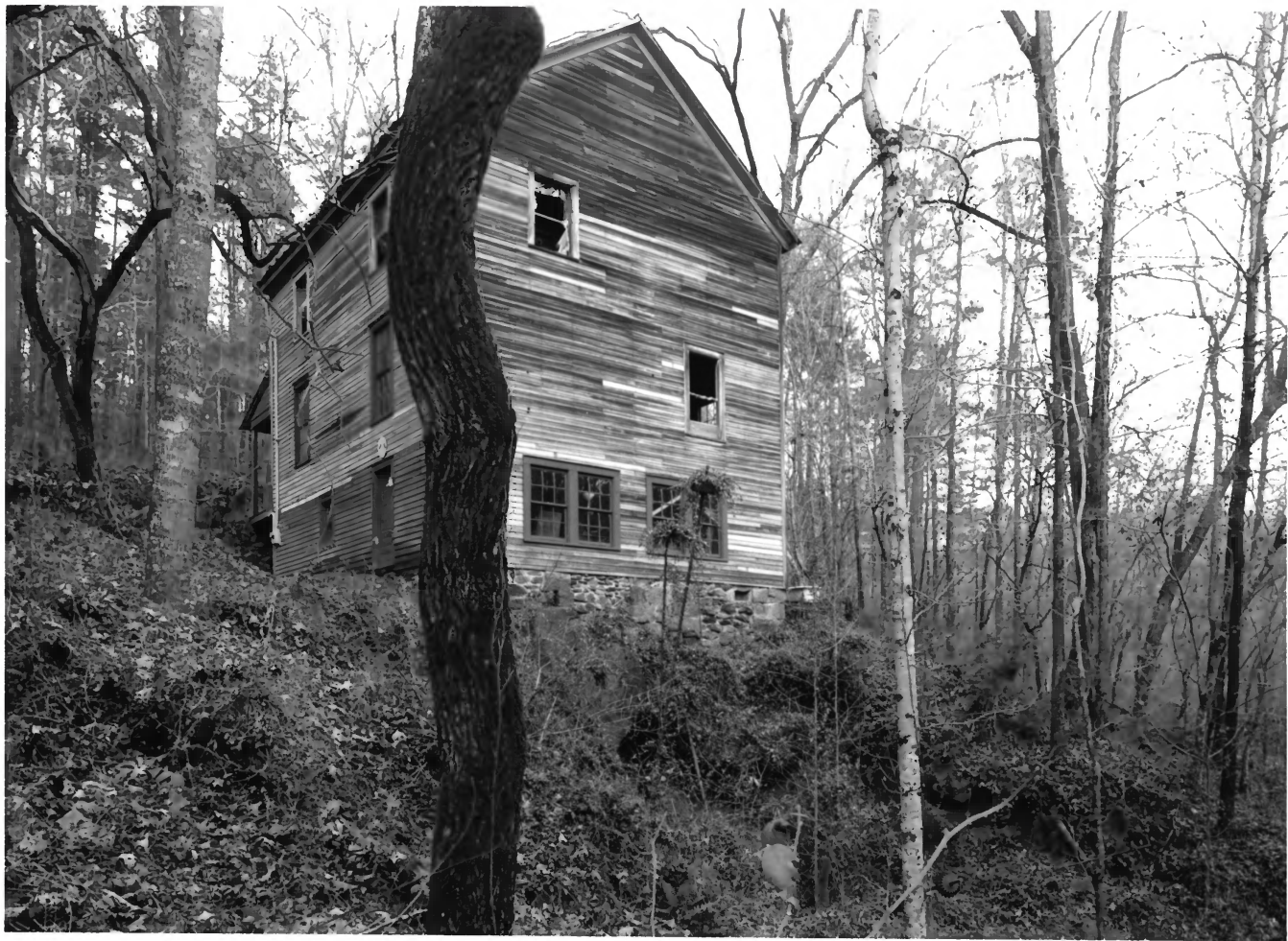
ELDER'S MILL COVERED BRIDGE AND ELDER MILL OCONEE COUNTY, GEORGIA 10 OF 14
