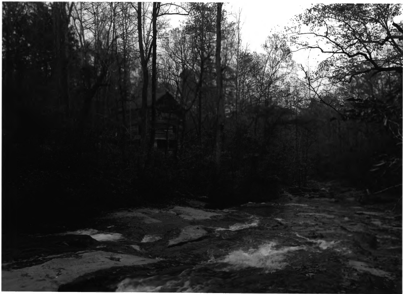
ELDER'S MILL COVERED BRIDGE AND ELDER MILL OCONEE COUNTY, GEORGIA 14 OF 14
