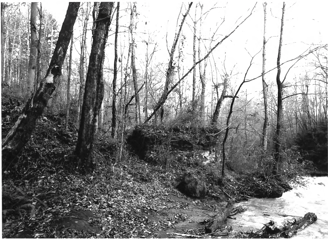
ELDER'S MILL COVERED BRIDGE AND ELDER MILL. OCONEE COUNTY, GEORGIA 8 OF 14
