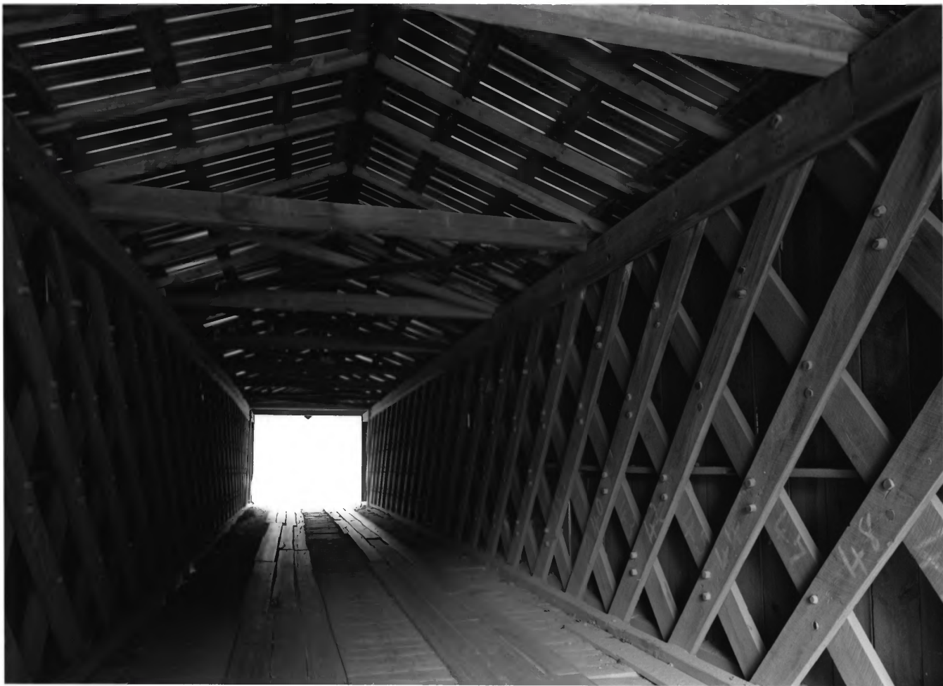
ELDER'S MILL COVERED BRIDGE AND ELDER MILL OCONEE COUNTY, GEORGIA 4 OF 14
