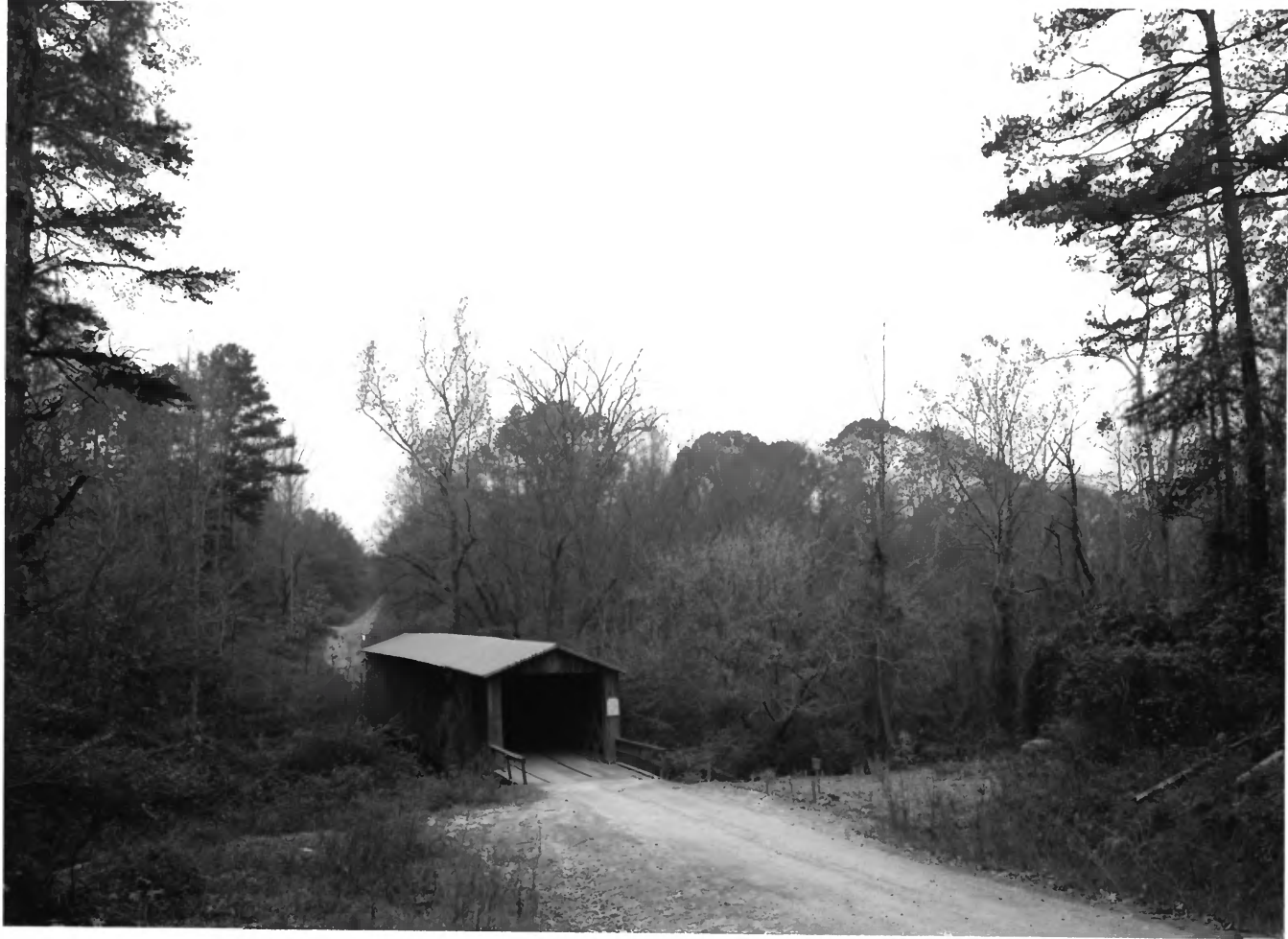
ELDER'S MILL COVERED BRIDGE AND ELDER MILL OCONEE COUNTY, GEORGIA 1 OF 14
