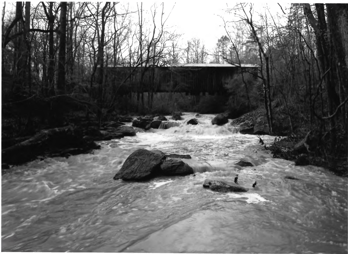
ELDER'S MILL COVERED BRIDGE AND ELDER MILL OCONEE COUNTY, GEORGIA 6 OF 14
