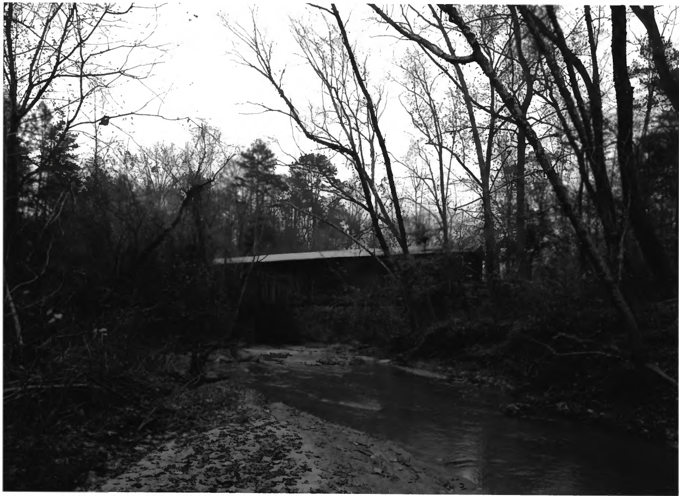
ELDER'S MILL COVERED BRIDGE AND ELDER MILL OCONEE COUNTY, GEORGIA 5 OF 14
