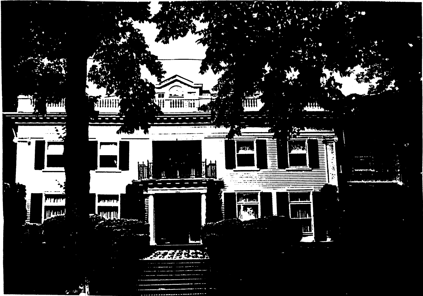
1961 S.W. Vista Avenue
