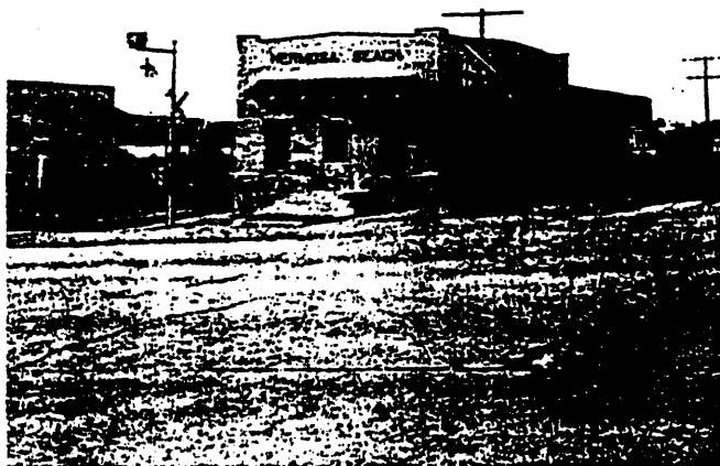
ABOVE: The Hermosa depot at 619 Pier Avenue taken in Nov. 1961. It opened in late 1927 as a ticket agency, train order office and Western Union Telegraph office. The 20x40 foot structure was built of concrete and contained two rooms. It was demolished on February 23-24, 1969.
