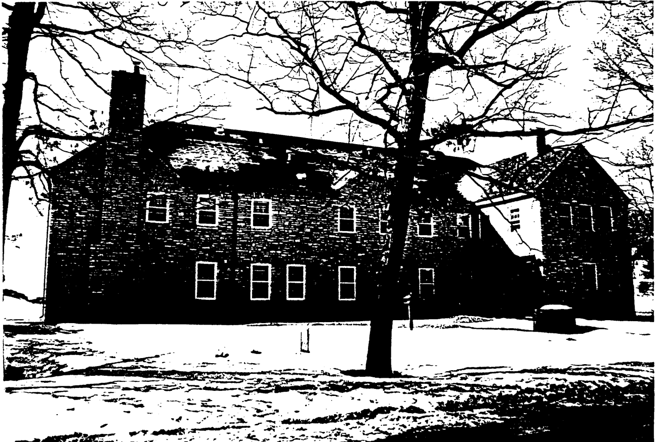
WISCONSIN INDUSTRIAL SCHOOL FOR GIRLS HISTORIC DISTRICT Fitchburg, WI Cottage #8 Looking West
