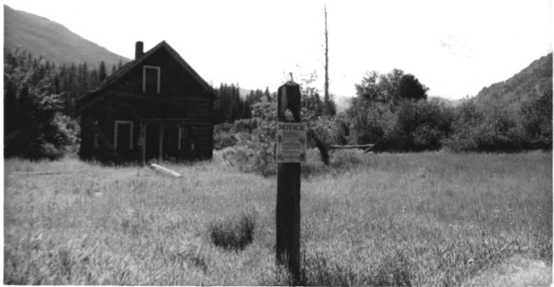
Photo #8 Bull River Guard Station Sanders County, MONTANA
