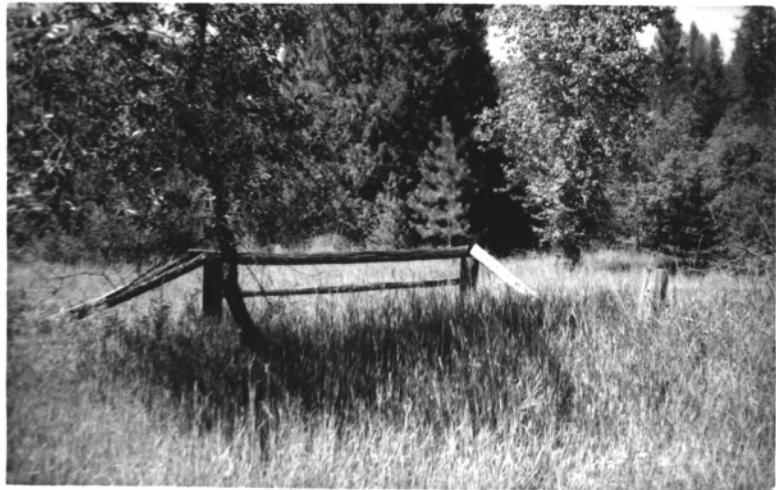
Photo # 7 Bull River Guard Station Sanders County, Montana
