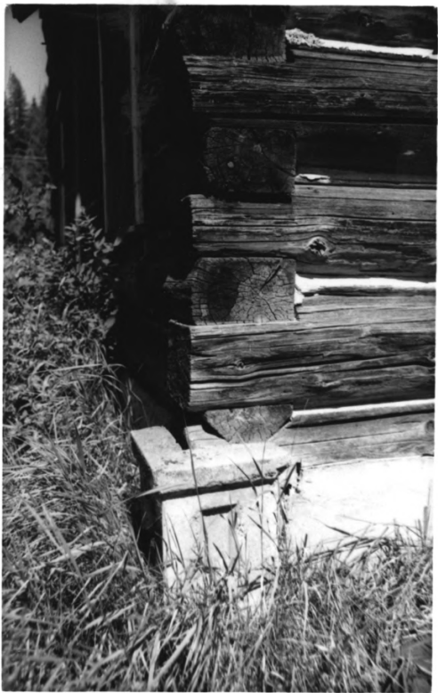
Photo #3 Bull River Guard Station Sanders County, Montana
