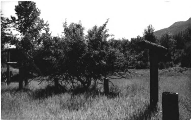
Photo #5 Bull River Guard Station SANDERS COUNTY, MONTANA
