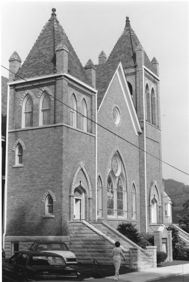
Methodist Episcopal Church South Prestonsburg MPS Floyd Co., KY
