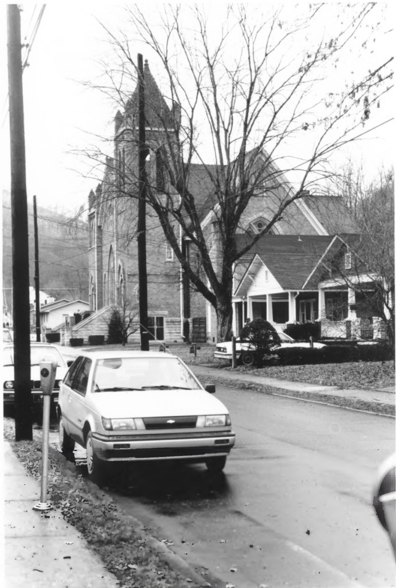
Methodist Episcopal Church South Prestonsburg MPS Floyd Co., KY 36
