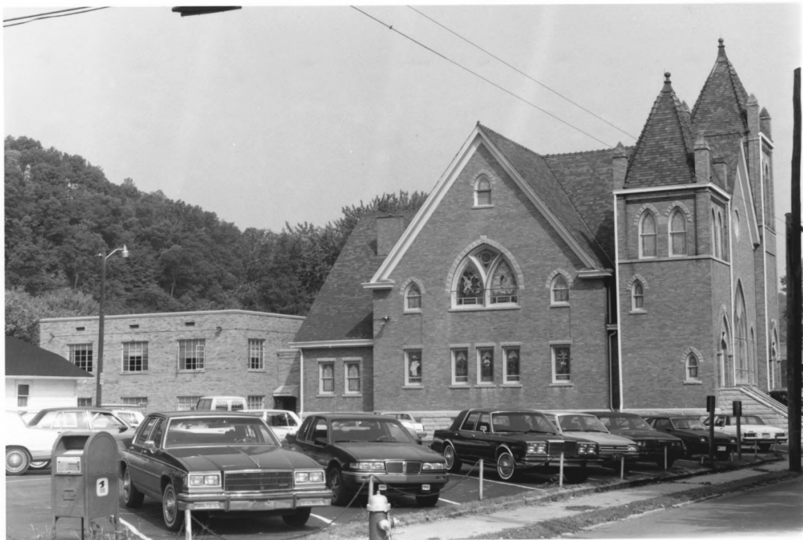
Methodist - Episcopal Church South Prestonsburg MRS Floyd Co., KY
