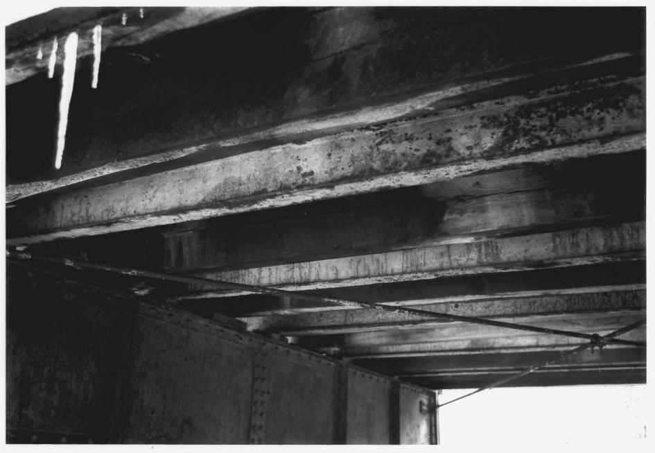
Photograph #5 Turn-of-River Bridge, Stamford, CT View of Deck Beam and Stringers Steven Bedford, January 1986 Negative on file at Connecticut Historical Commission
